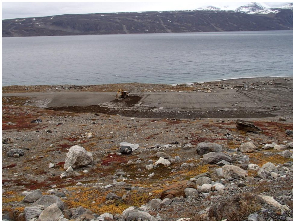
Photograph 30. Beach Area – Reshaping To Fill Drainage Ditch. September 5, 2013 (South West) ↑
