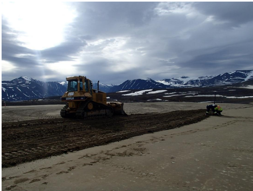
Photograph 8. LS Tier II DF – Placing Type 2 Granular Fill (Cell #1). July 6, 2013 (West)↑
