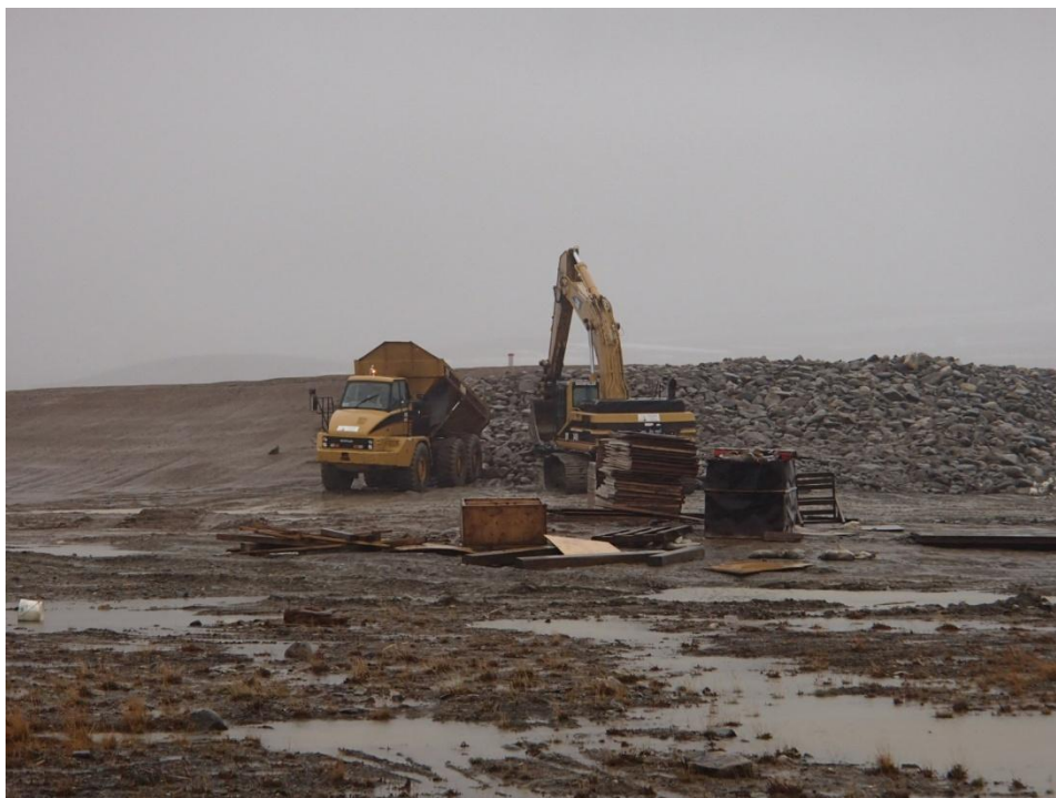
Photograph 11. LS Powerhouse Landfill – Type 1 Granular Fill Placement. July 12, 2013 (North East)↑
