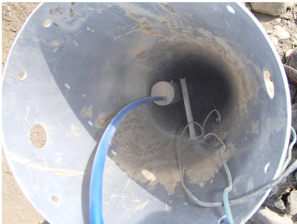
Photograph 23. LS Tier II DF – Typical Installation of Thermistor Cable. August 14, 2013 ↑
