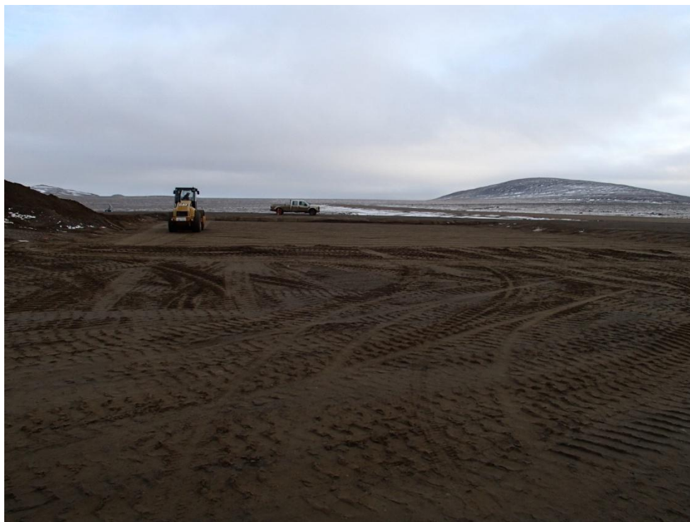
Photograph 31. LS NHWL – Construction of Type 2 Granular Cover Layer (Cell #2). September 13, 2013 (South)↑
