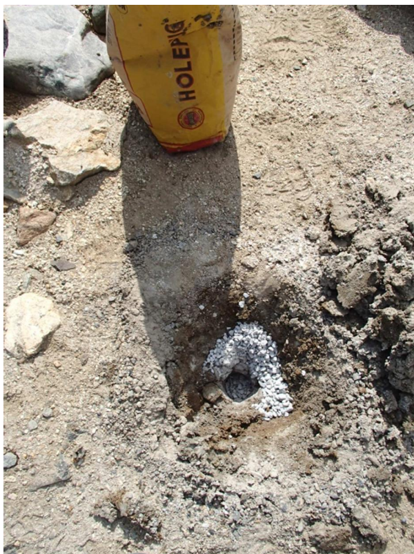
Photograph 21. US Tier II DF – Temporary Monitoring Well MW09-22A Decommissioning. July 29, 2013↑
