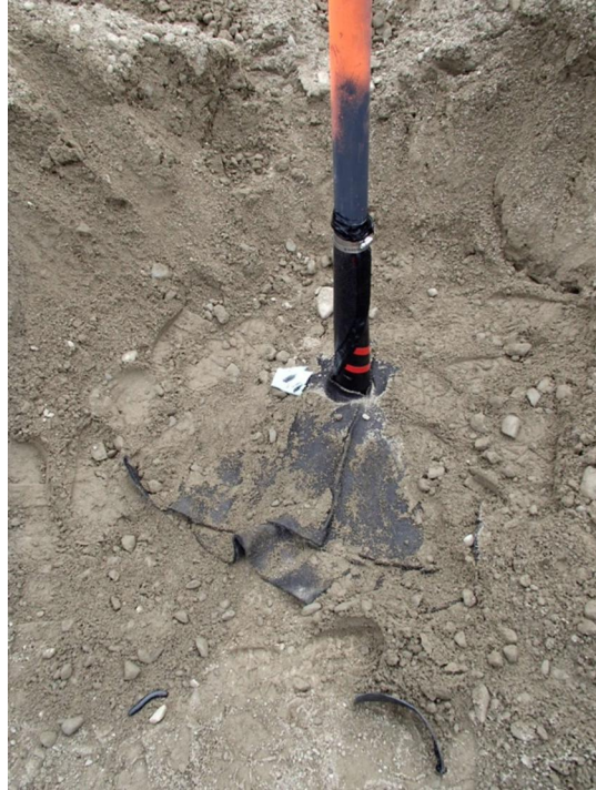
Photograph 19. LS Tier II DF – Installation of Neoprene Boot for VT-3. July 23, 2013 (N/A)↑
