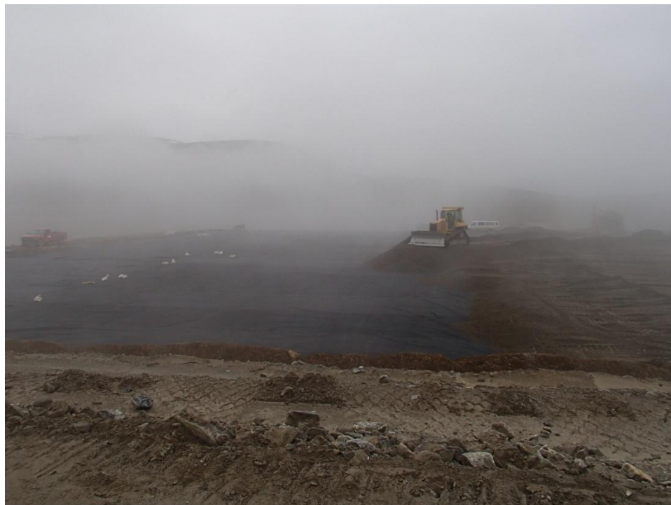
Photograph 20. LS Tier II DF (Cell #2) – Type 5 Granular Fill Placement. July 24, 2013 (North East) ↑
