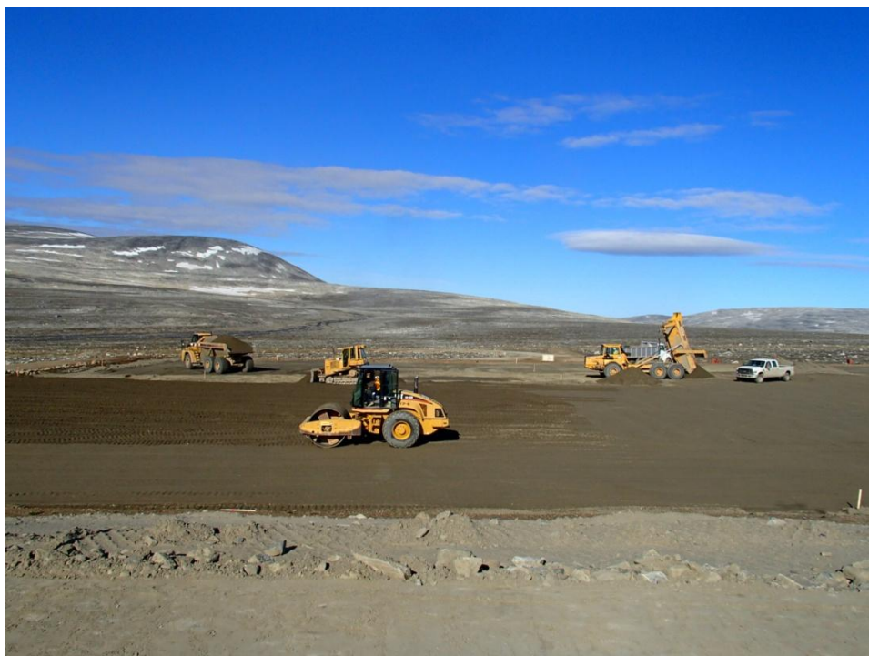
Photograph 12. LS Tier II DF – Placing Type 5 Granular Fill (Cell #2). July 15, 2013 (North East) ↑
