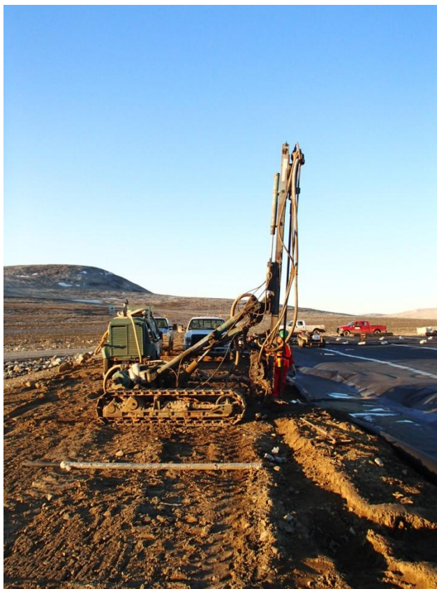
Photograph 16. LS Tier II DF – Drilling Thermistor VT-1. July 22, 2013 (North East)↑
