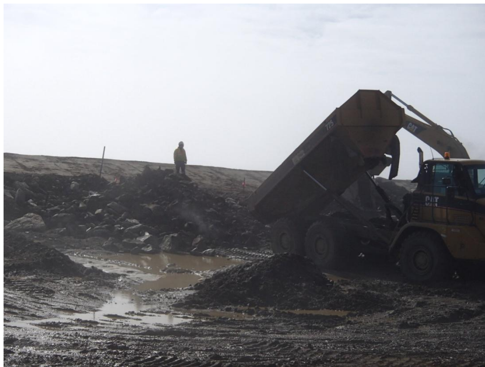
Photograph 15. US Tier II DF – Type 1 Granular Fill Placement. July 21, 2013 (North)↑
