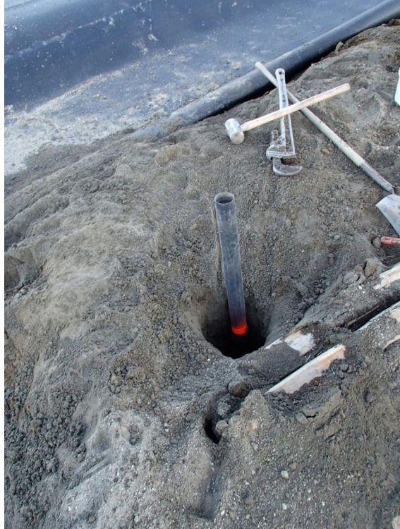
Photograph 17. LS Tier II DF – Installation of PVC Casing for VT-1. July 22, 2013 (N/A)↑
