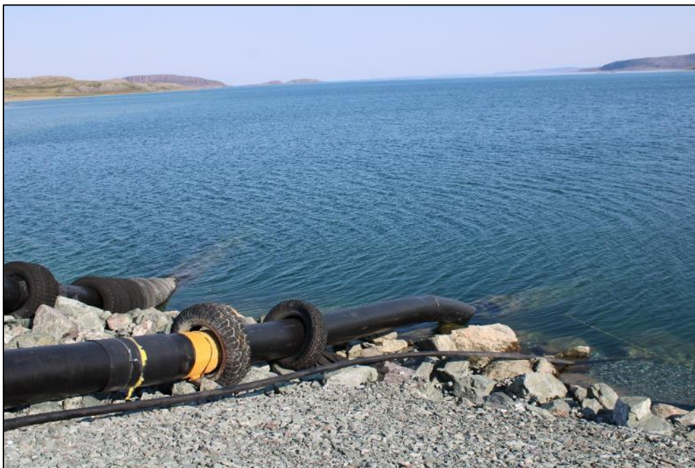
Photo 21: Saline Discharge and Water Recirculation lines.
