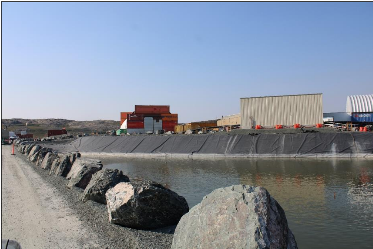
Photo 5: Sedimentation Pond at Doris North which collects Runoff Water.
