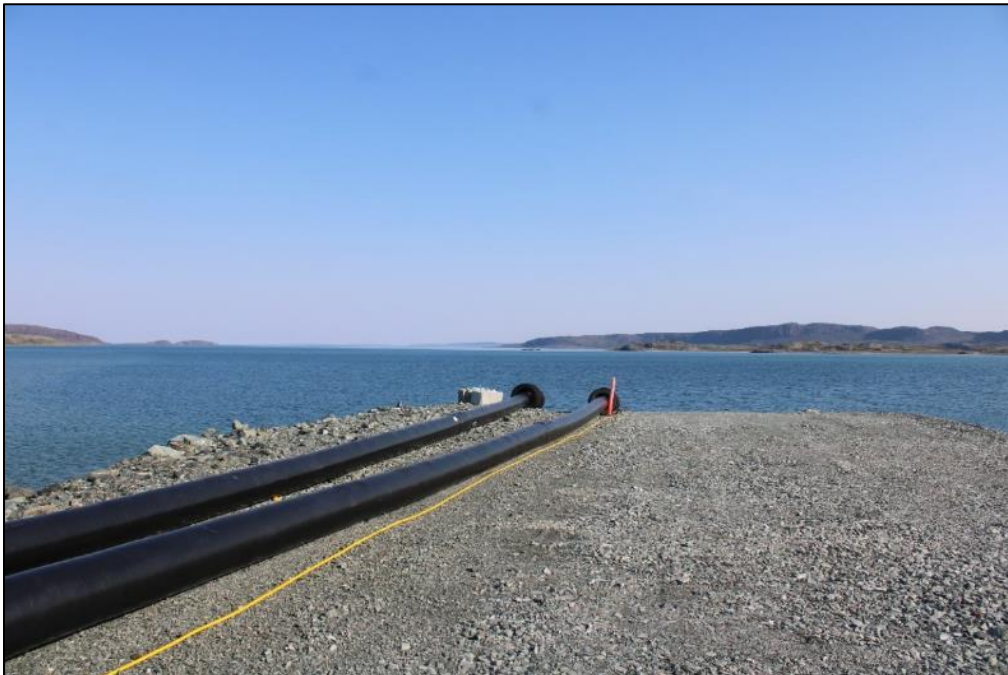
Photo 20: Saline Discharge and Water Recirculation Lines along the Roberts Bay Jetty.
