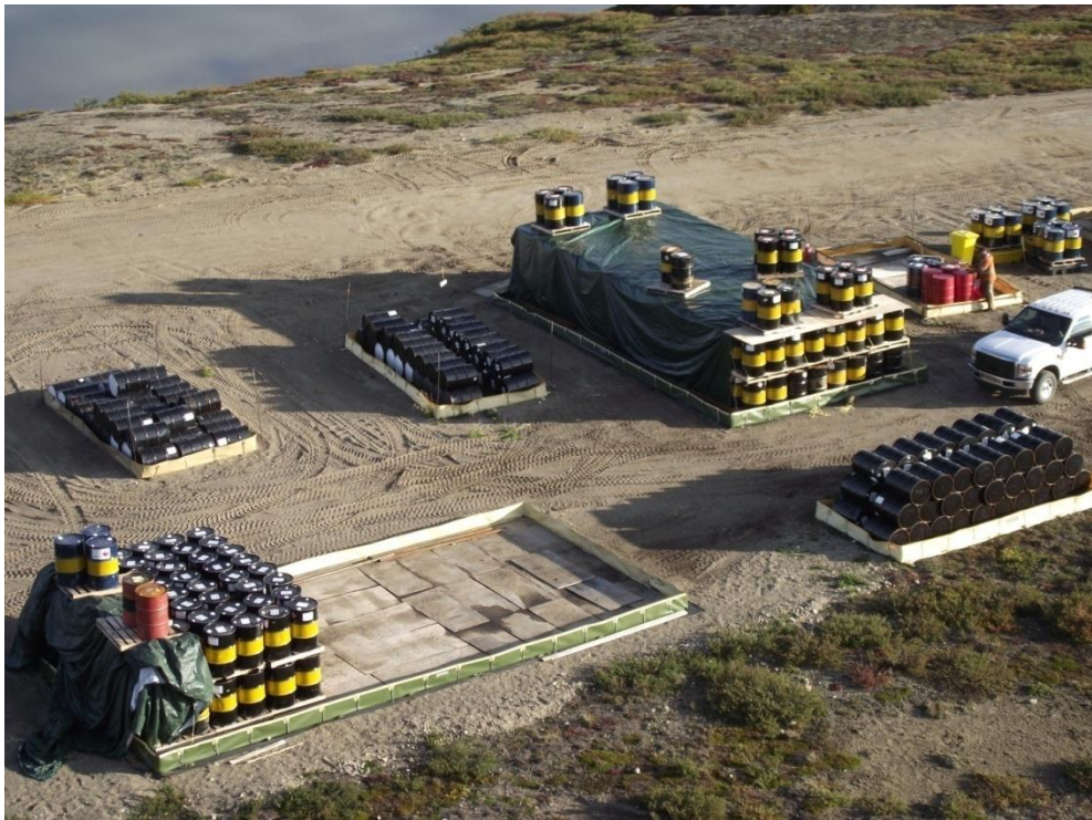
Drum storage onsite with secondary containment berms – August 2011
