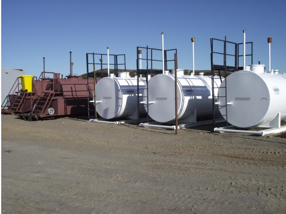
Fuel farm 11,000L double walled portable tanks with spill kit – August 2011
