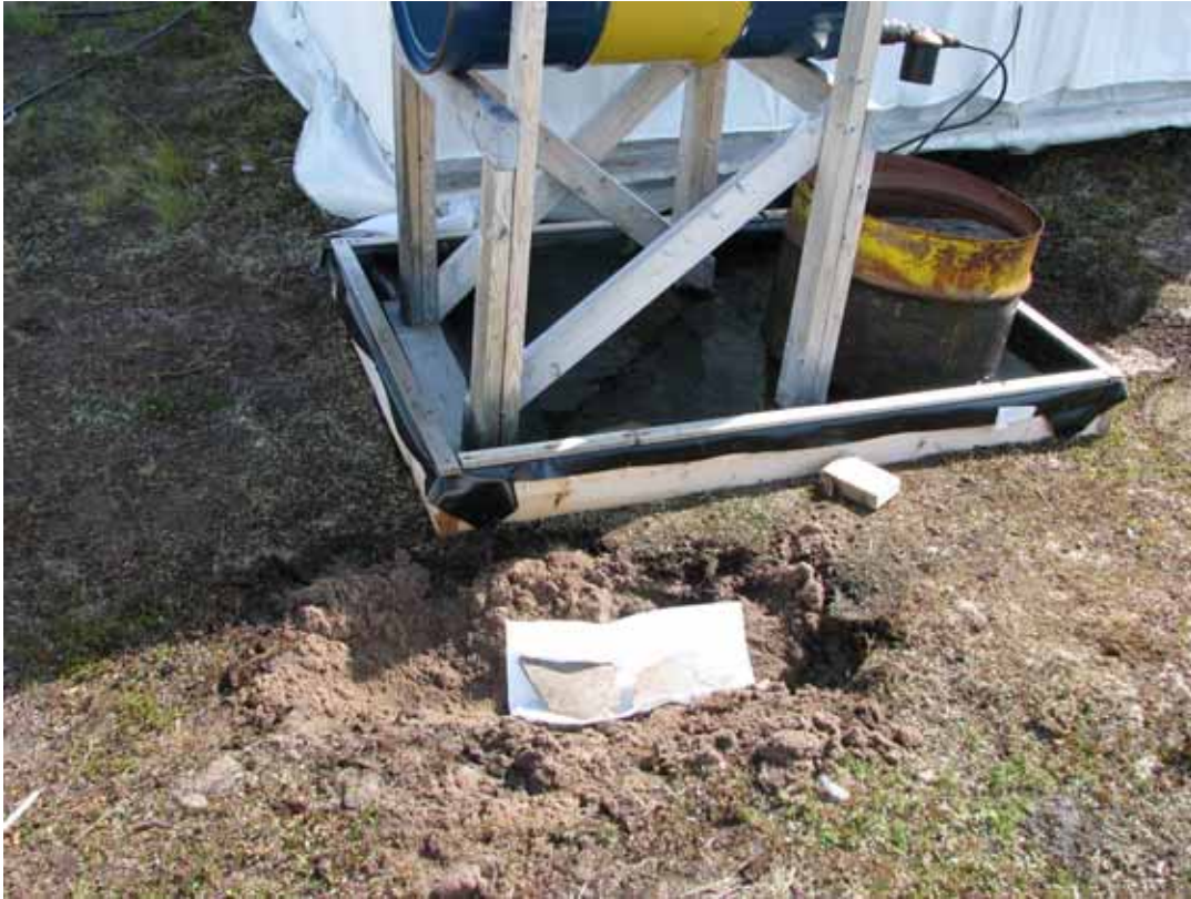
Figure 6: Excavation of fuel-contaminated soil with absorbent matting.
