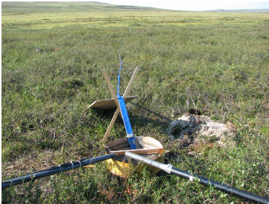
Figure 21: Grey water sump pit. The blue collapsible blue line pumps screened grey water 100 feet further inland from Thom Lake.
