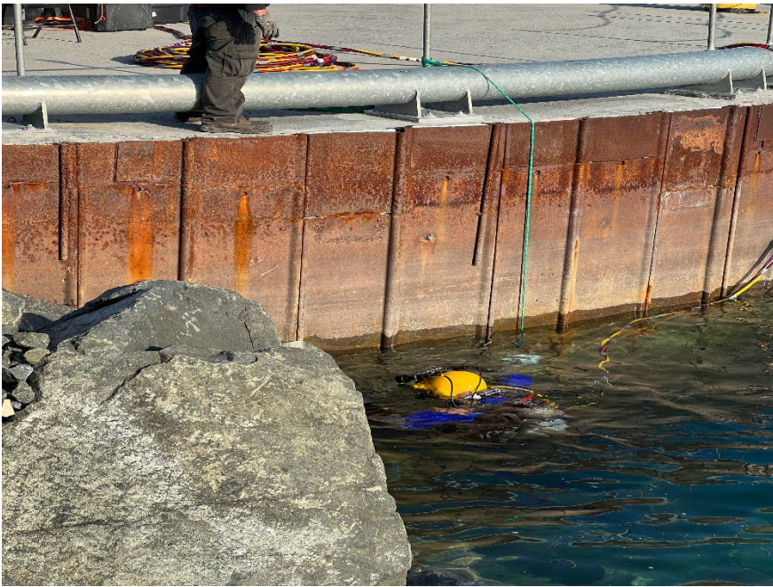
Figure 4. Wharf Dive Inspection
