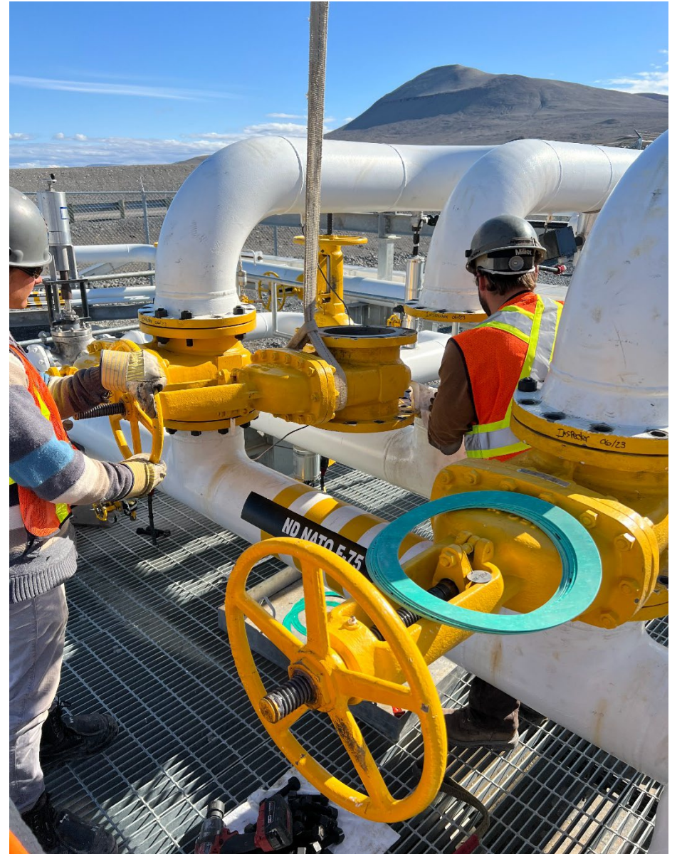
Figure 3. Valves Replacement
