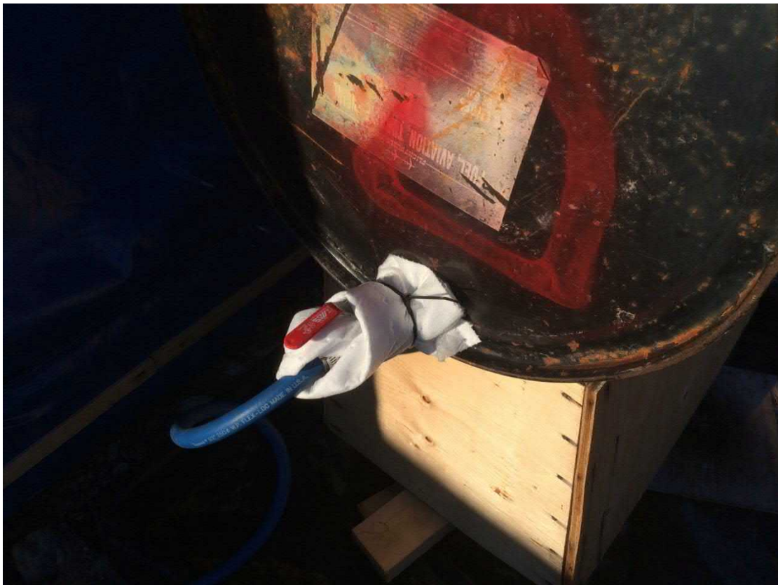
Photo 4: Absorbent Matting Wrapped Around Tent Drum Fuel Line Fitting
