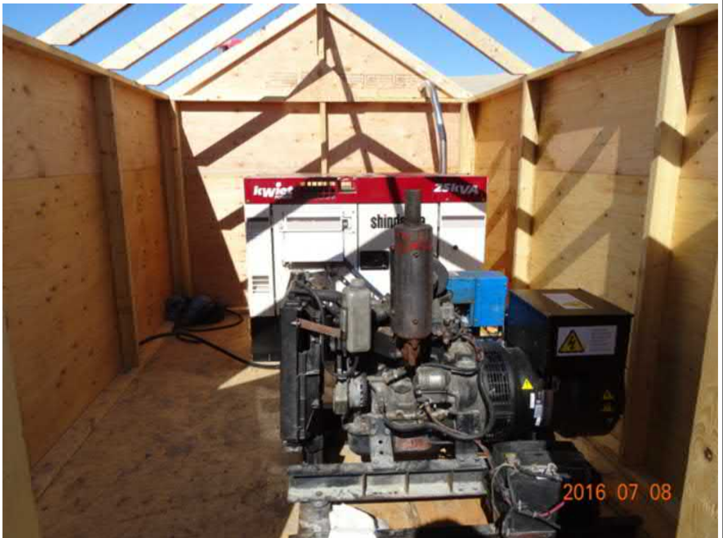
Figure 12 Gen shack with back up
