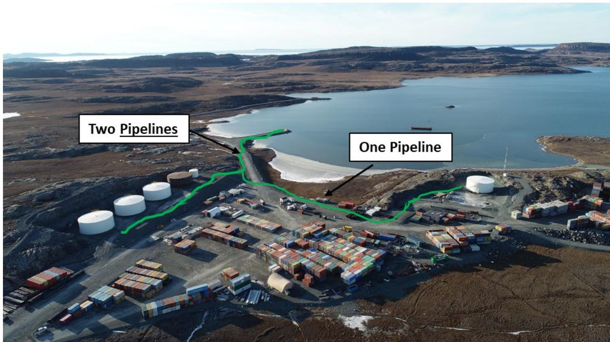
Figure 3 Fuel Transfer Pipeline Routing Looking West
