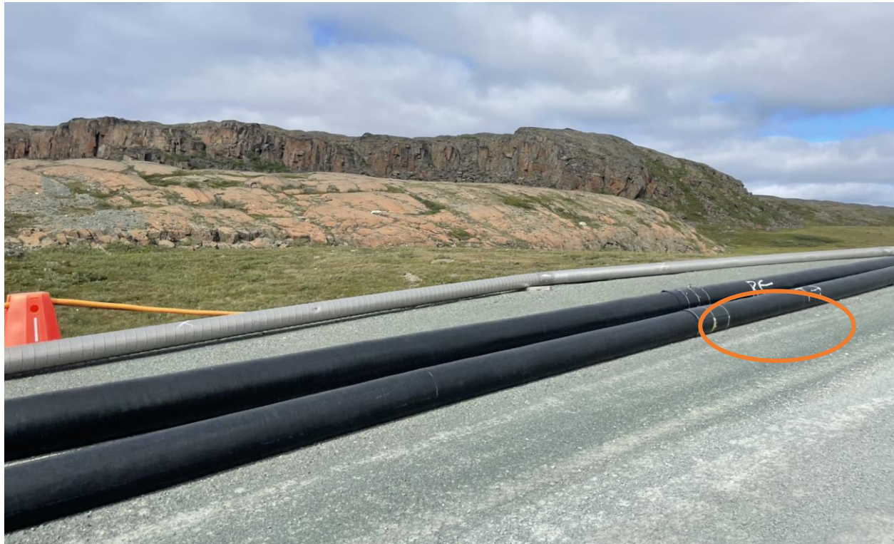
Photo 29: Waterlines labelled 'T' and 'R' run along the TIA Access Road, Transferring Treated Effluent to Roberts Bay and Effluent to the TIA Reclaim Pond
