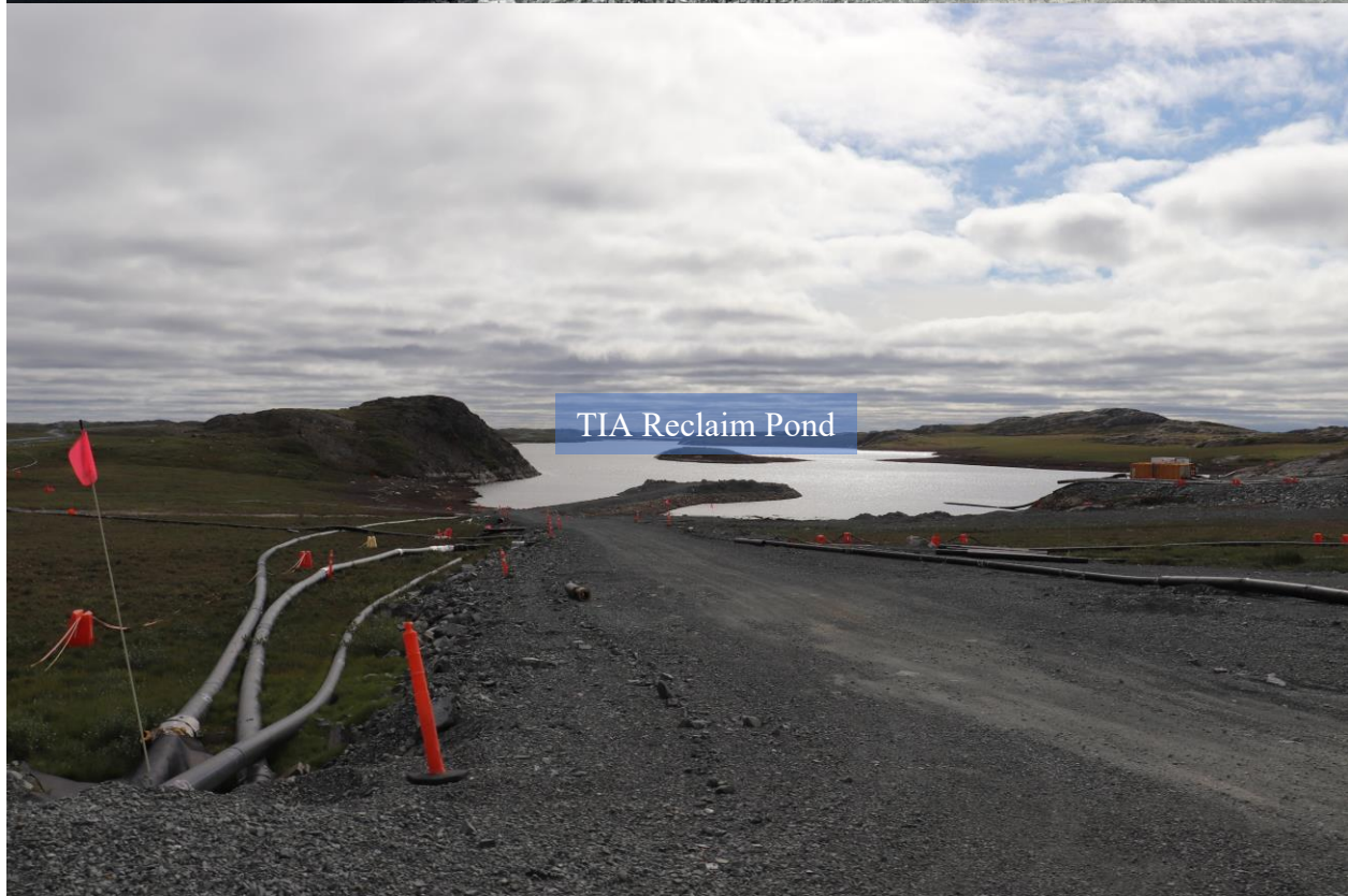
Photo 36: TIA Lake, Effluent Water Treatment Plant (EWTP), and Reclaim Pumphouse
