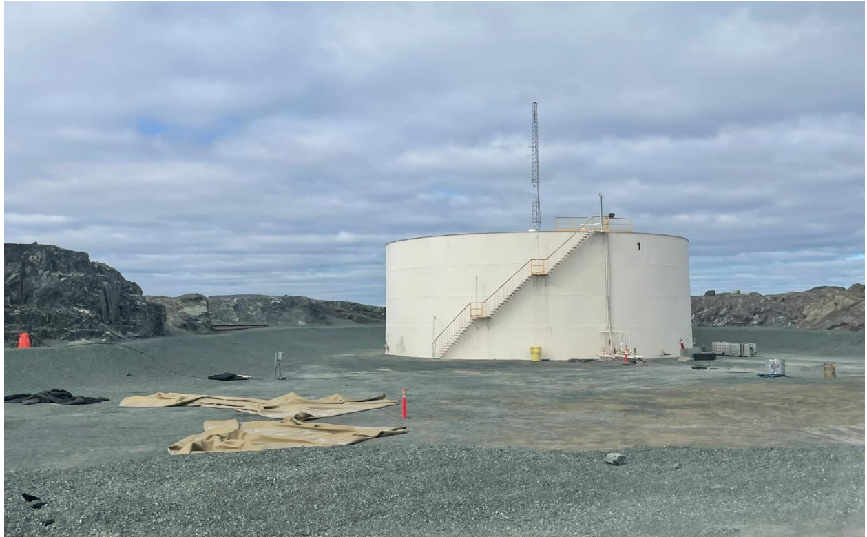
Photo 3: Tankfarm within Secondary Containment
