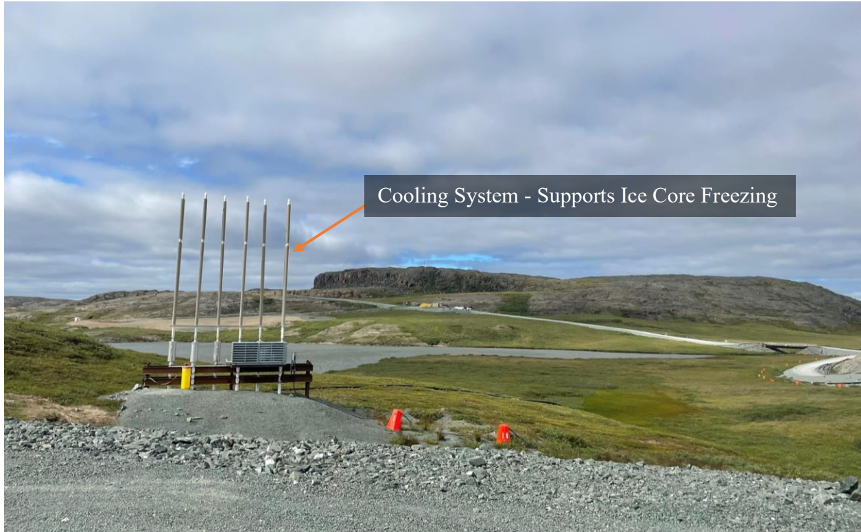
Photo 34: Thermosyphon Cooling System at the North Dam
