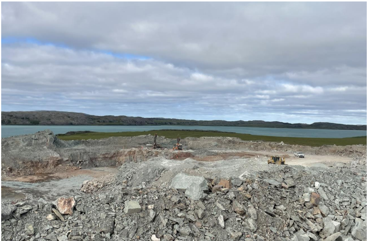
Photo 59: Construction of Saline Water Storage Pond at Quarry D
