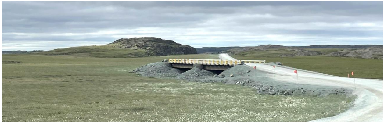
Photo 39: Bridge and Flags on Doris-Windy All-Weather Road
