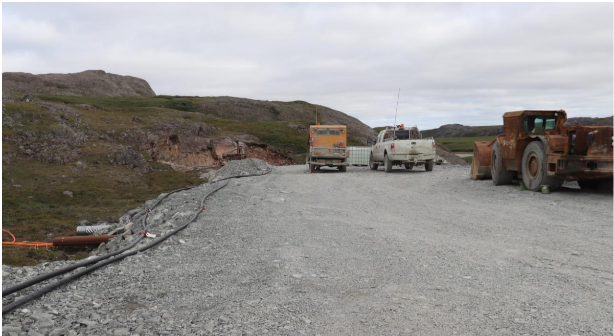
Photo 49: Construction of Ventilation Raise Collar at Naartok East
