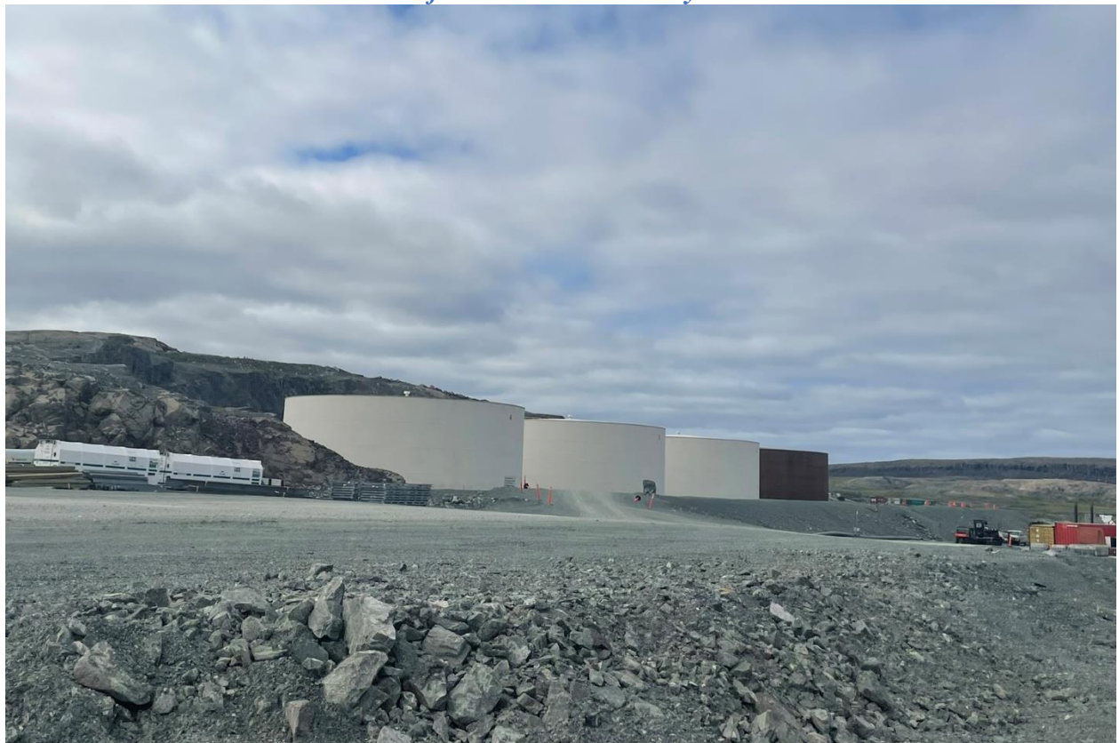
Photo 4: Tankfarm – Southwest View from Primary Road
