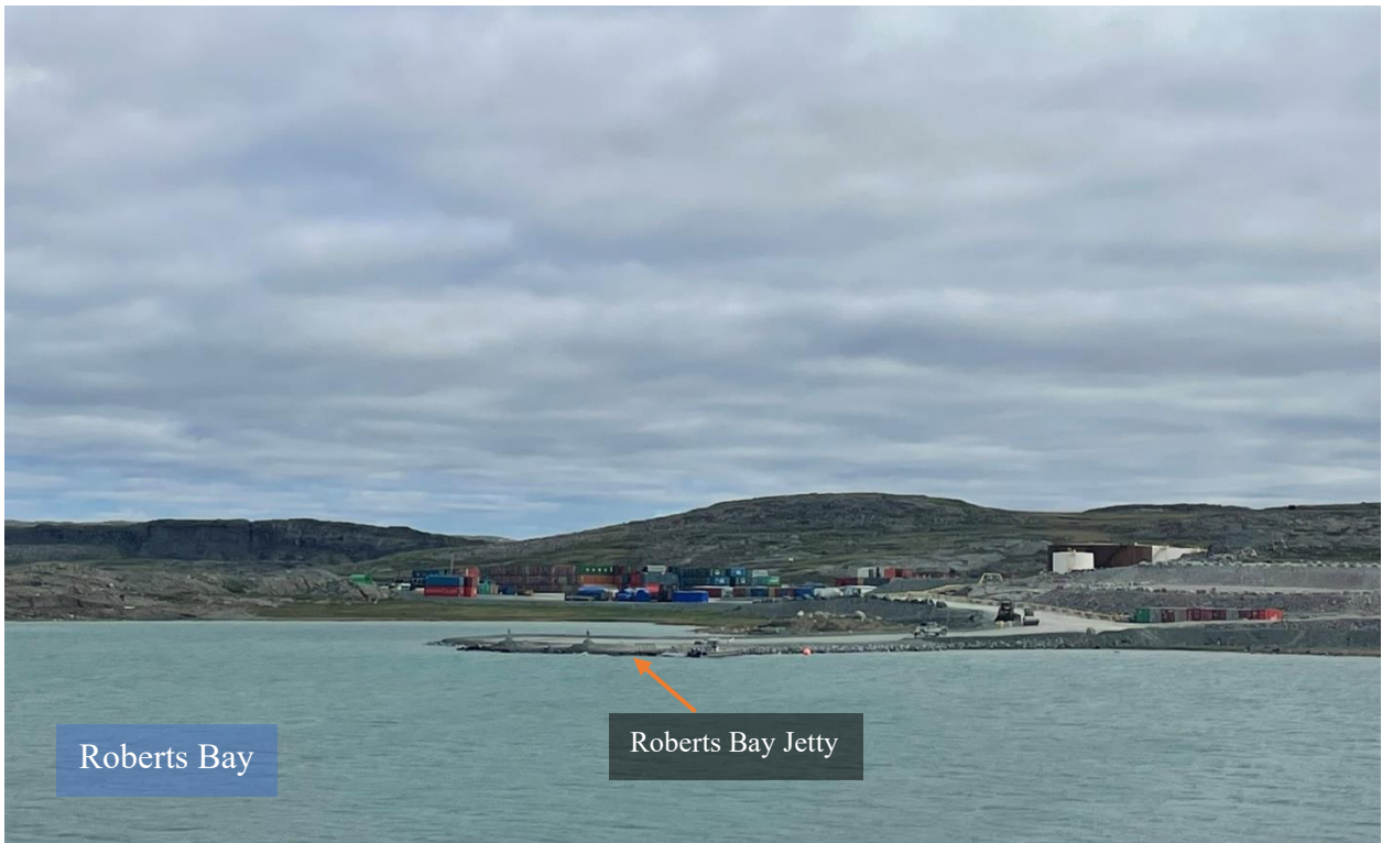
Photo 2: Roberts Bay Laydown Area, west view from the Roberts Bay Access Road
