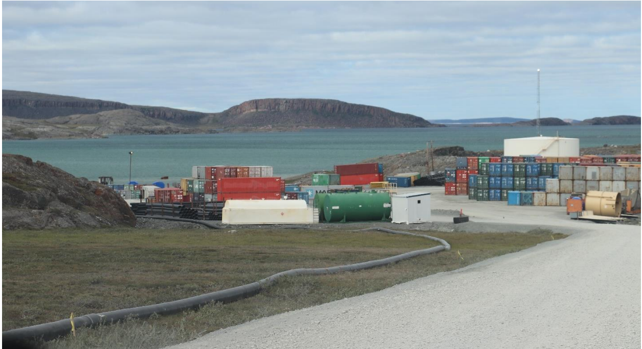
Photo 1: Roberts Bay Facilities and Laydown Area, Northwest View from the Primary Road
