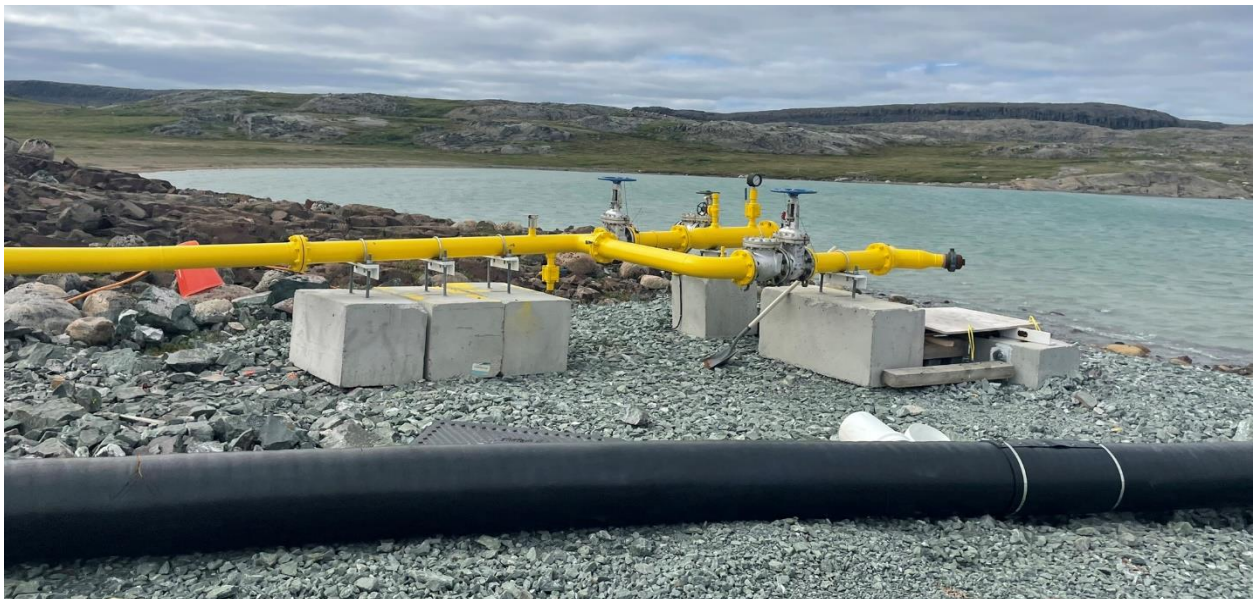
Photo 8: Fuel Line Anchor
