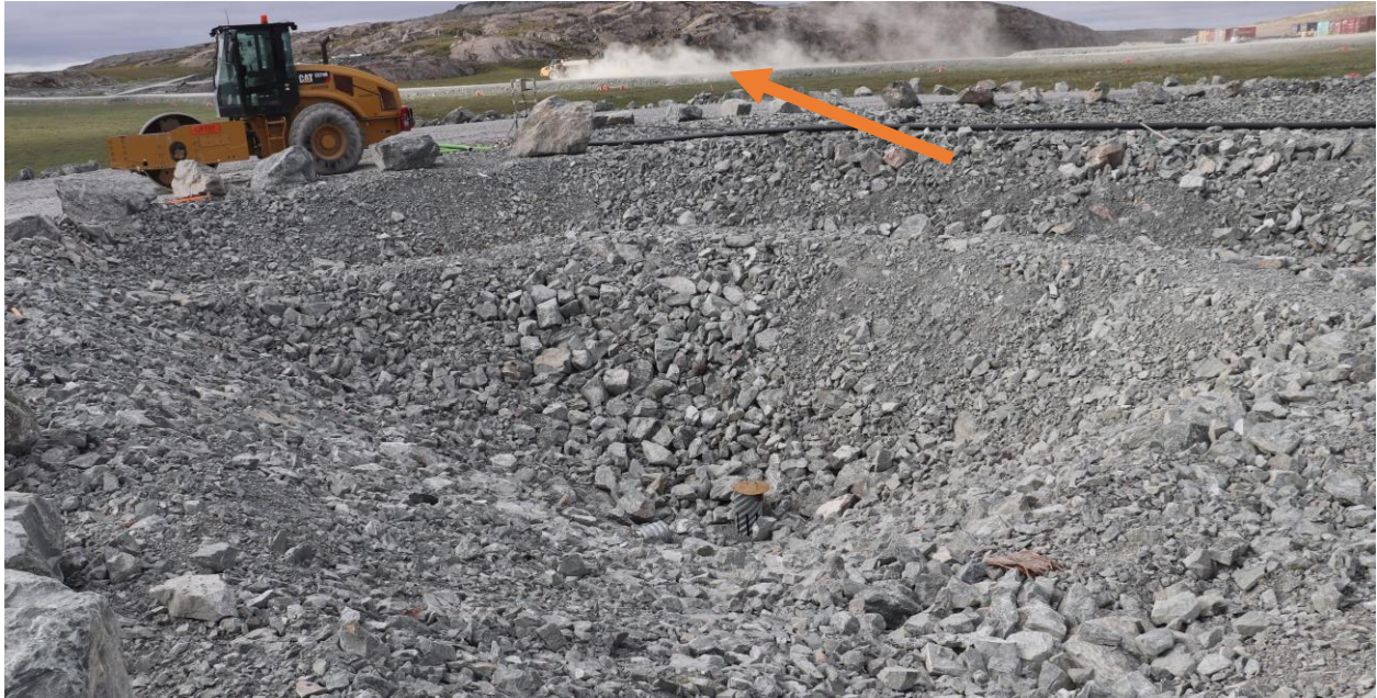
Photo 53: CPRT Sump with vehicle transit on Madrid All-Weather Road in background
