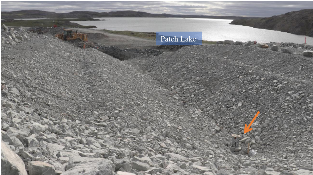
Photo 52: Crown Pillar Recovery Trench (CPRT) and Sump
