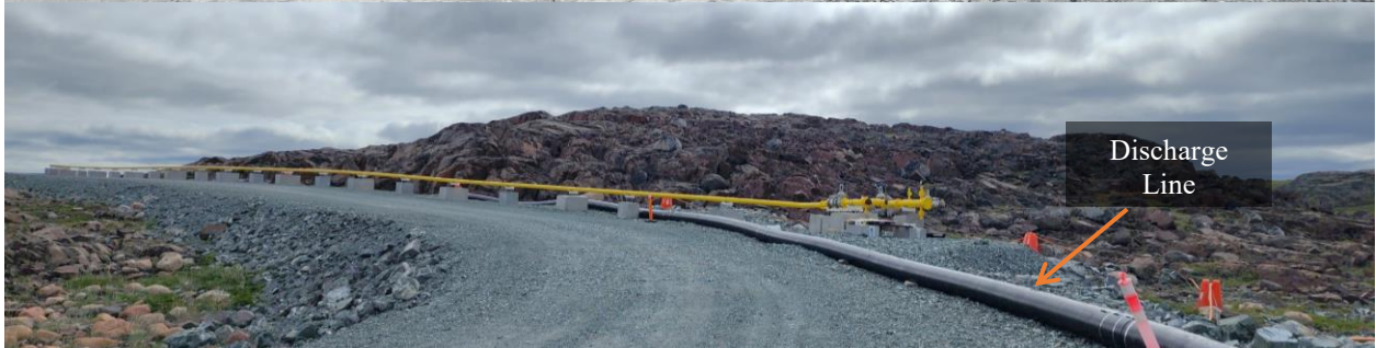
Photo 6: Fuel Line at Roberts Bay
