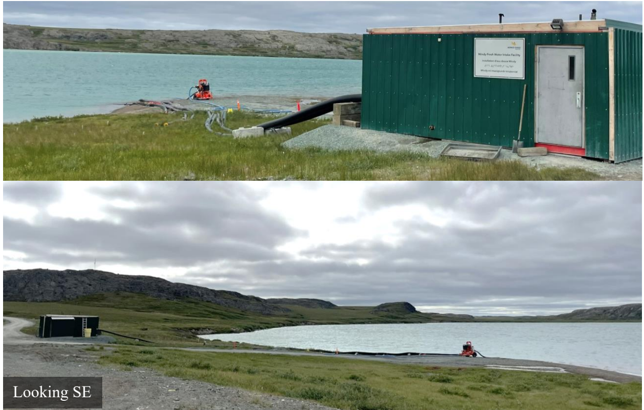
Photo 44: Windy Lake and Windy Fresh Water Intake Facility
