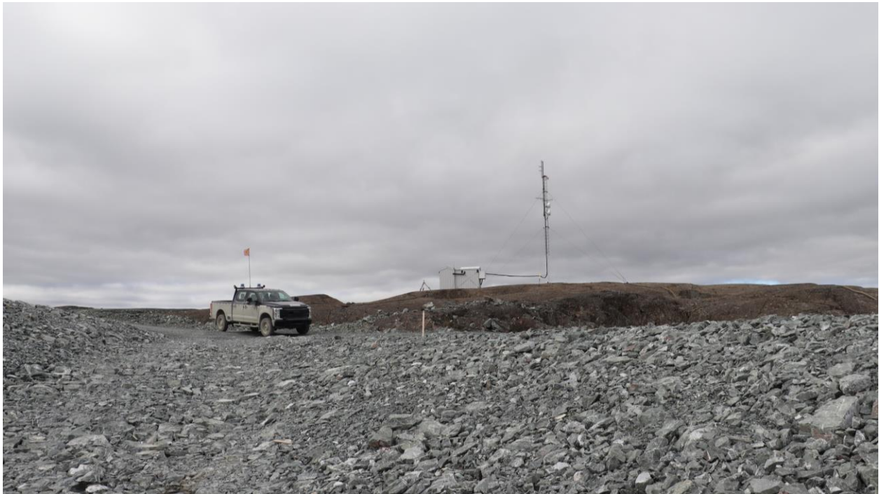
Photo 58: Weather Station at Madrid North
