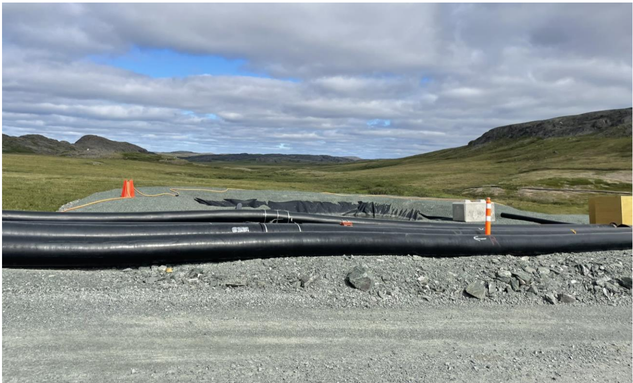
Photo 31: Catch Basin 1 - One of Two Catch Basins Located on Opposite Sides of Doris Creek Bridge for Emergency Discharge
