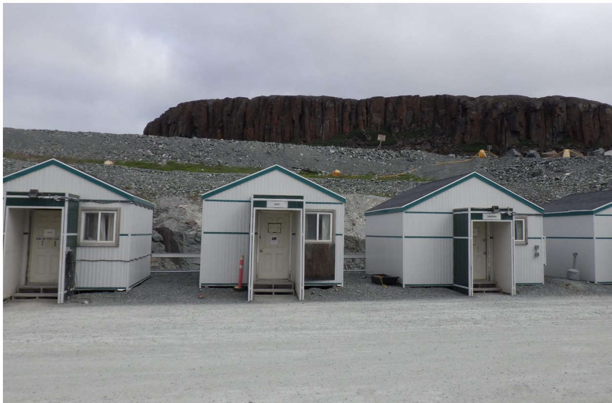
Photo 26: Emergency Response Team (ERT) and Training Buildings
