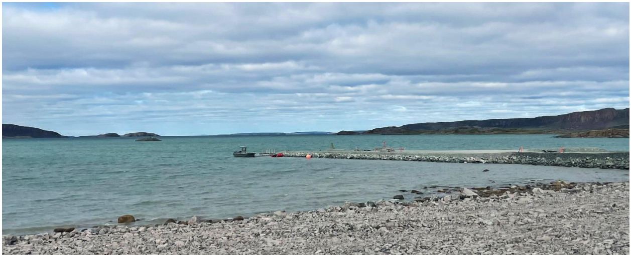
Photo 9: Treated Effluent Discharge Pipeline and Pumphouse – Weight Addition and Diffuser Reattachment Completed in 2024
