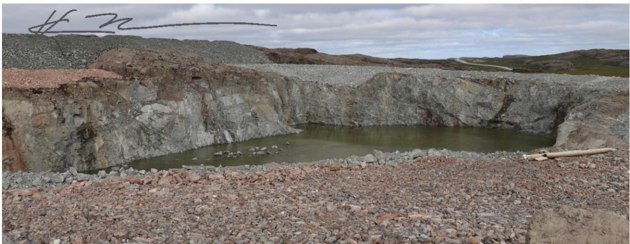
Photo 55: CWP2 Sump - used for collecting leakage from CWP2
