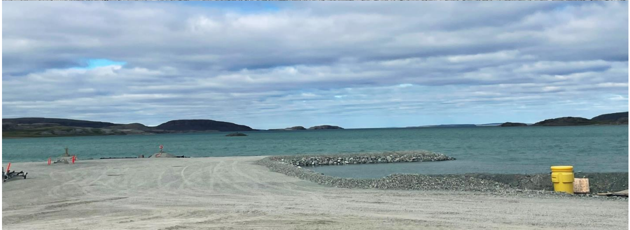
Photo 10: Roberts Bay Jetty
