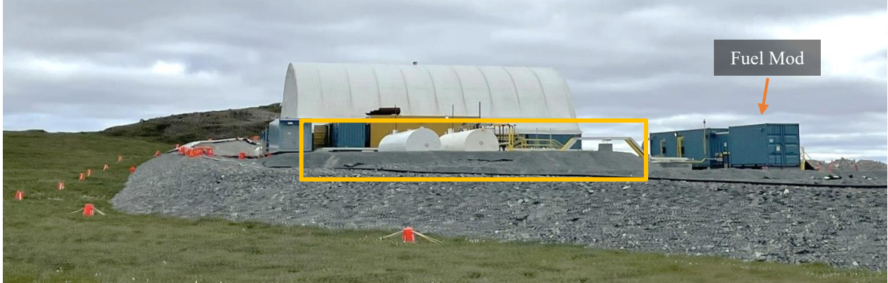
Photo 51: Infrastructure Pad adjacent to Naartok CPRT with fuel tanks in containment
