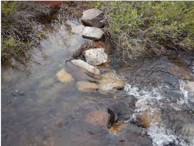
Photo E-5: View of a boulder and a cobble flow mitigation structure located 217 m upstream from the Goose Lake confluence on Rascal Creek – West, 5 July 2021.
