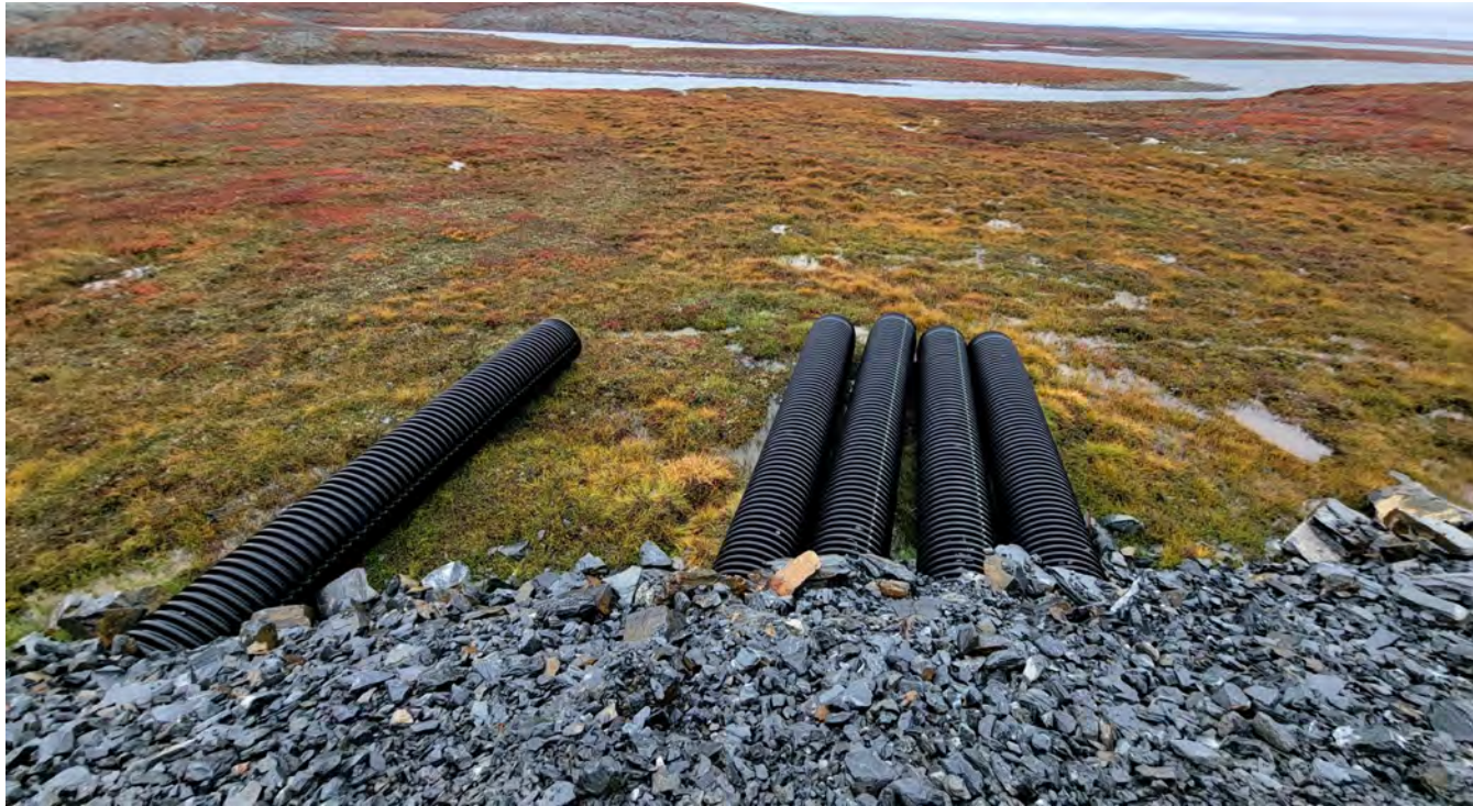
G-89. – Culvert: Outlet. Note some ponding water at the toe of the road
