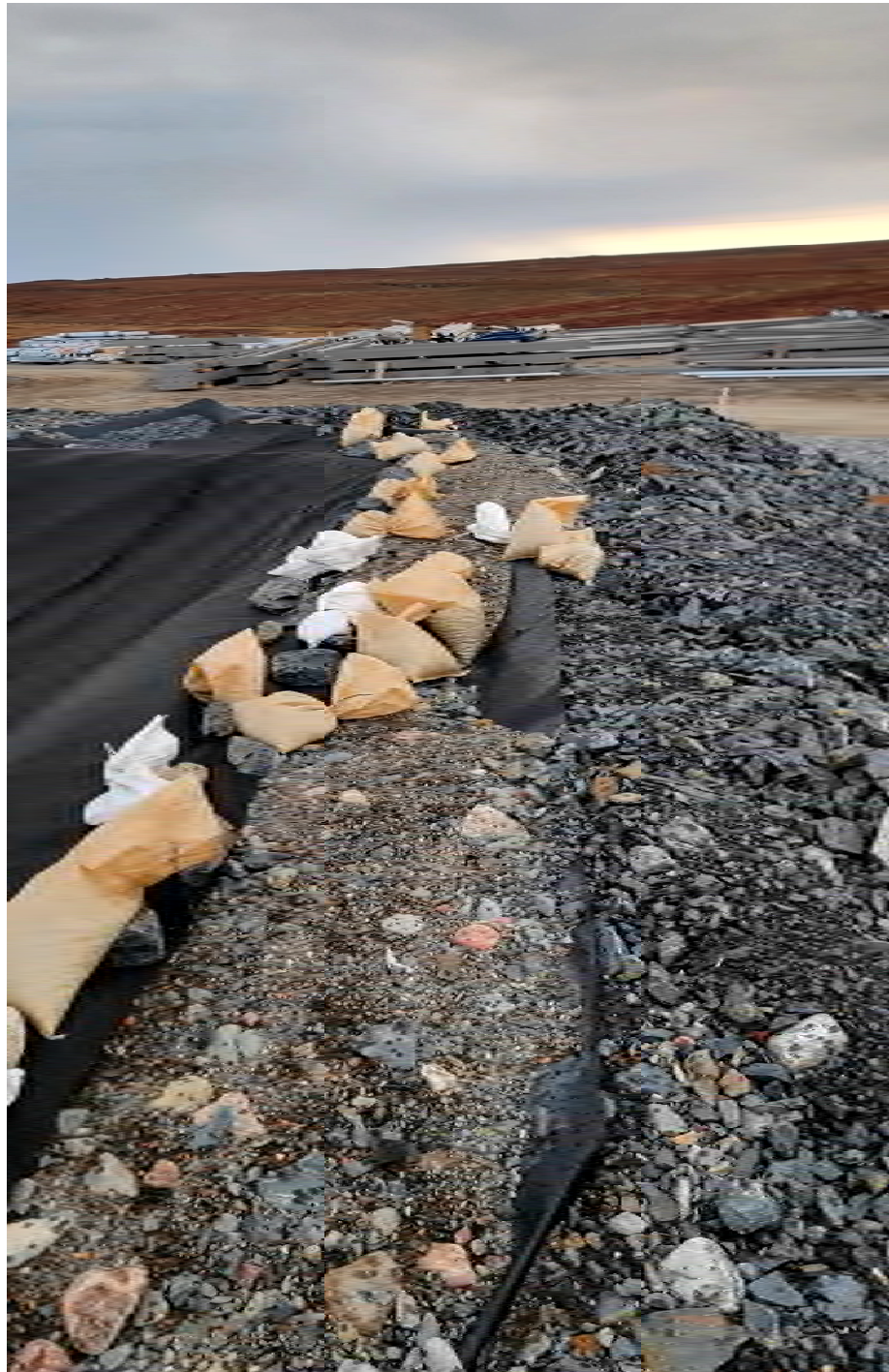
G-37 . – Edge of the HDPE liner is exposed on top of the SW corner of the berm, looking south
