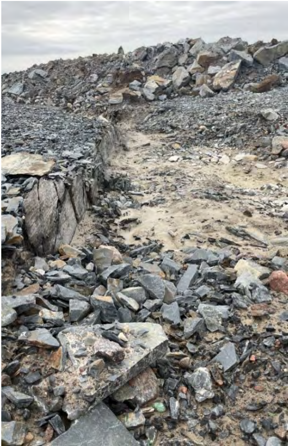
G-71. - Bedrock – overburden contact at the base of the spillway
