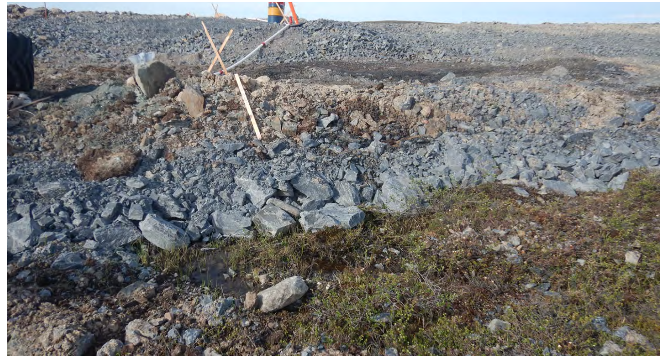
G-54. – Ponding water at the downstream side of the key trench approx. at Sta 0+550
