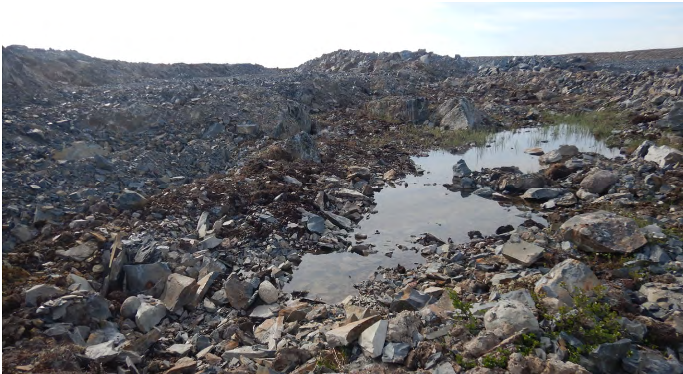
G-53.- Ponding water at the upstream side of the key trench approx.at Sta 0+250
