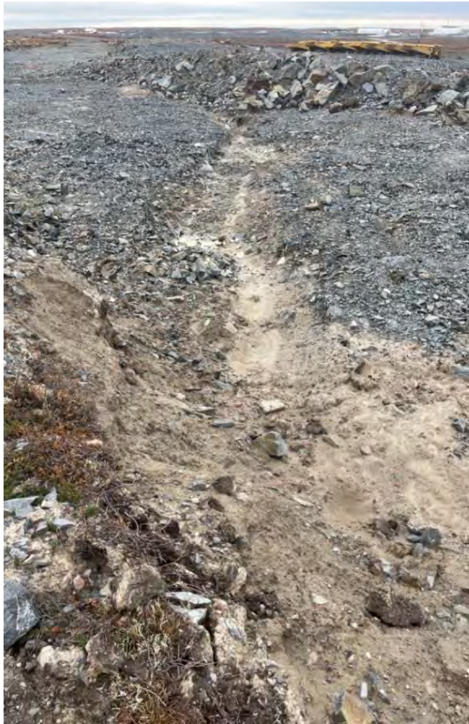
G-69. - Erosion channel at the base of the spillway close to the northern end
