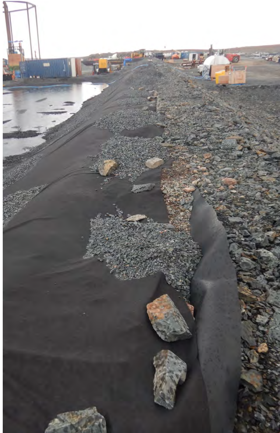
G-38. – Edge of the HDPE liner is exposed on top of the southern berm, looking east
