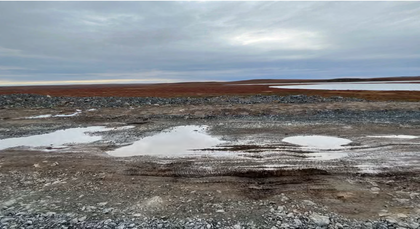
G-73. - Road embankment undulation
