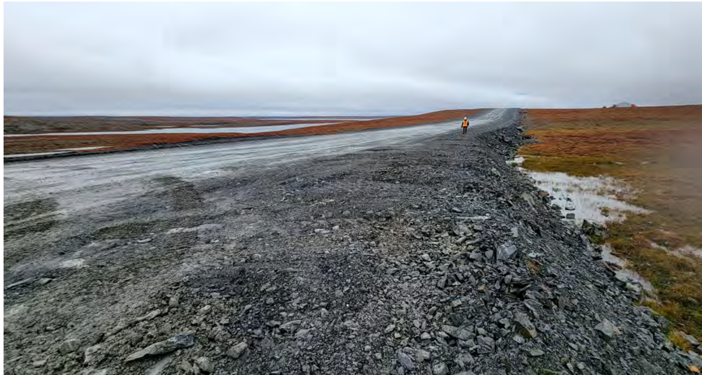
G-92. – Outlet location. An outlet was buried under the engineering fill. Note the thickness of the fill material
