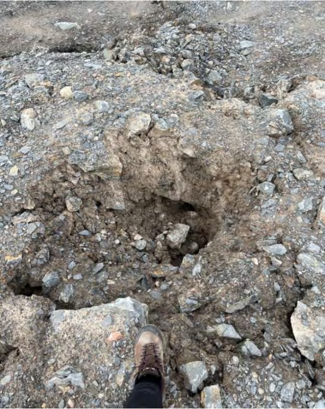
G-58 and G-59. - Embankment degradation approx. at Sta 0+260.
