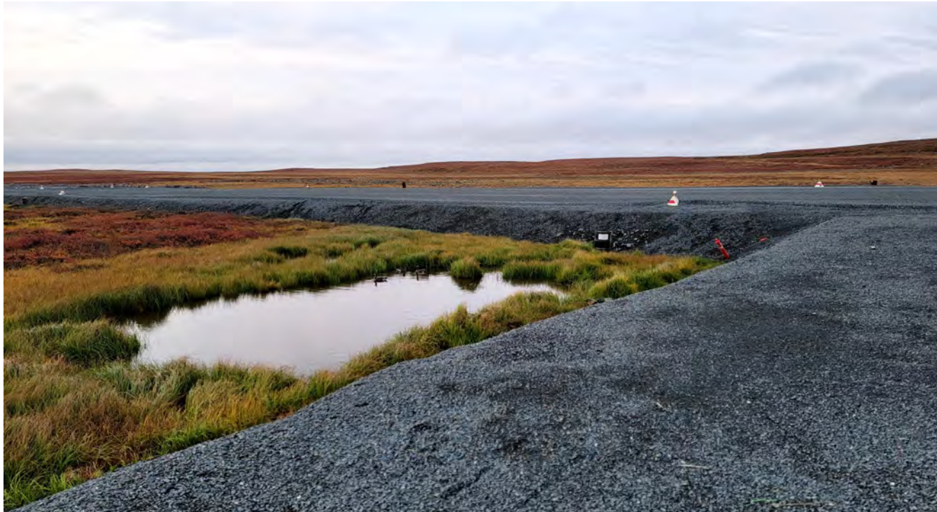
G-140. – Ponding waters on the eastern side of the pad, looking north. Note the thickness of the pad
