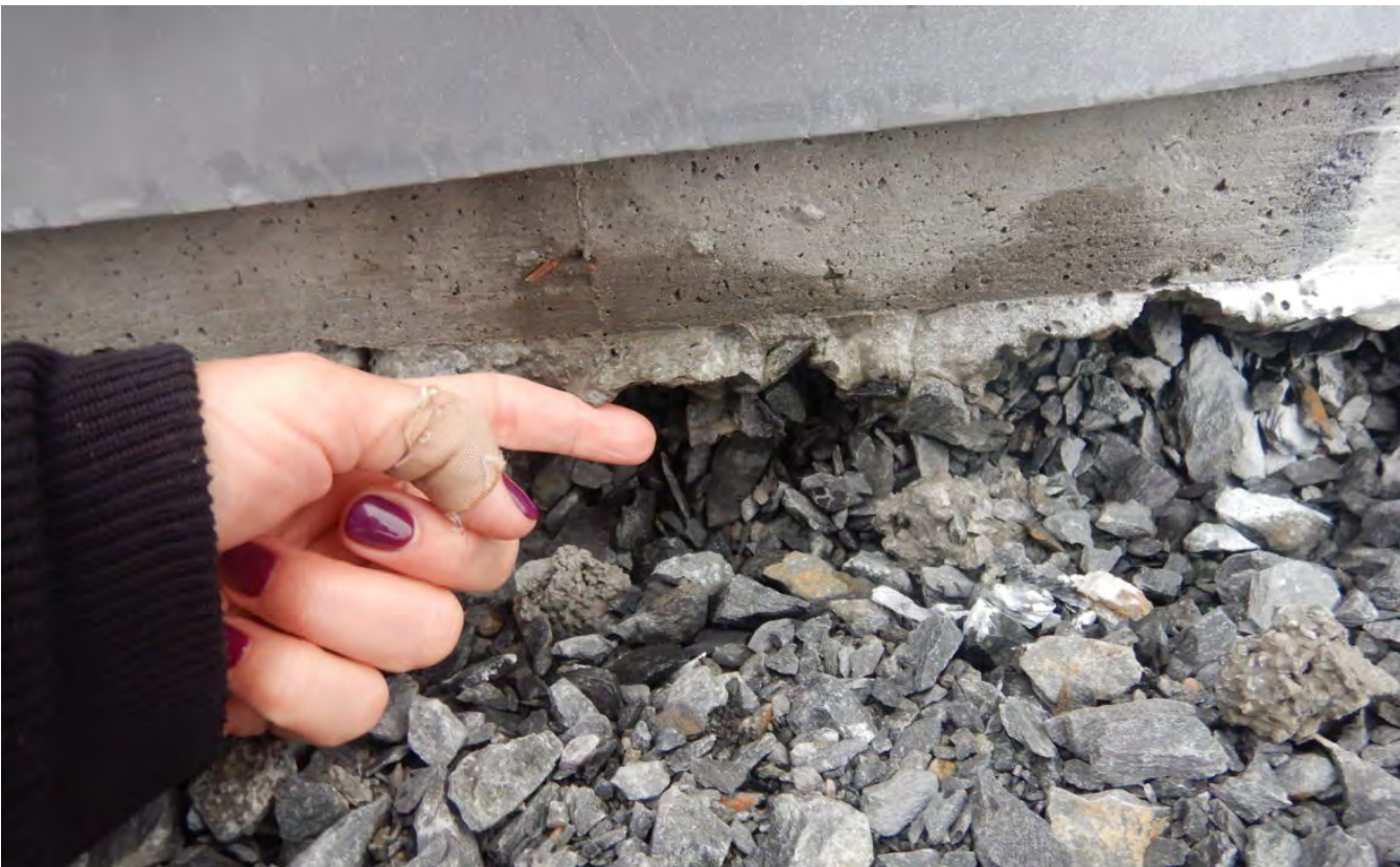
G-128. - Some voids observed between the footing and the fill material
