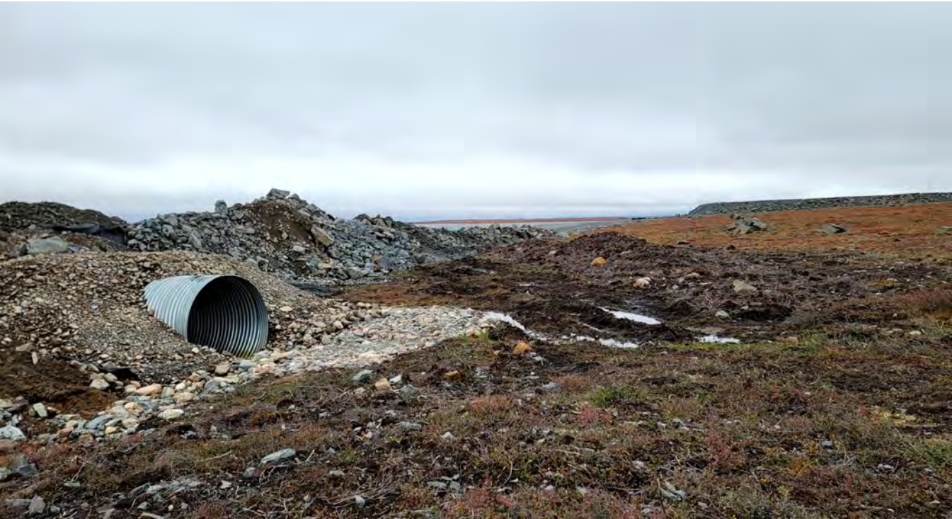
G-102. Culvert #3: Outlet. Note the tundra degradation around the outlet
