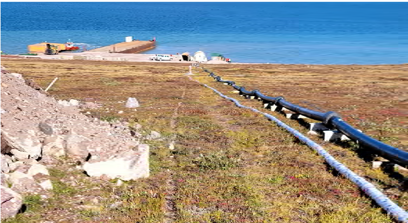
M-12. – Pipelines go from the Camp area to the Shoreline Pad. Note that the pipe connections are in between wooden blocks
