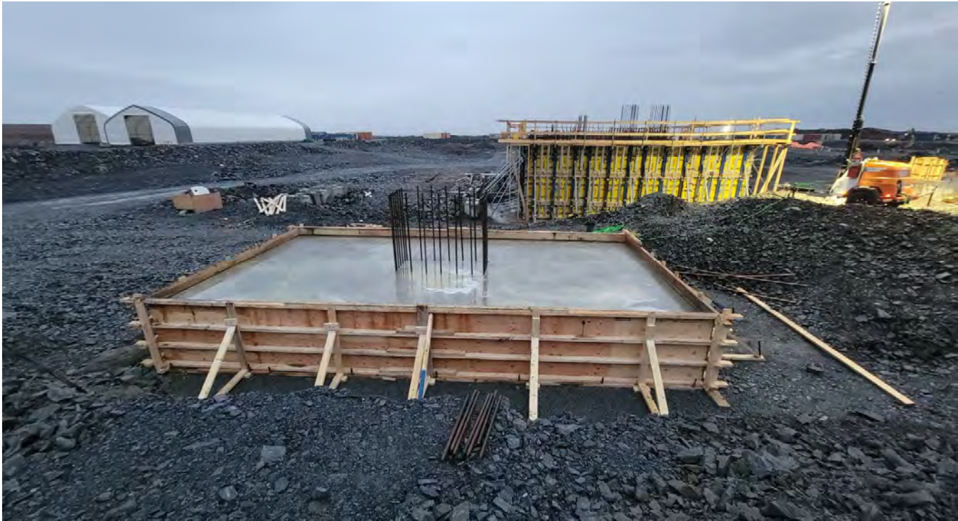
G-123. – Processing Plant: construction od the footings
