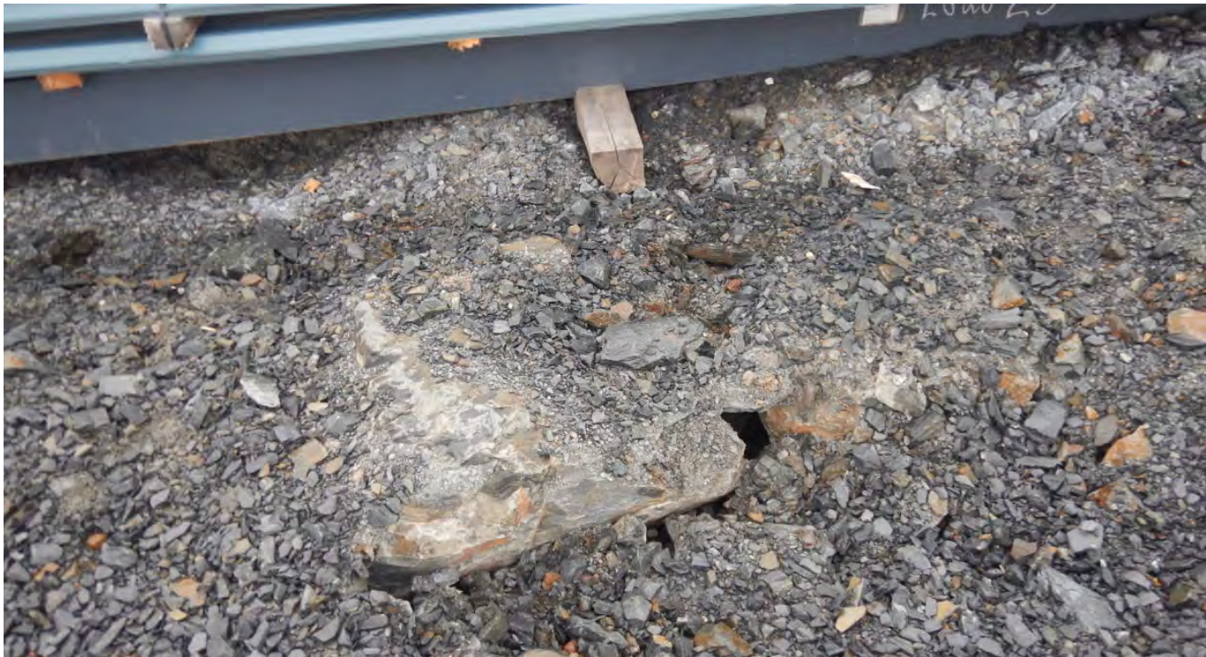
G-134. - Southern slope of the Plant Site Pad, looking north. Note some voids in the fill material
