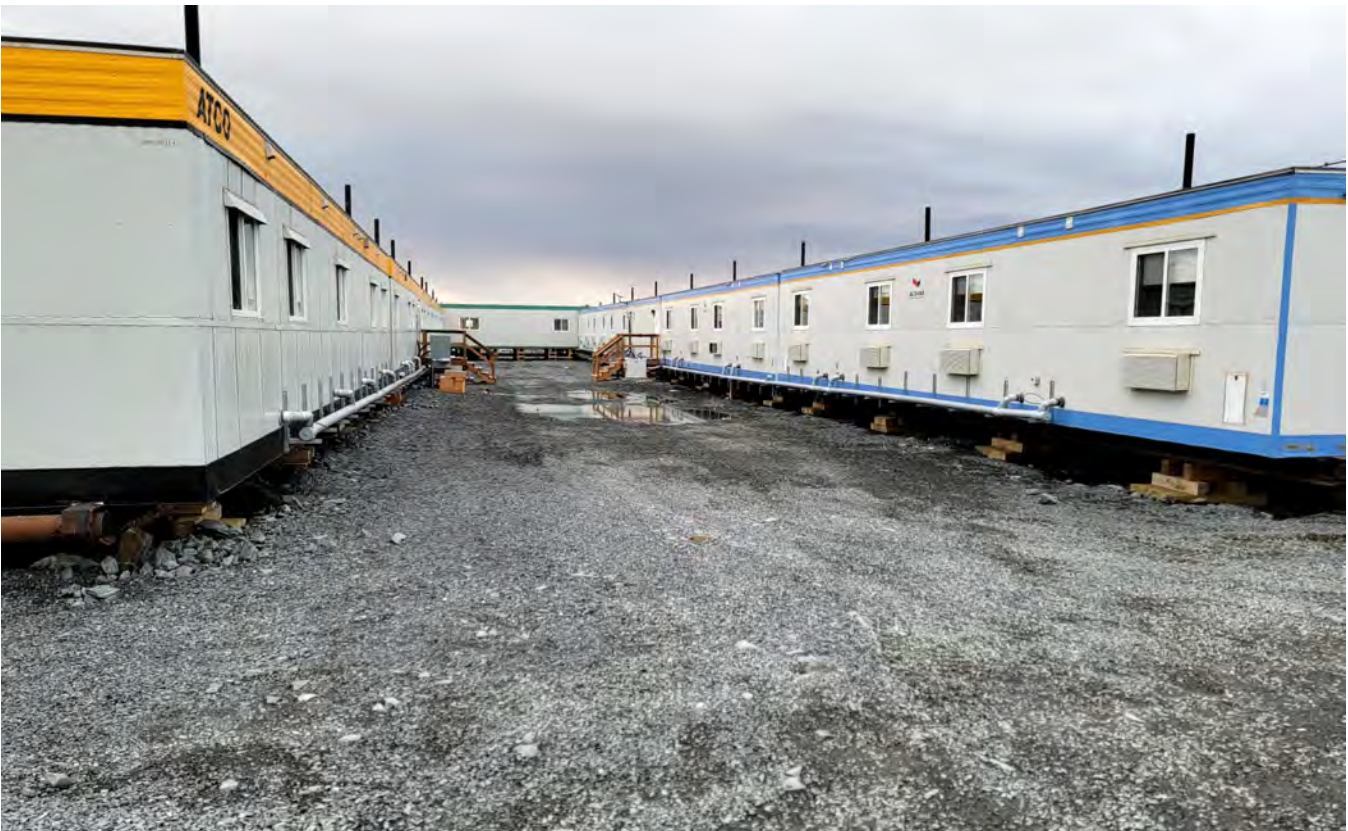
G-111. – All dormers have been mounted onto the wooden foundation to allow airflow below the buildings
