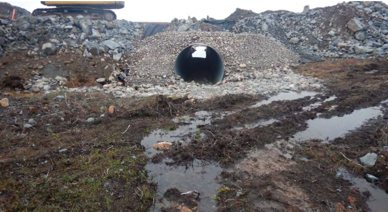
G-104. Culvert #3: Outlet. Note the thickness of the overculvert fill
