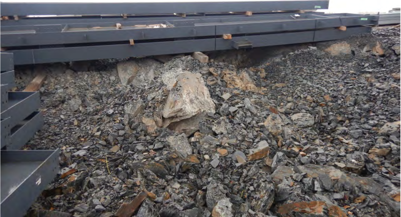
G-131. – Southern slope of the Plant Site Pad, looking north. Note some voids in the fill material
