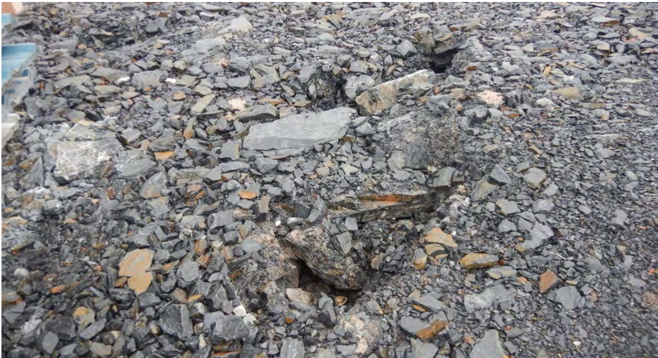
G-135. - Southern slope of the Plant Site Pad, looking north. Note some voids in the fill material
