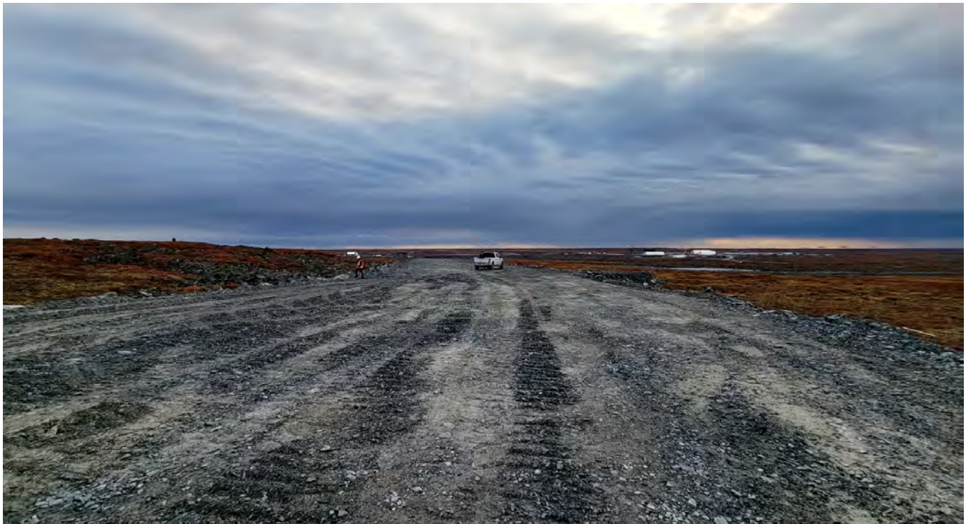
G-159. - Example of the fill material used for road construction. The photo was taken looking south
