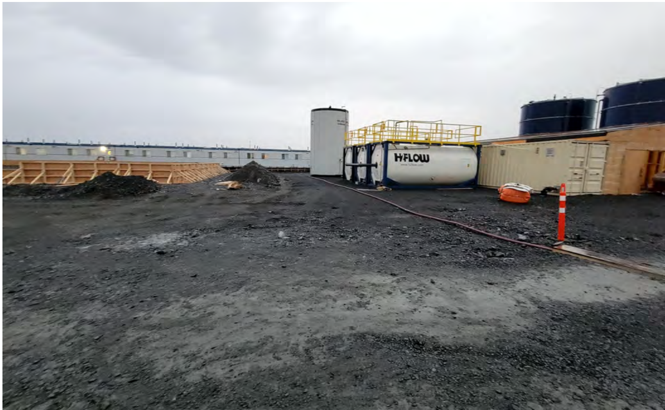
G-109. – Warehouse construction is in progress. Example of the fill material used in the pad construction
