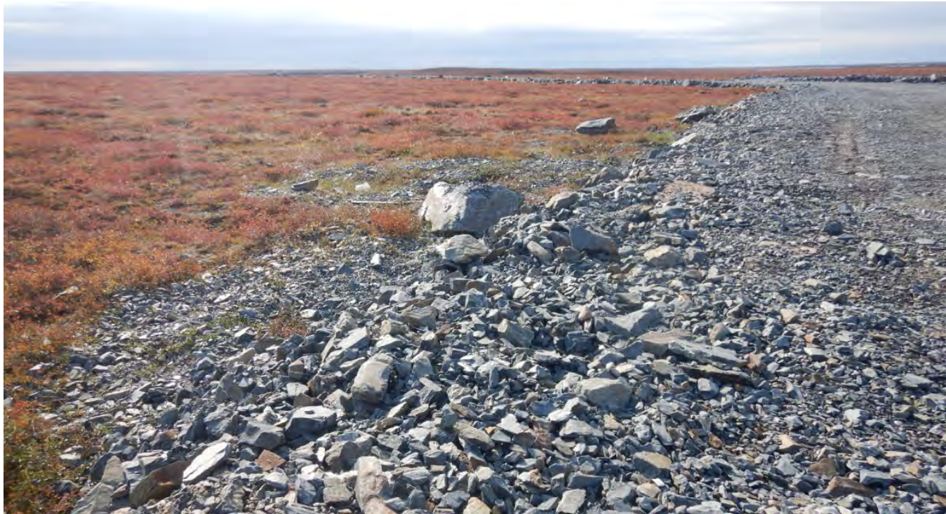
G-177. – Southern edge of the temporary access road, looking north, note thickness of the pad
