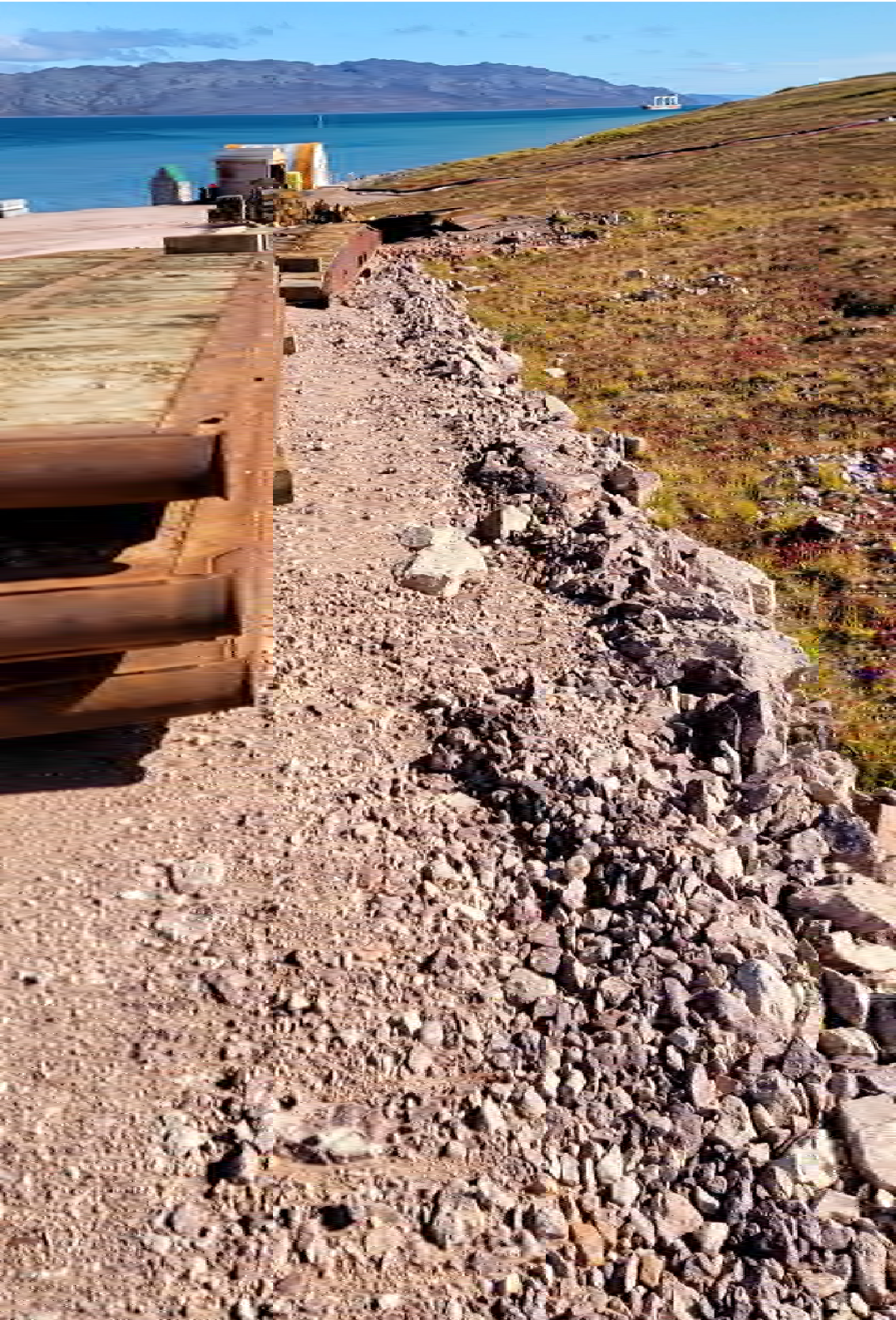
M-10 Southern side of the Shoreline pad looking northeast. Note the thickness of the fill material
