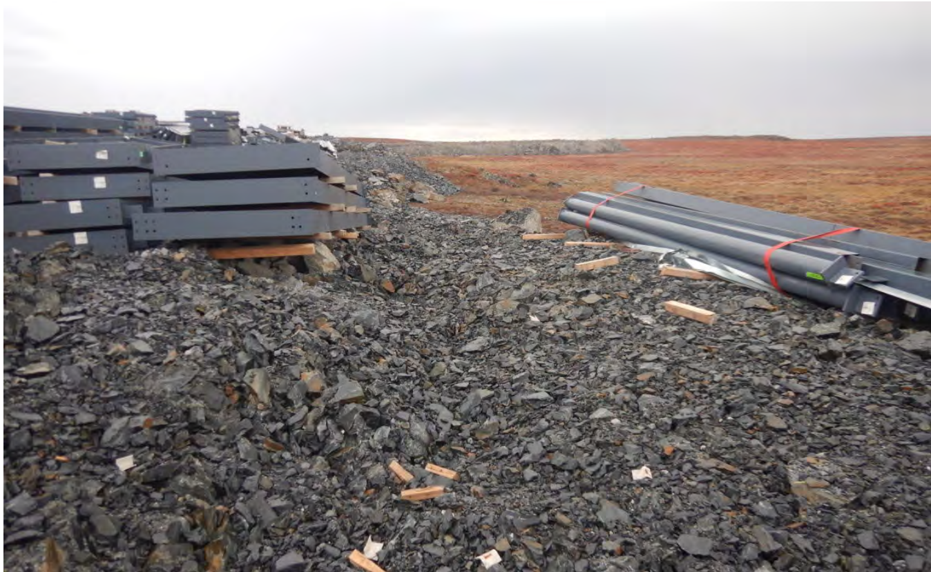
G-129. – Southern slope of the Plant Site Pad, looking east. Note that stored materials are placed too close to the edge of the pa
