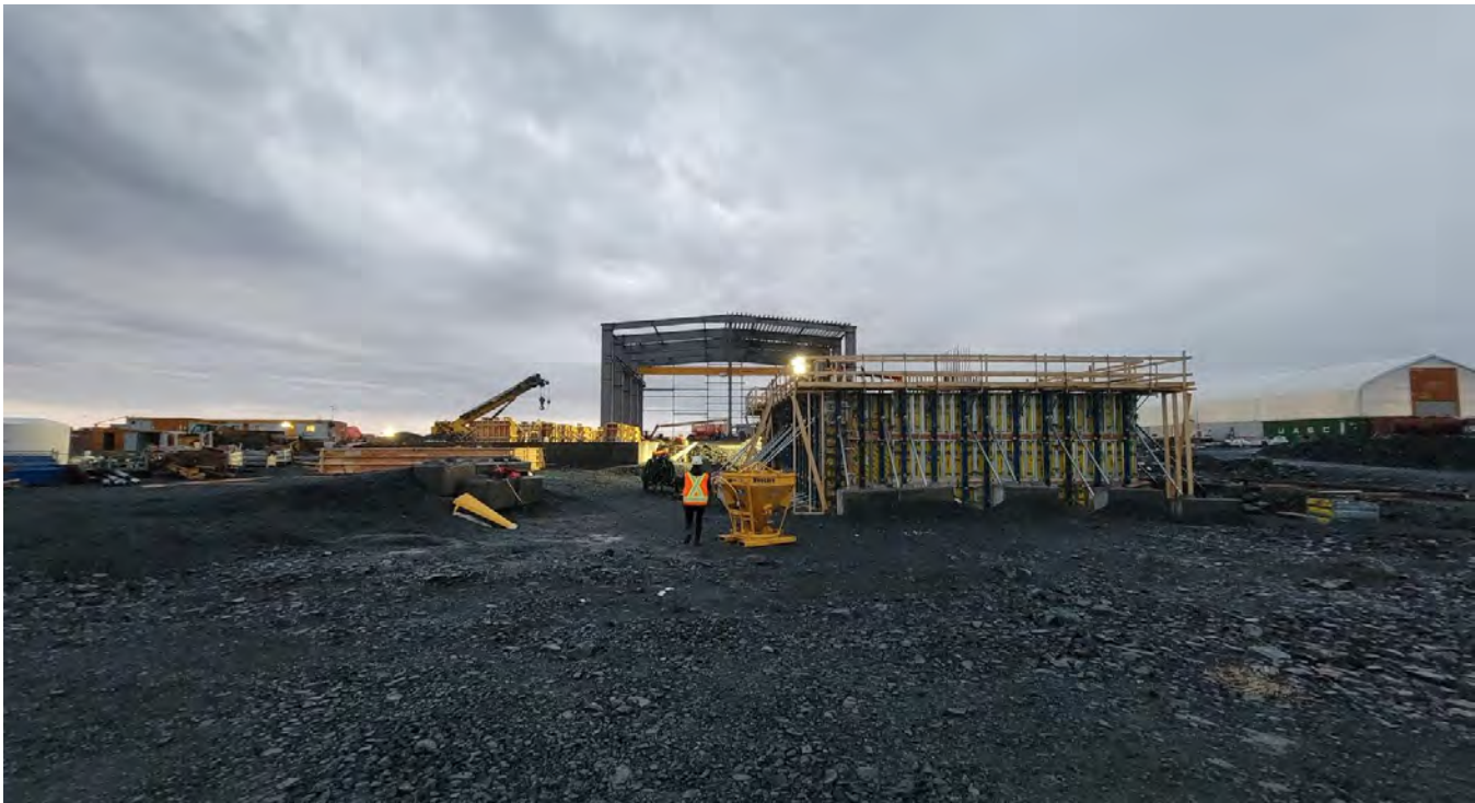
G-125. – Processing Plant: construction od the footings
