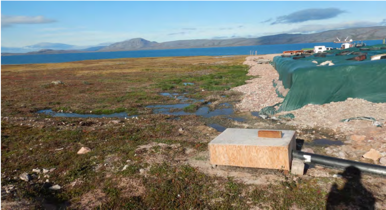
M-16. – Discharge point at the eastern corner of the Freight Storage Pad. Note ponding waters along the east side of the Pad
