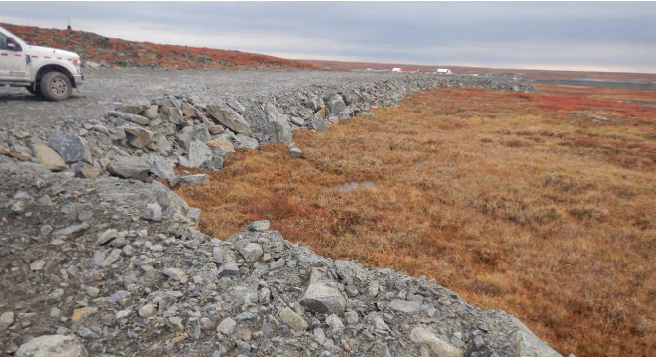
G-158. - Northern end of the road. Note the thickness and the slope of the embankment.
