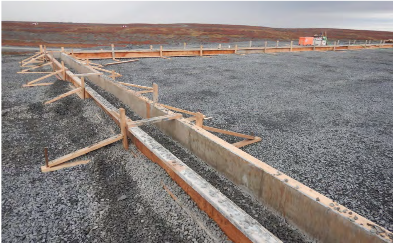
G-126. – Construction of the tent foundation
