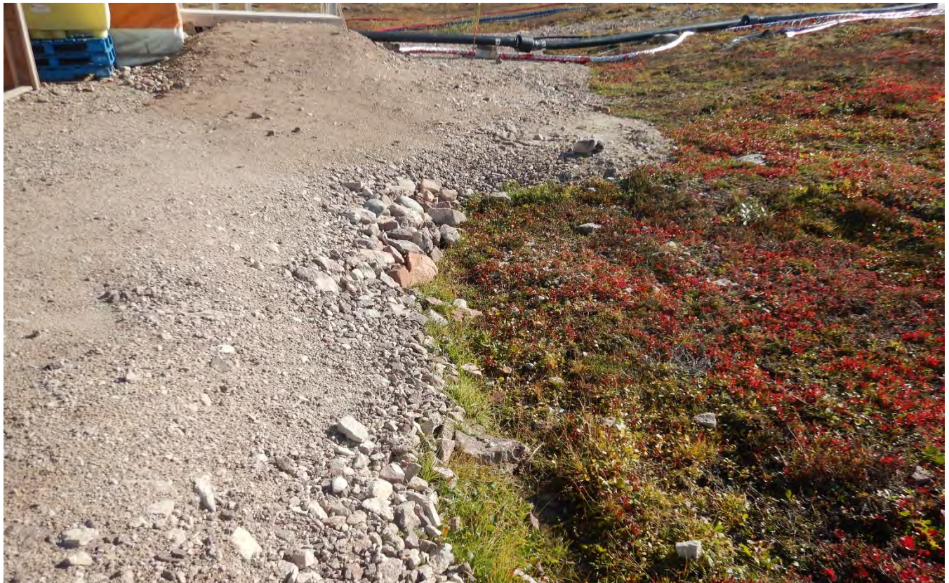
M-11 Southern side of the Shoreline pad looking southeast. Note the thickness of the fill material is less than 0.5m
