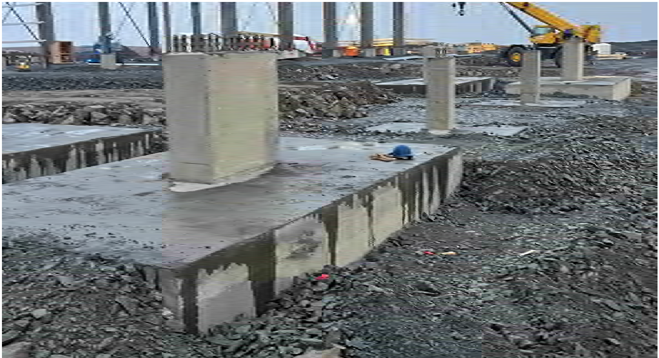
G-124. – Processing Plant: construction od the footings
