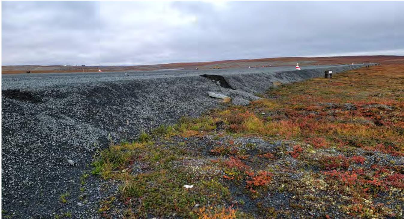
G-149. - Eastern side of the pad, looking NW, note the thickness of the pad and erosion gullies
