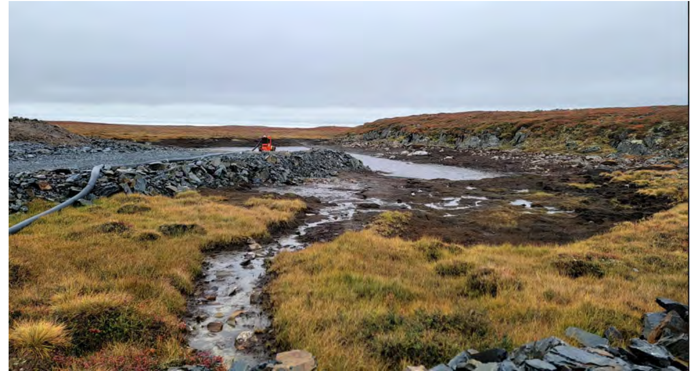
G-106. – A pond at the toe of the diversion berm and discharge point of the drainage water from Echo Pit
