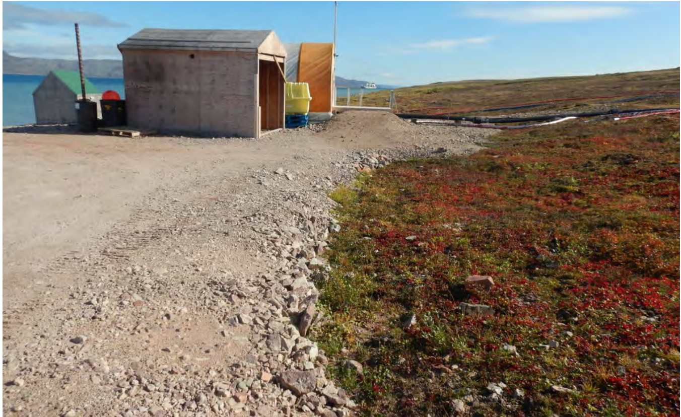
M-8 Southern side of the Shoreline pad looking southeast. Note the thickness of the fill material
