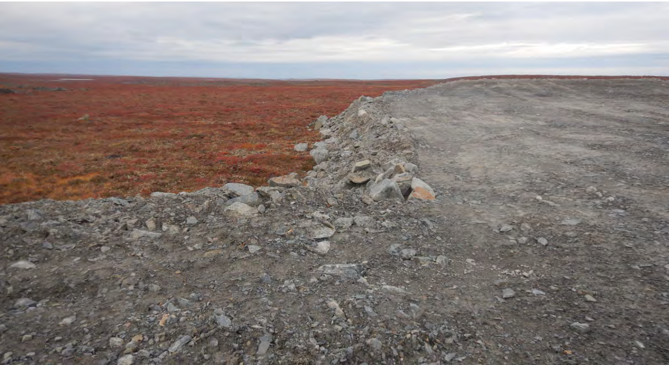
G-160. - Example of the fill material used for road construction. The photo was taken looking south
