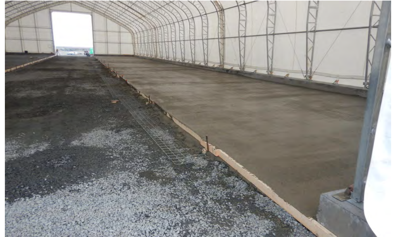
G-127. – Base of the tent: pored concrete
