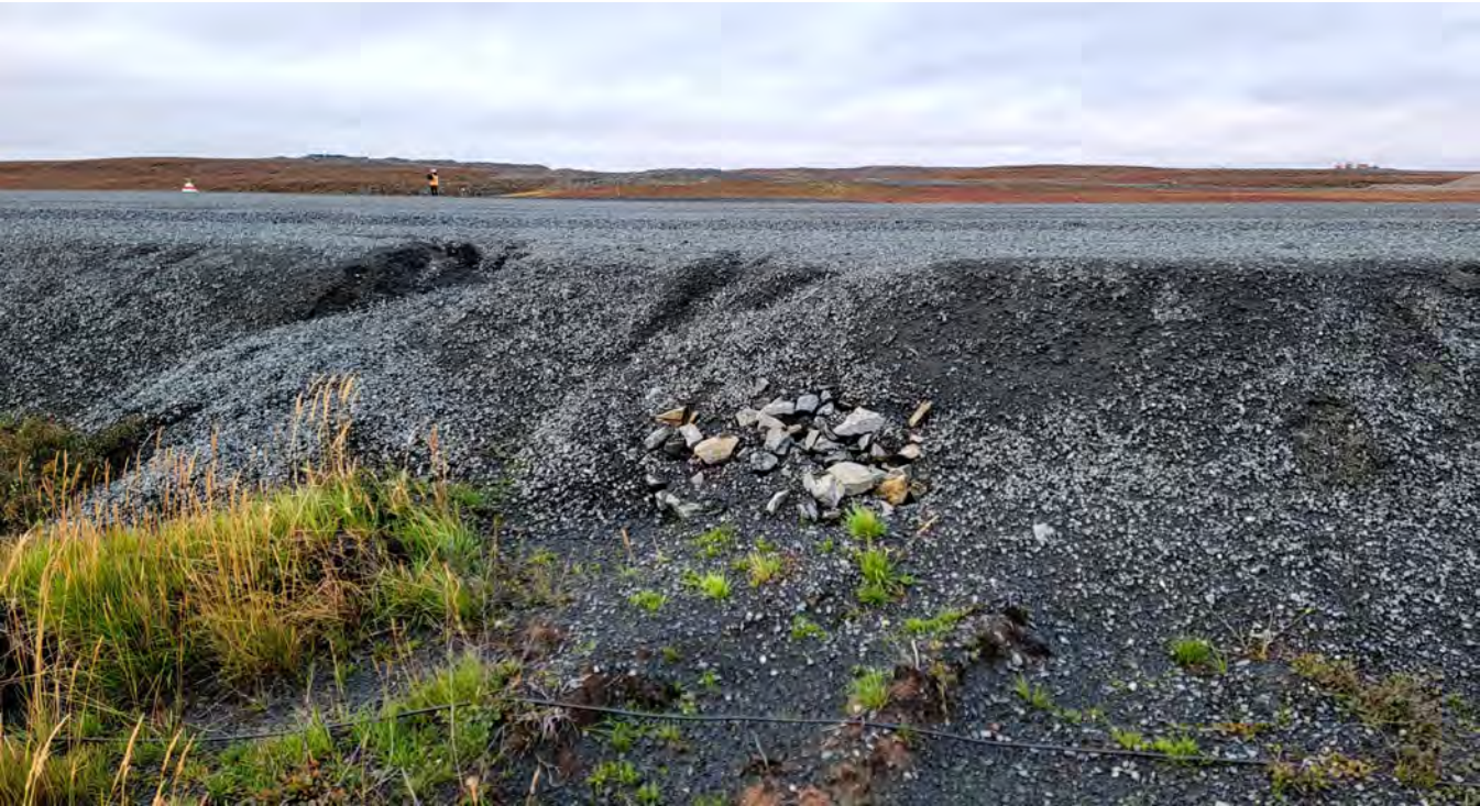
G-150. – Erosion gullies on the eastern side of the pad, looking south
