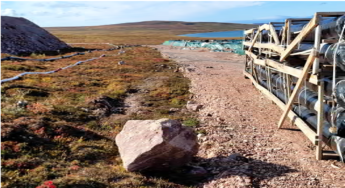
M-18. – Northeast side of the Freight Storage Pad. Note that the fill thickness is less than 0.15m
