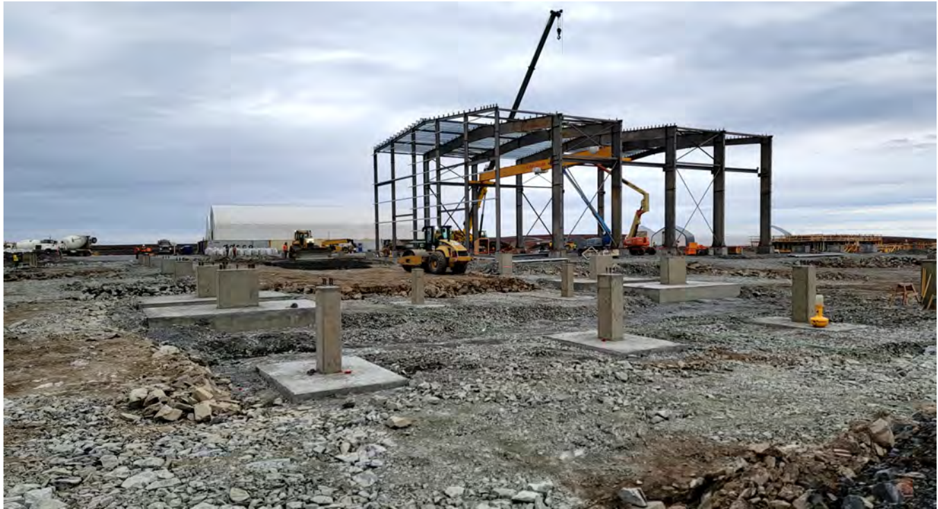
G-122. – Processing Plan: construction of the footings
