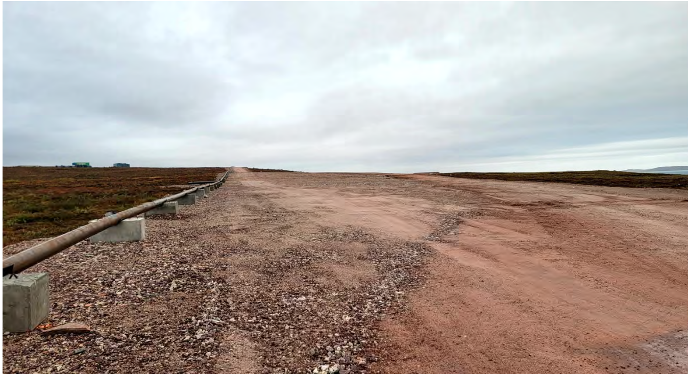
M-88. – Fuel Offload Access road. Note that the edges of the road lack proper compaction of the fill material.
