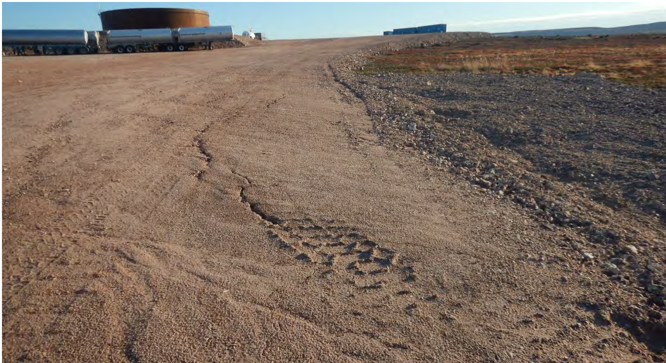
M-40. – Former Explosives Storage Berm. Note cracks along the road edge.
