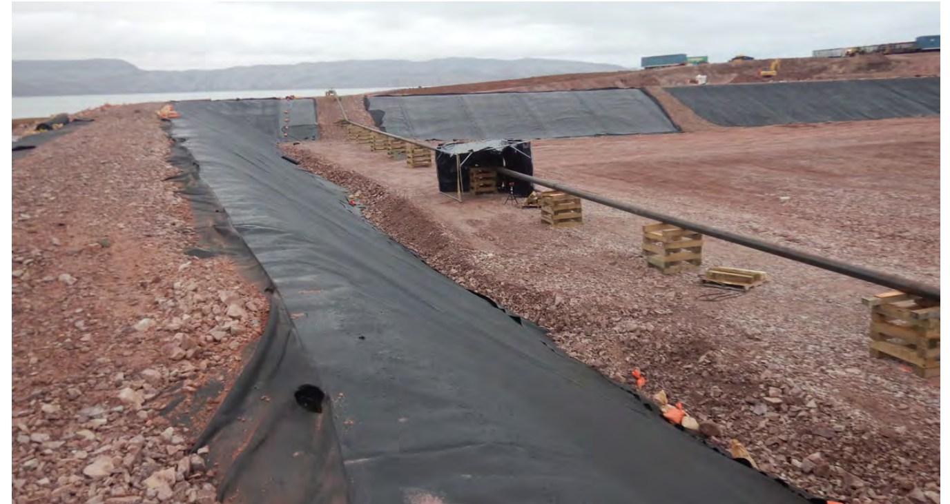
M-61. – Northern and western inner slopes. Note that the slopes are oversteepened (approx. 1.5H:1V) and not covered with the fill material.
