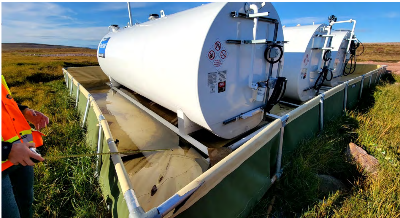
M-42. – Insta Berm with three empty fuel tanks. Note ponding water at the base of the containment area
