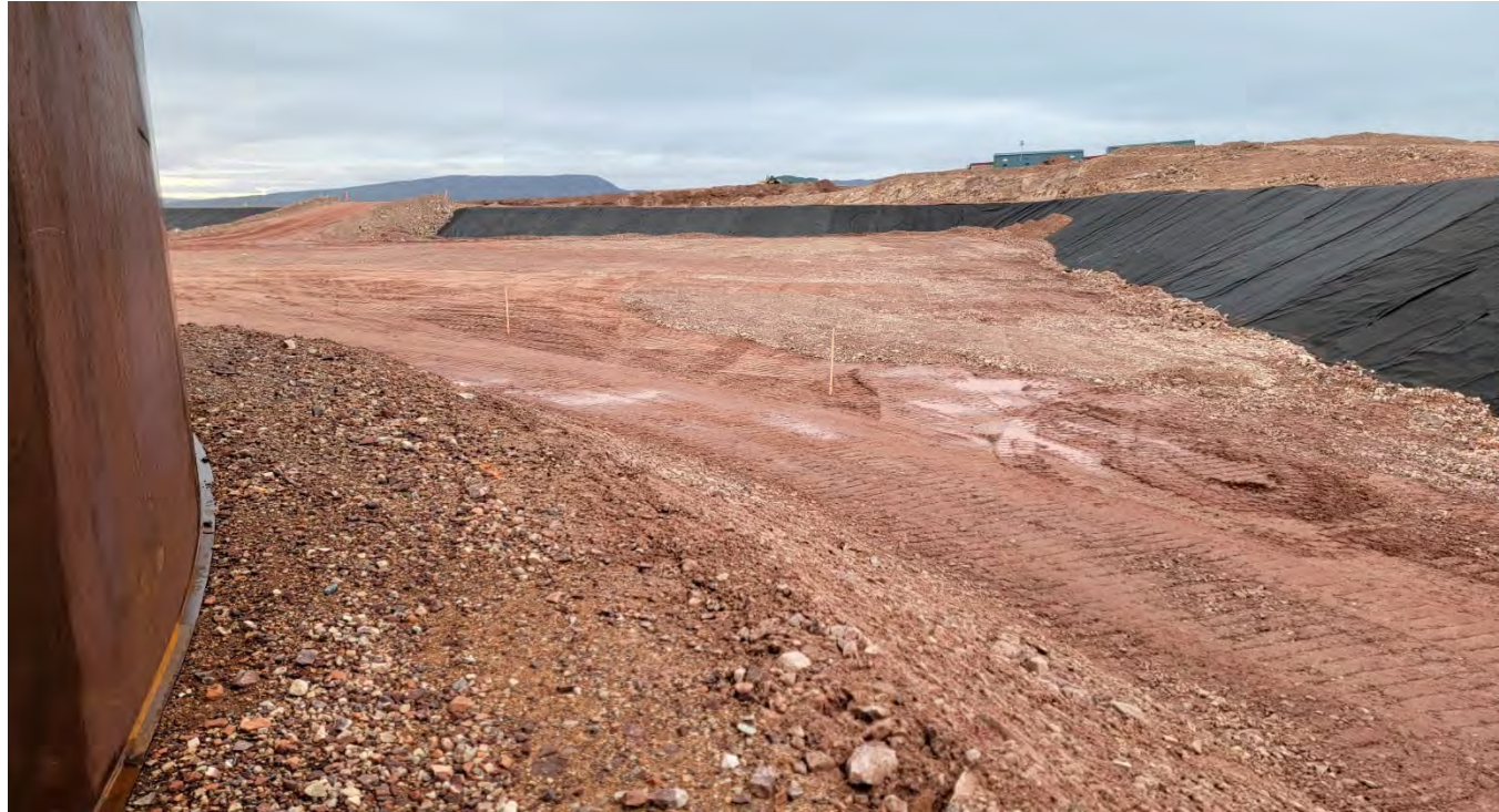
M-65. – Tank #2 pedestal. Southern slope and berm, looking NE. Note some cracks at the crest.
