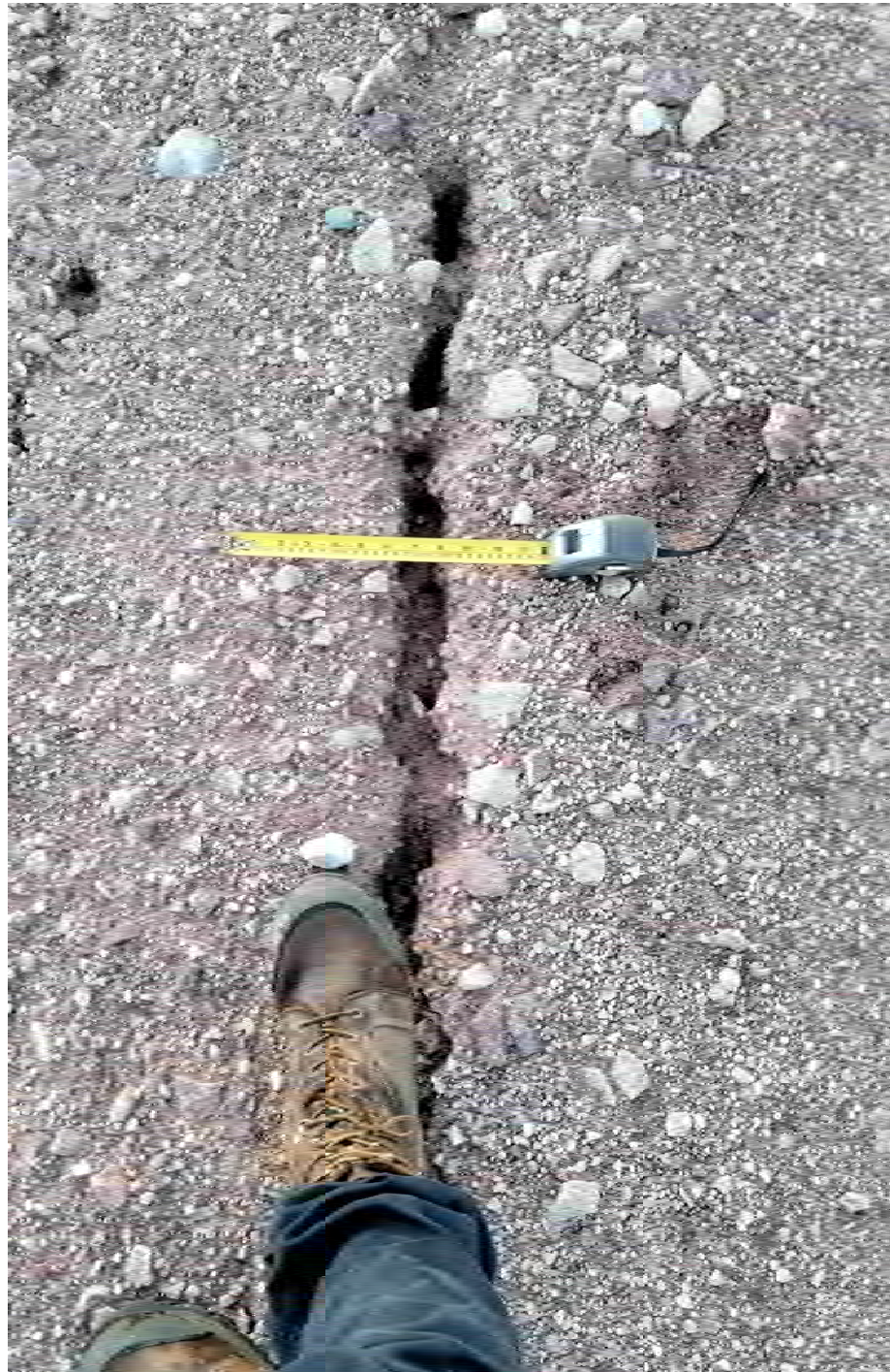
M-50a. – SE End of the airstrip. Note that the crack width is 2-2.5 inch
