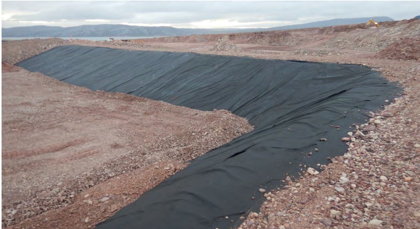
M-60. – SE corner and eastern berm of the containment area. Note that the HDPE liner is not backfilled.
