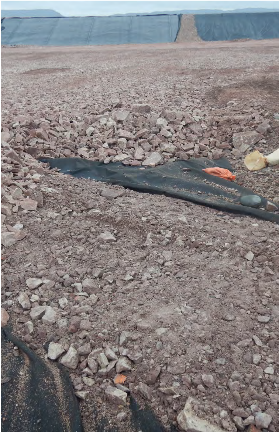
M-76. – Exposed Geotextile and HDPE liner at the base of the containment area.
