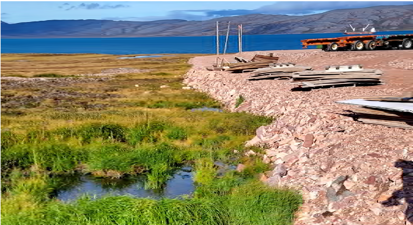
M-22. – Eastern side of the Freight Storage Pad. Note ponding waters along the toe of the pad
