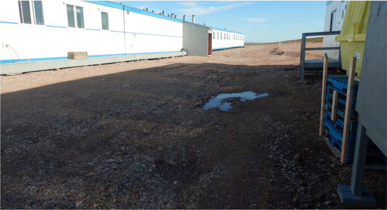
M-28. – Surface undulation at the Camp Pad.
