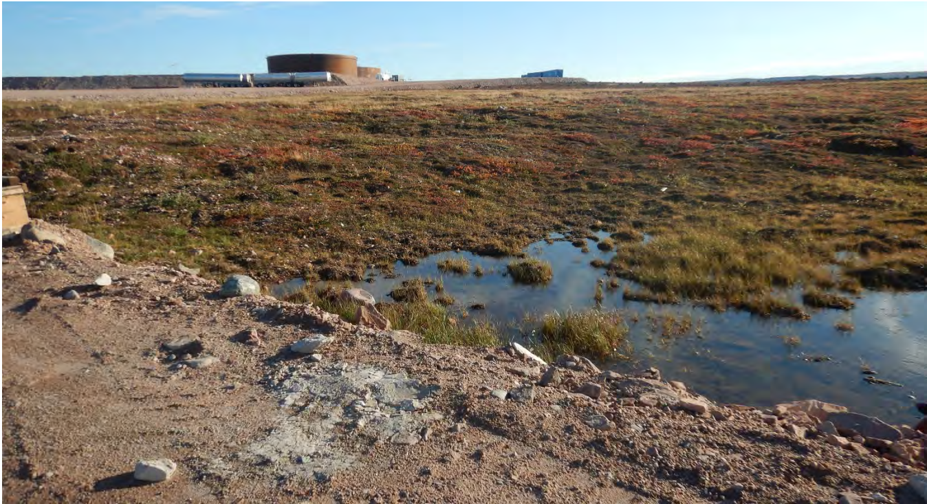
M-39 Former Explosives Storage Berm. Note ponding waters along the toe of the embankment
