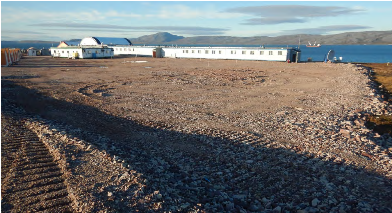
M-33. – Southern extension of the Camp Pad looking north. Note the uncompact material and thickness of the pad.
