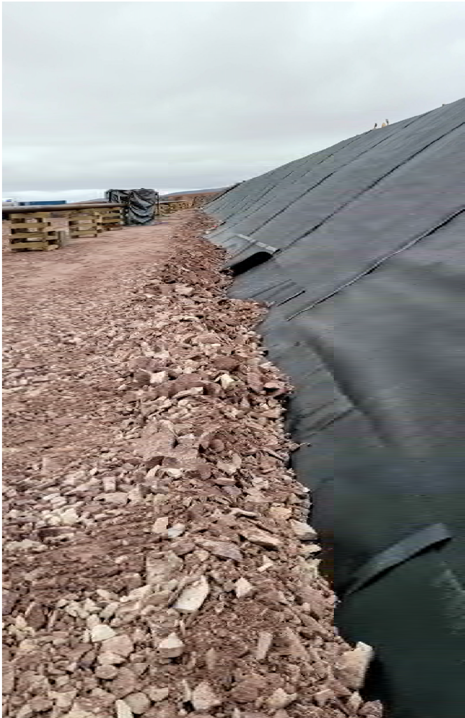
M-73. – Northern berm of the containment area. Note unwelded and unprotected HDPE liner panels at the toe
