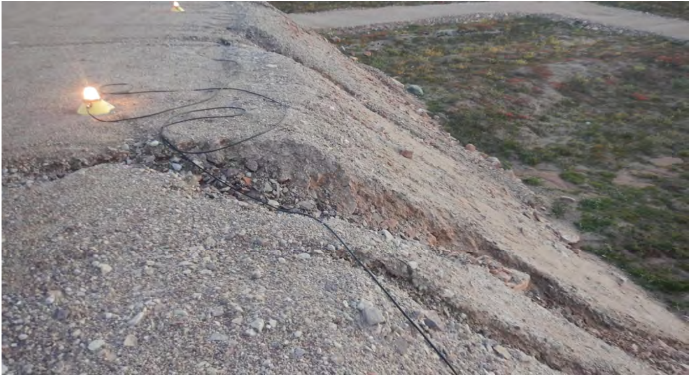
M-46a. – Erosion gullies at the NW end of the airstrip
