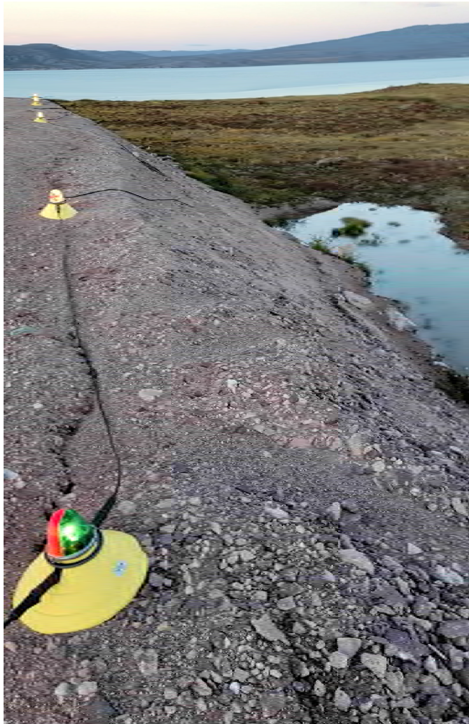
M-51. – SE end of the airstrip. Note ponding waters at the toe of the embankment and crack at the crest.
