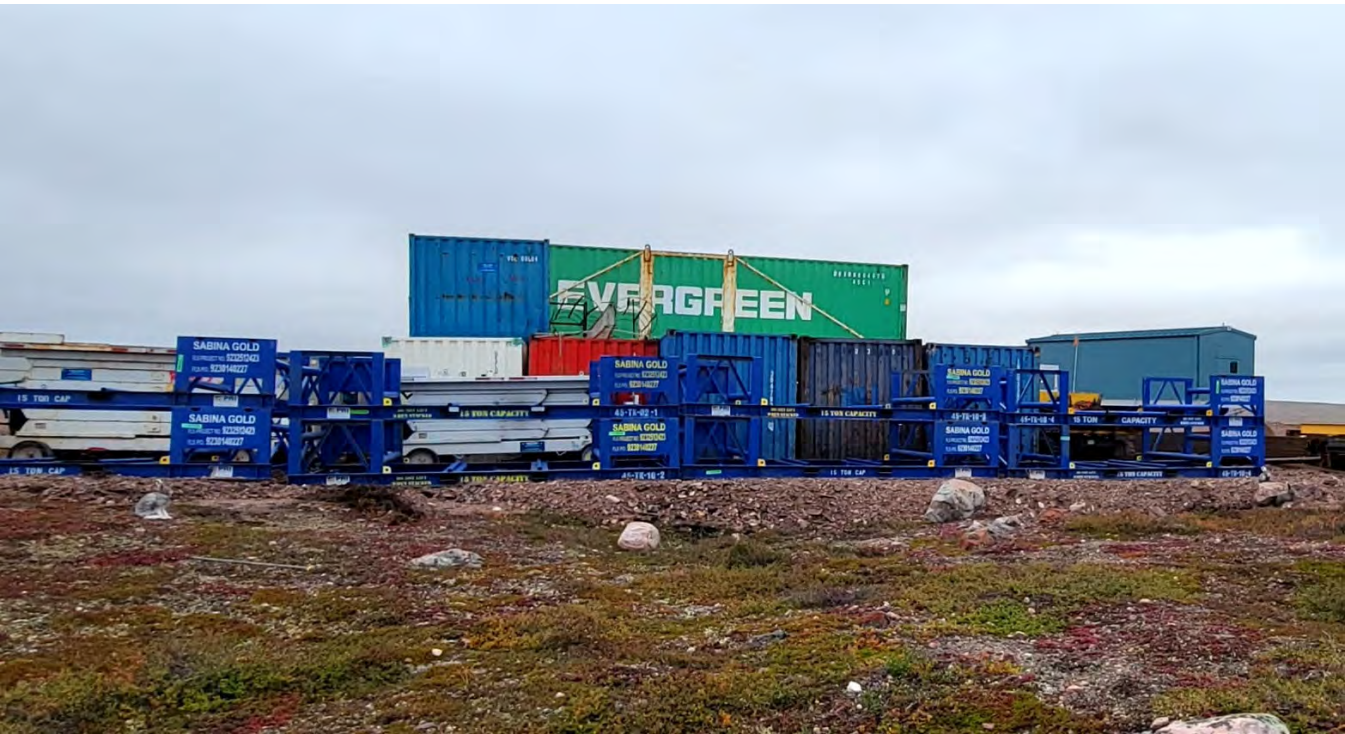
M-83. – Eastern side of the Upper laydown Area, looking NW. Note that the thickness of the pad is less than 1m and materials are stored to close to the crest.
