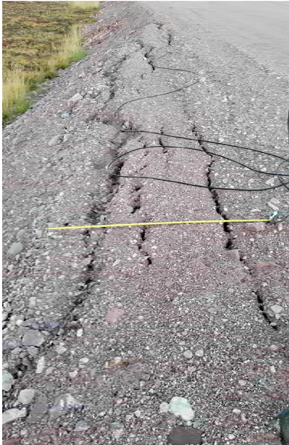
M-50. – SE end of the airstrip. Note a series of elongated cracks at the embankment crest.
