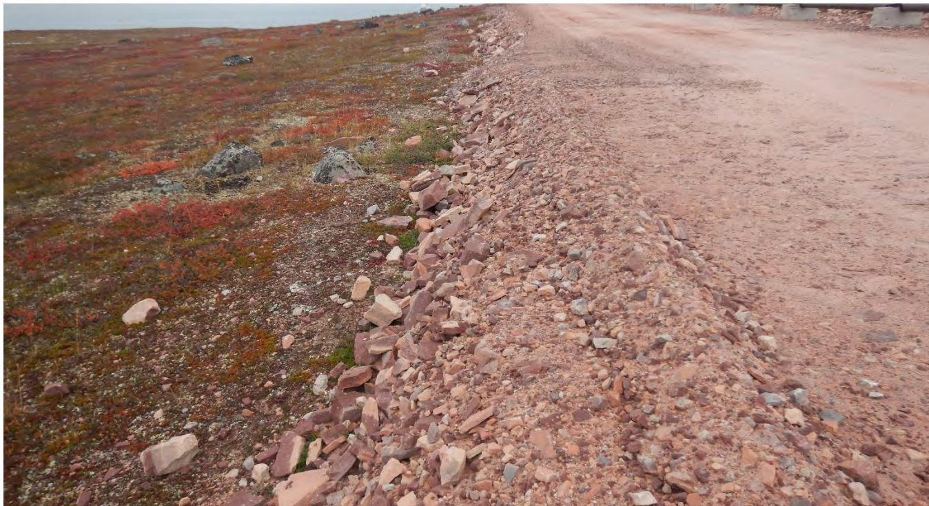
M-84. – Fuel Offload Access road. Note the thickness of the embankment
