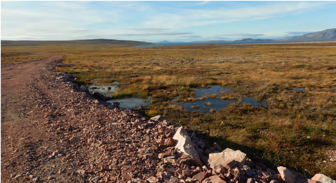
M-37. – Former Explosives Storage Berm. Note ponding waters along the toe of the embankment
