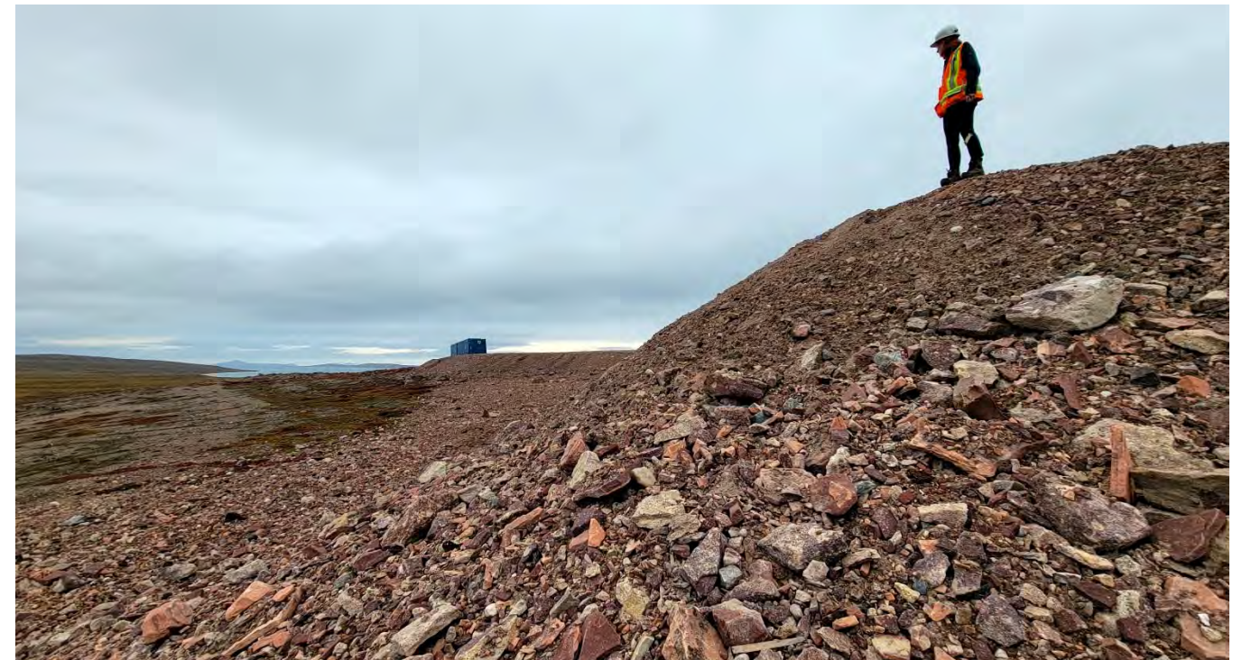
M-63. – Outer slope of the SW corner of the containment area. Note that the slope is oversteepened and has a height about 4 m
