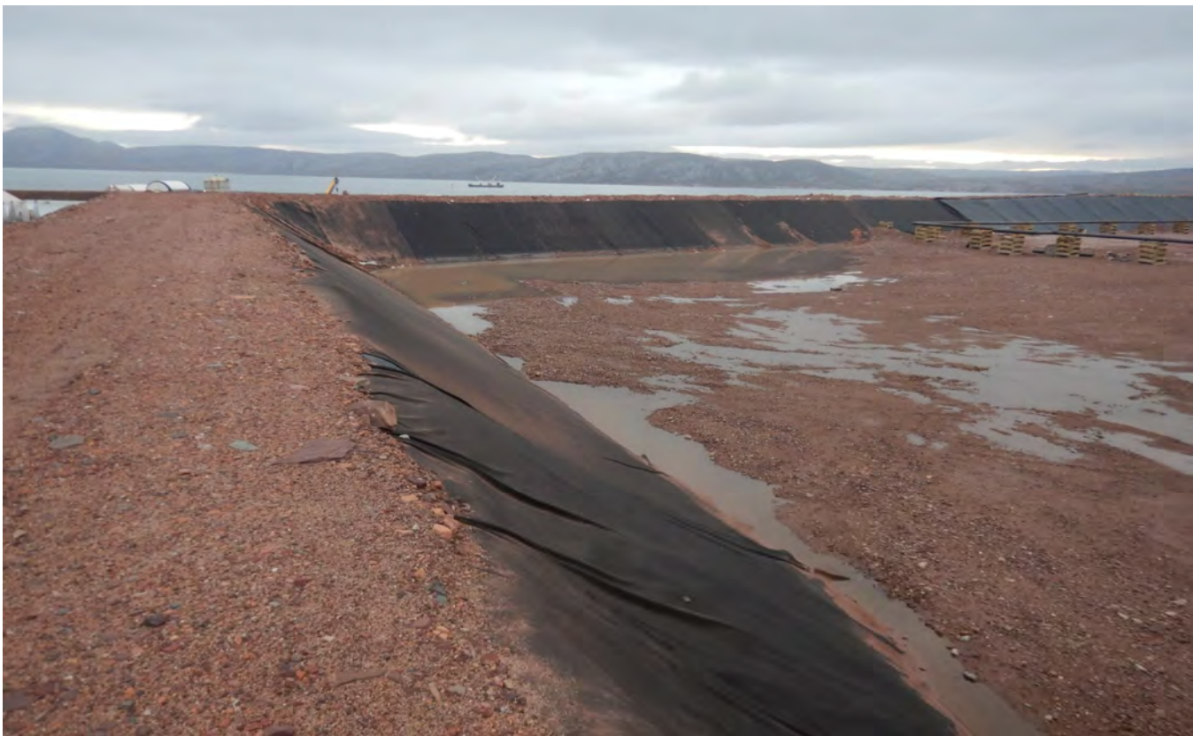
M-57. – Ponding water at the base of the NW corner and along the toe of the western berm of the containment area, looking NE.
