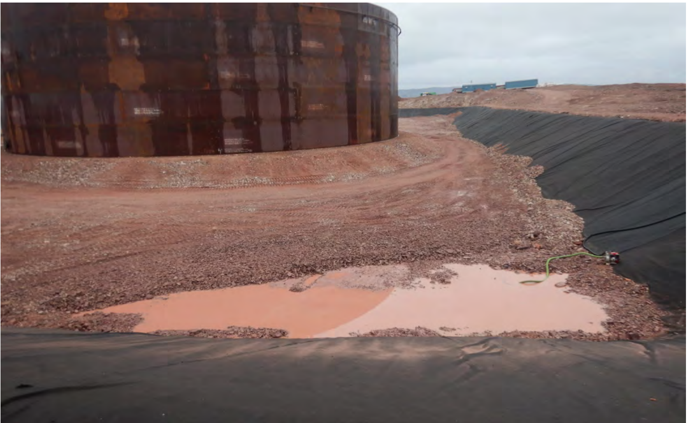
M-58. - Ponding water at the base of the SW corner of the containment area, looking NW.
