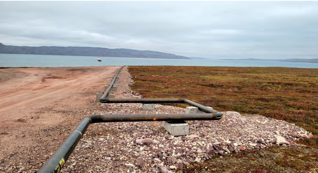
M-87. - Fuel Offload Access road. Note the thickness of the embankment
