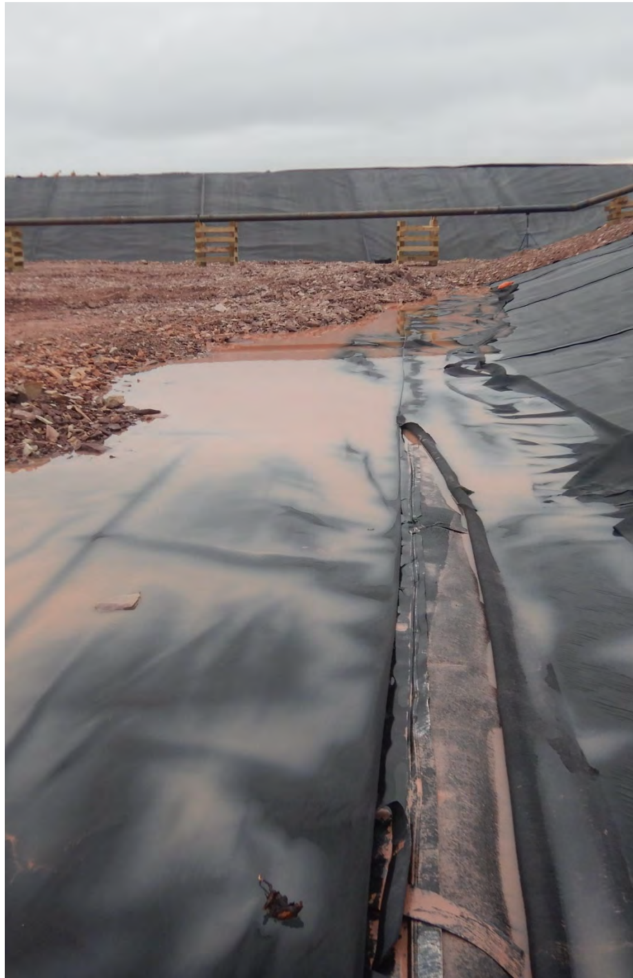
M-74. – exposed liner at the toe of the eastern berm
