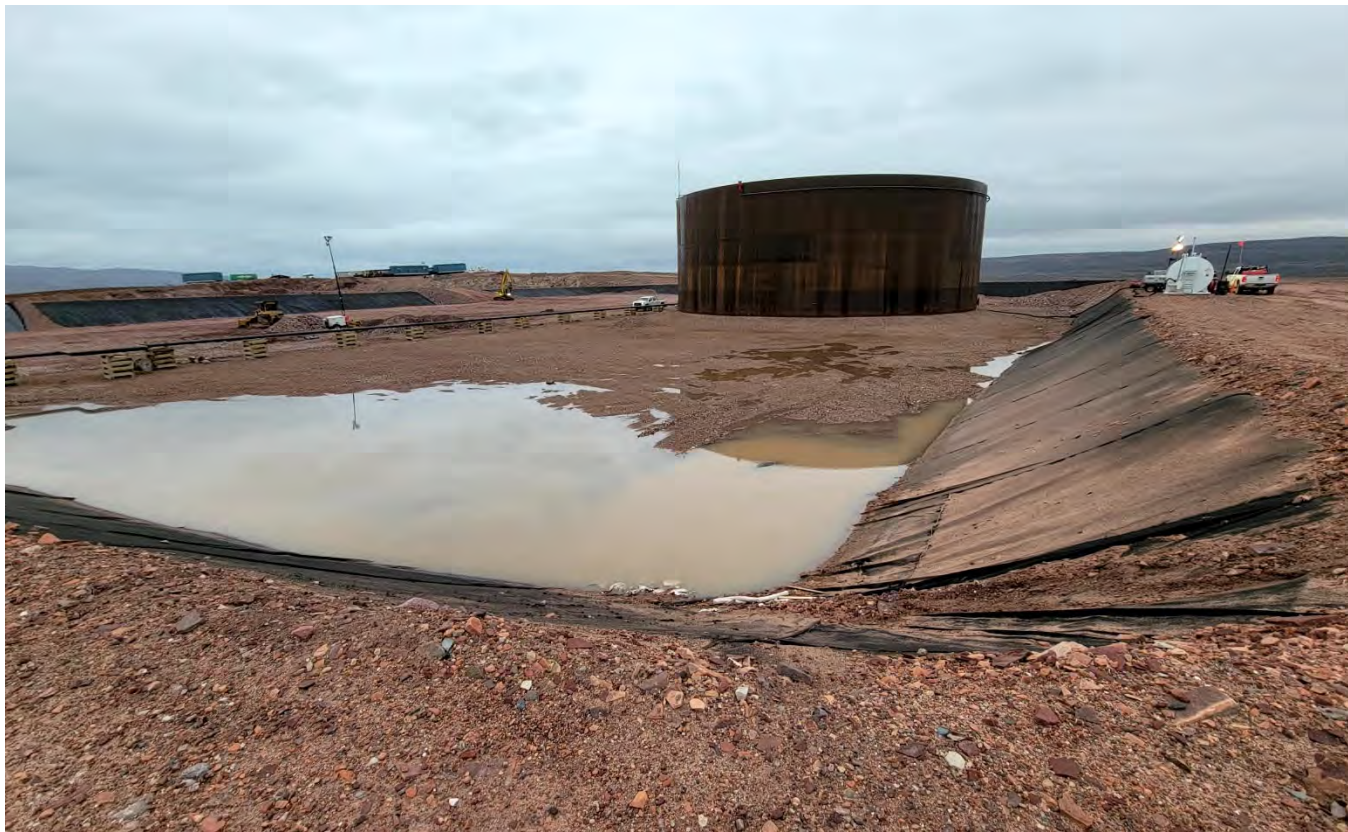
M-56. – Ponding water at the base of the NW corner of the containment area, looking south.
