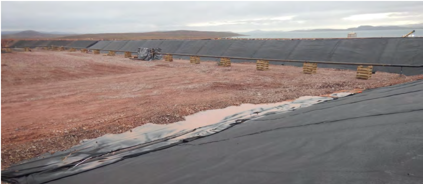
M-59. – Ponding water at the base of the NE corner along the toe of the western berm of the containment area, looking N.
