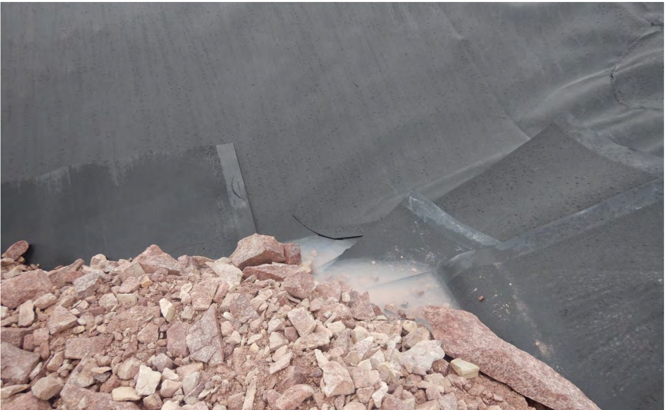
M-79. – NE corner of the containment area. Note unwelded and unprotected HDPE liner panels at the toe.
