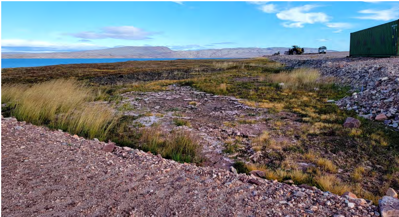
M-21. – Northern corner of the Freight Storage Pad. Note some ponding water signs at the lower points between access road and the pad
