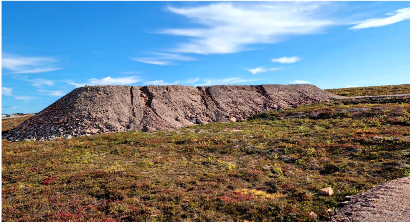
M-46. – Set of deep erosion gullies at the NW end of the airstrip
