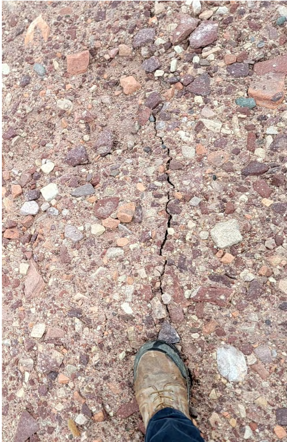
M-72. – Southeast berm of the containment area. Note that the fill material cracking at the crest.
