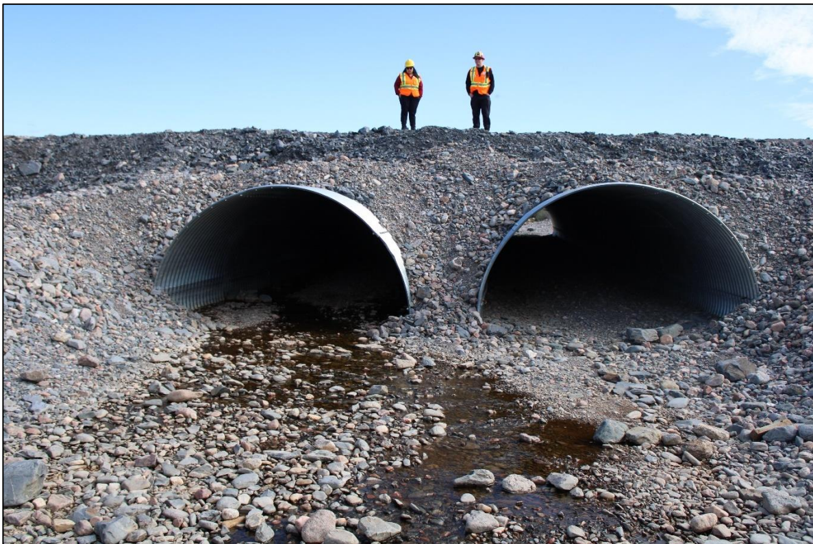
Photo 22: Culverts installed at Rascal Stream Crossing
