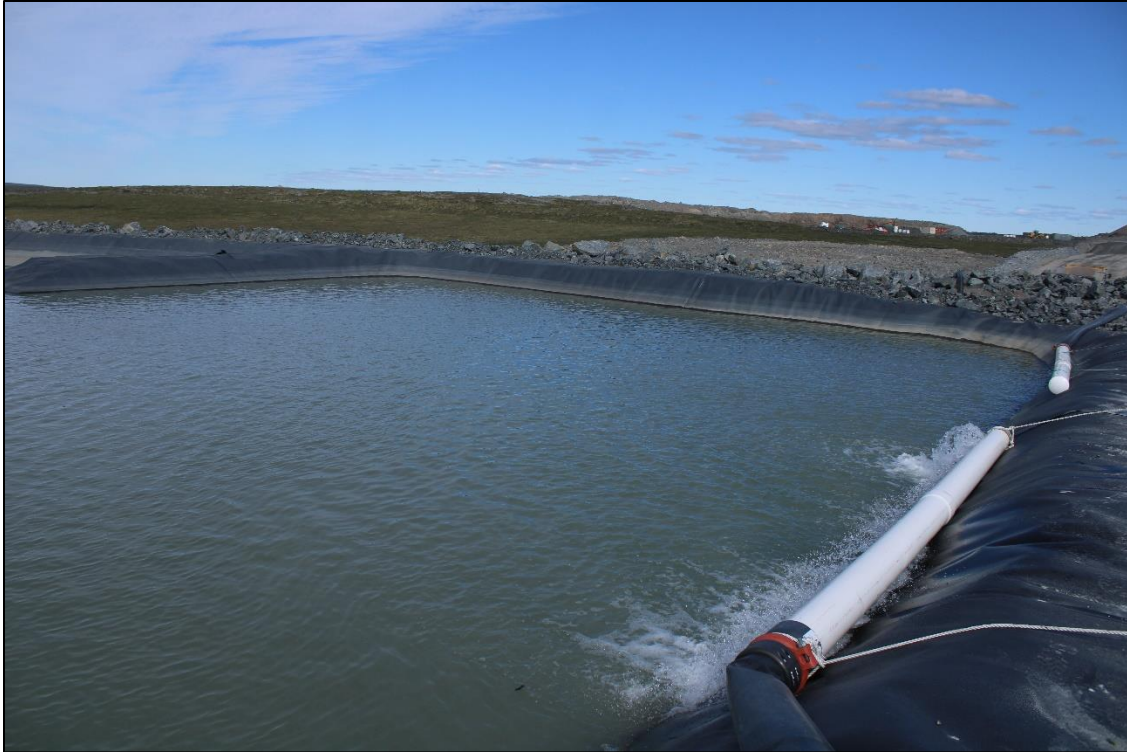
Photo 21: Lime Treatment being applied to sedimentation Ponds
