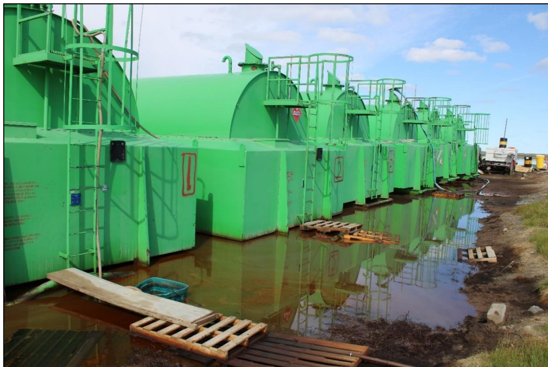
Photo 11: Contaminated Water Storage Inside the lined Bulk Fuel Storage Area
