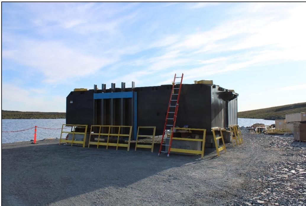
Photo 6: Lake Barge to be installed in Goose Lake for the New Water Intake Line
