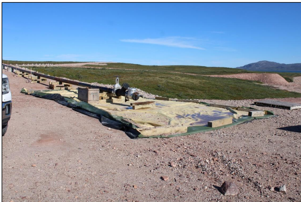
Photo 39: Fuel Barge Transfer Line prepared to Receive the 2024 Fuel Barge
