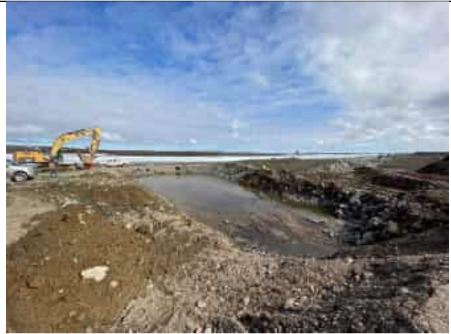
Photo 4: Twin multiplate culvert excavation at 9:53.
