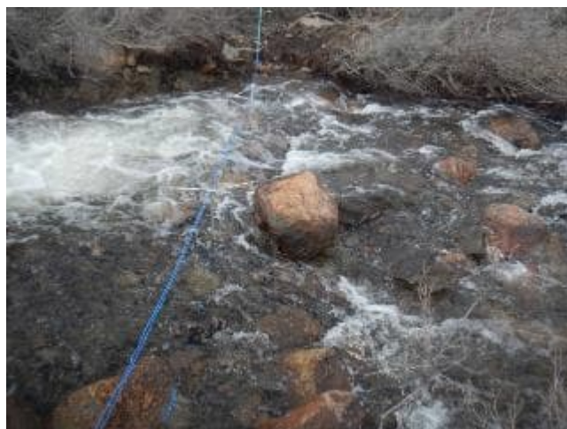
Photo B-22: Rock weir structure 4, facing left downstream bank, 5 June 2024.
