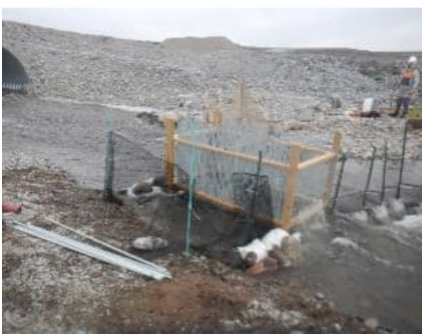
Photo B-6: Looking upstream at first fish fence trap setup from RDB.
