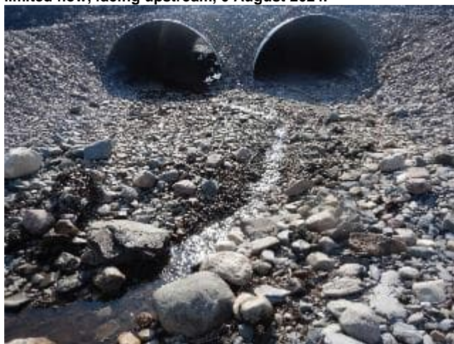
Photo B-41: Modifications made to improve fish passage, facing upstream, 8 August 2024.
