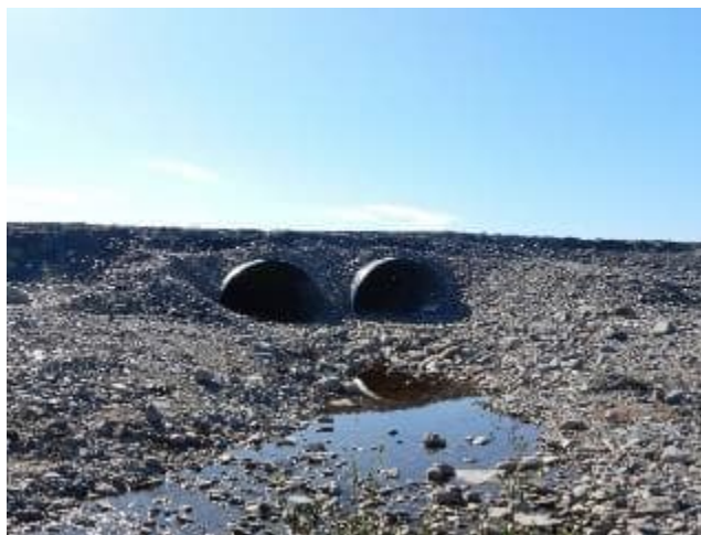
Photo B-39: Potential barrier from culverts downstream due to limited flow, facing upstream, 6 August 2024.
