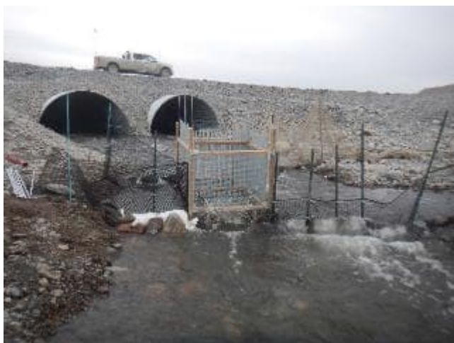
Photo B-7: Looking upstream at first fish fence trap setup from mid-channel.
