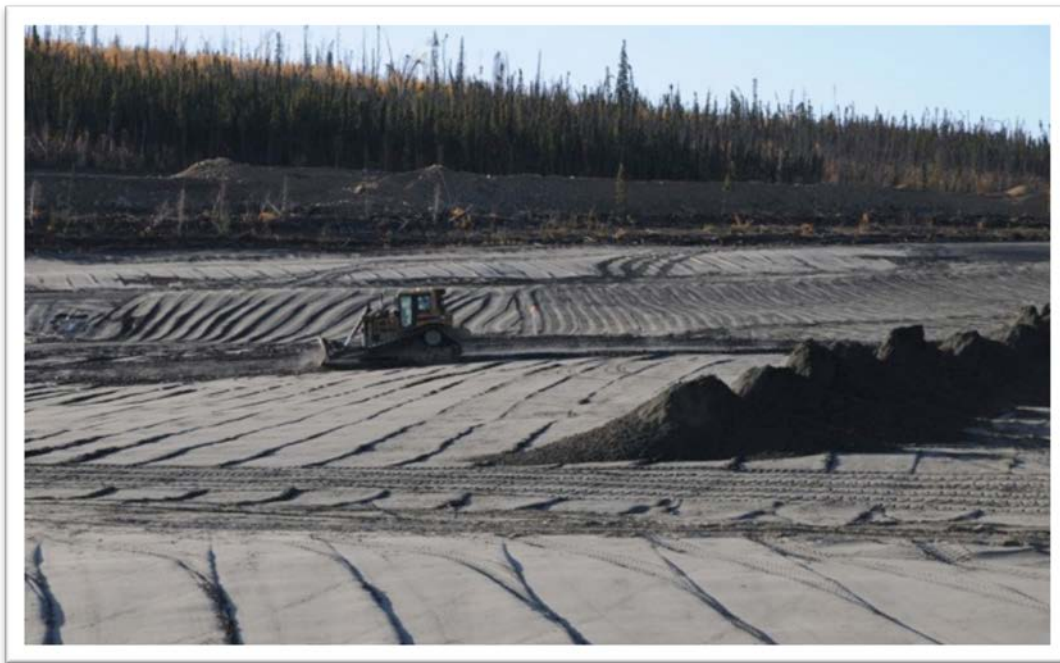
Figure 2.4-14 Tailings Dry Stack
