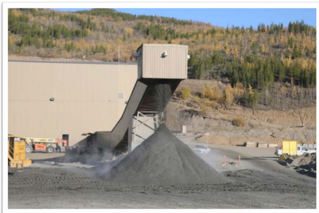
Figure 2.4-13 Typical Dry Tailings Stockpile at Process Plant
