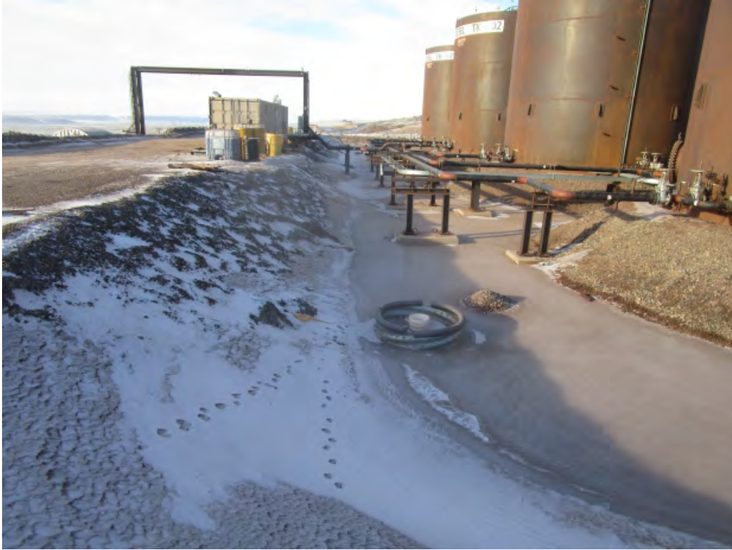
15. Mine Site Steel Fuel Tank Farm Containment.
