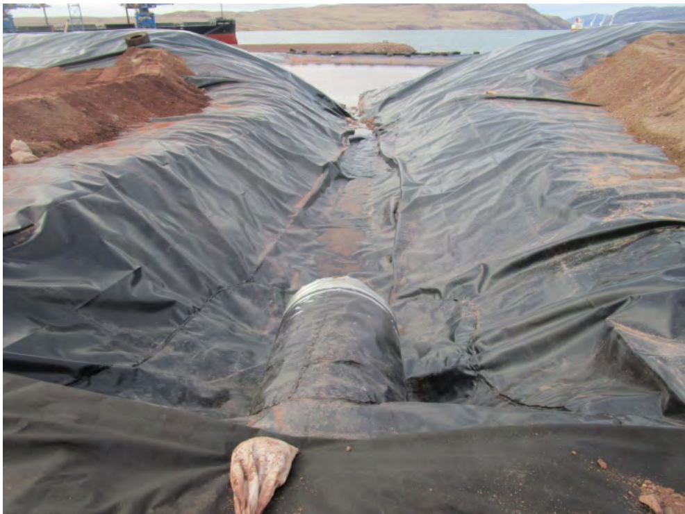
28. Sedimentation Pond East - Liner at south inlet
