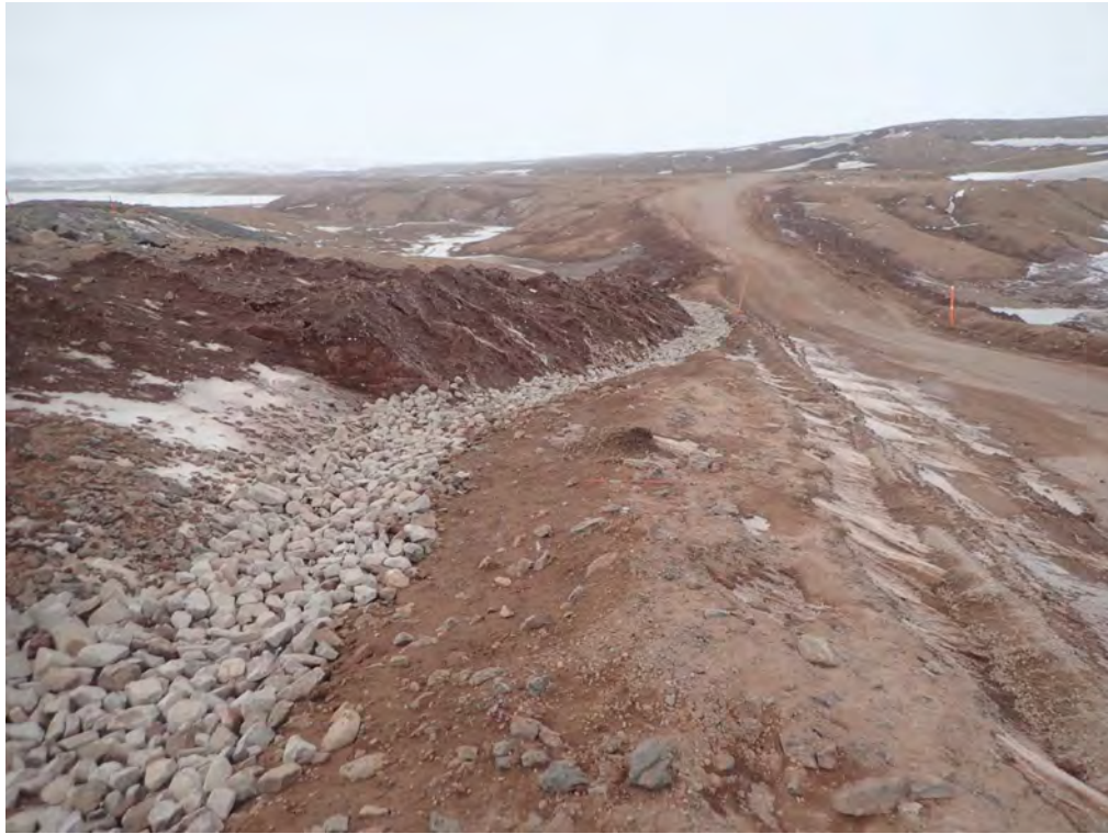
Photo 3. BG-01 Downstream Ditch Riprap Armouring (May 13, 2021)
