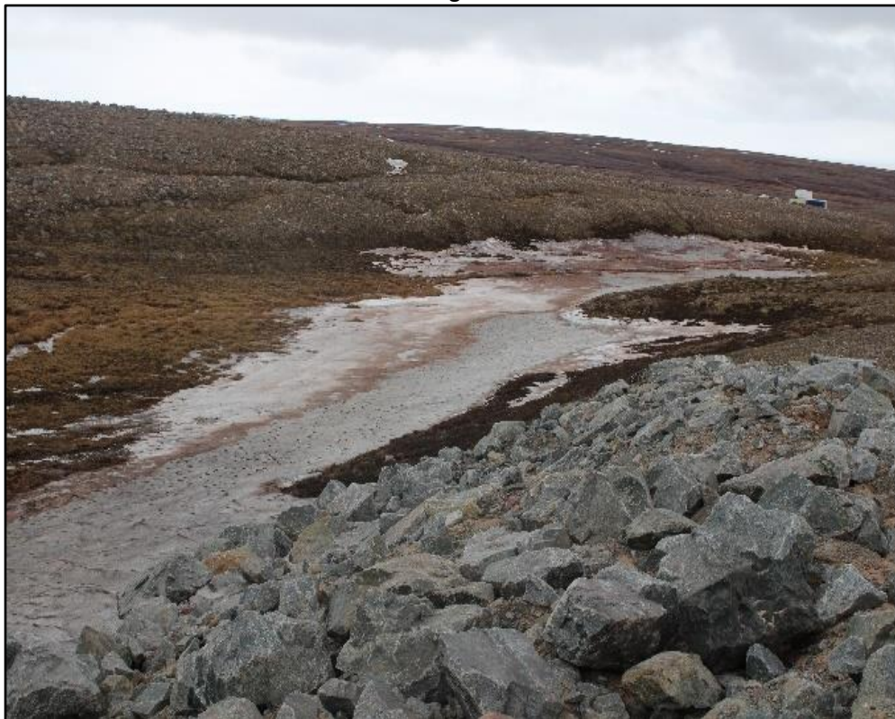
Photo 26: Slope and Ripraps of Sewage Outfall Area Embankment.
