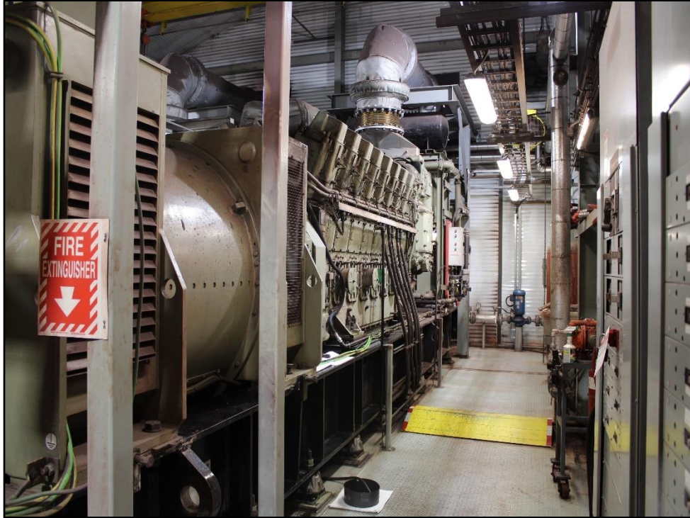
Photo 28: Indoor Diesel Generators Installed at Mary River Mine Site.
