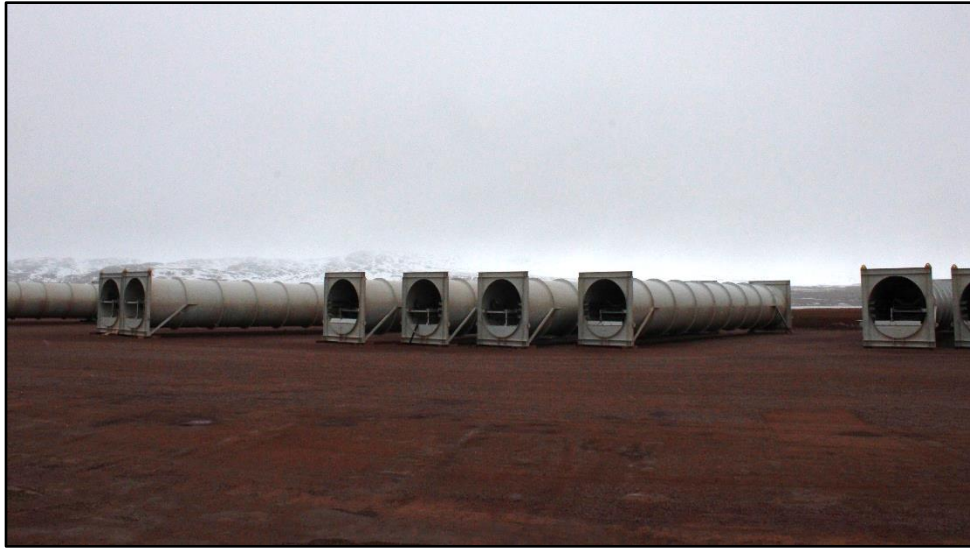
Photo 52: Phase 2 Development Enclosed Conveyor System.
