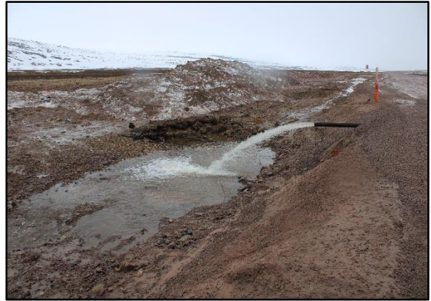
Photo 37: Temporary Water Pumping to Continue Flow.
