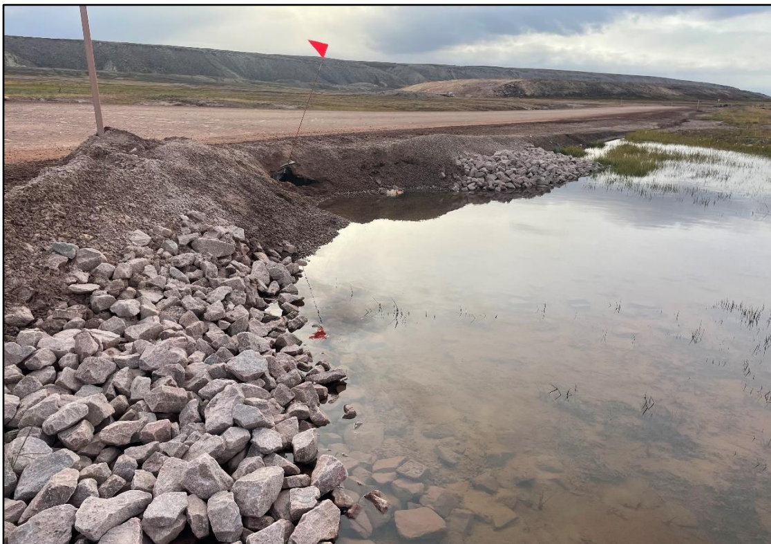
Photo 21: Rip Rap Along the Tote Road Near the Mine Site
