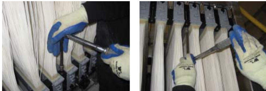
Figure 5.29 - Tightening Expanders
