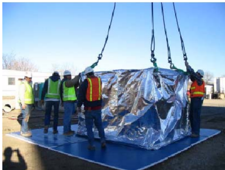
Figure 5.7 - Lifting a Cassette Without a Four-Point Lift Frame and Spreader Bar
