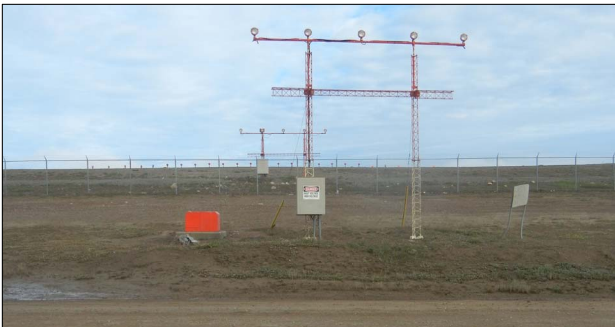
Photo C-5: Current Non-Standard Approach Lighting, towards Runway
