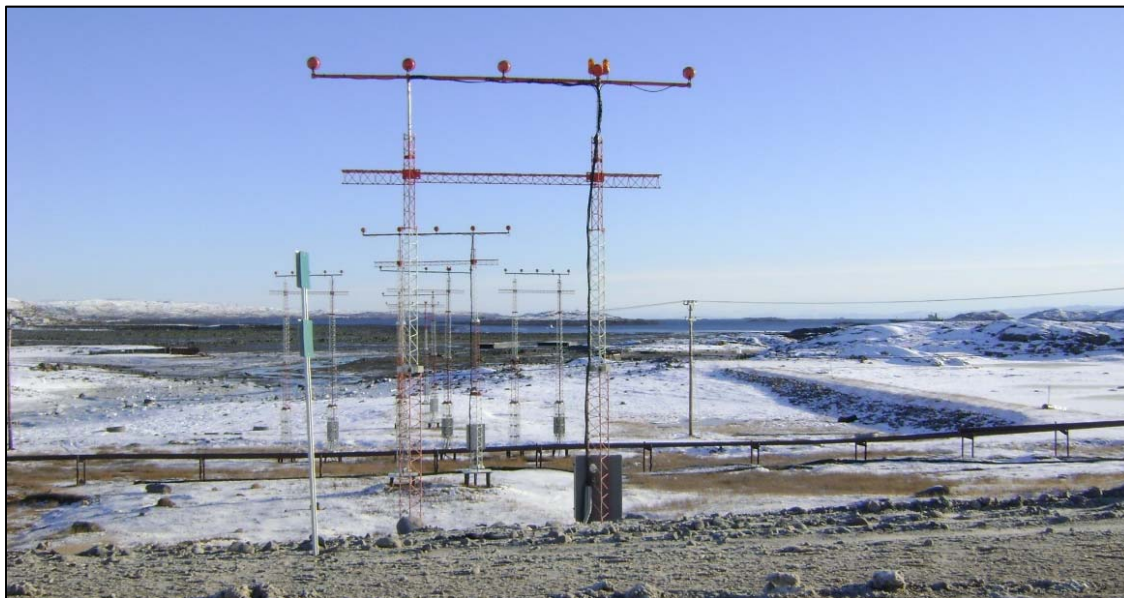
Photo C-3: Current Non-Standard Approach Lighting, towards Frobisher Bay
