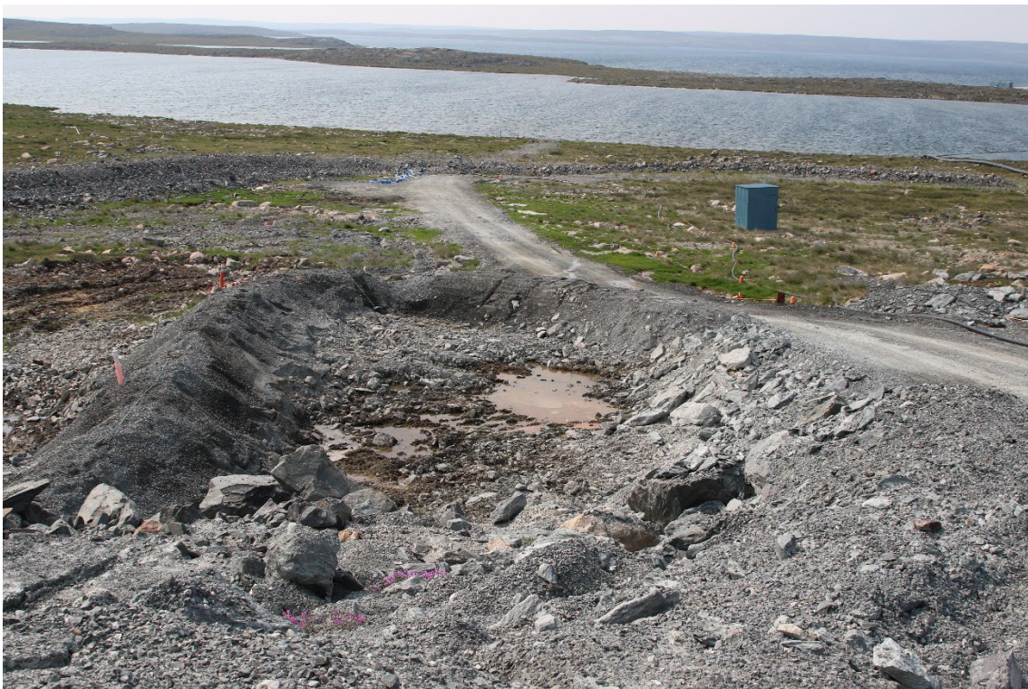
Photo 40: Silt discharge area downslope from Mill, work ongoing.
