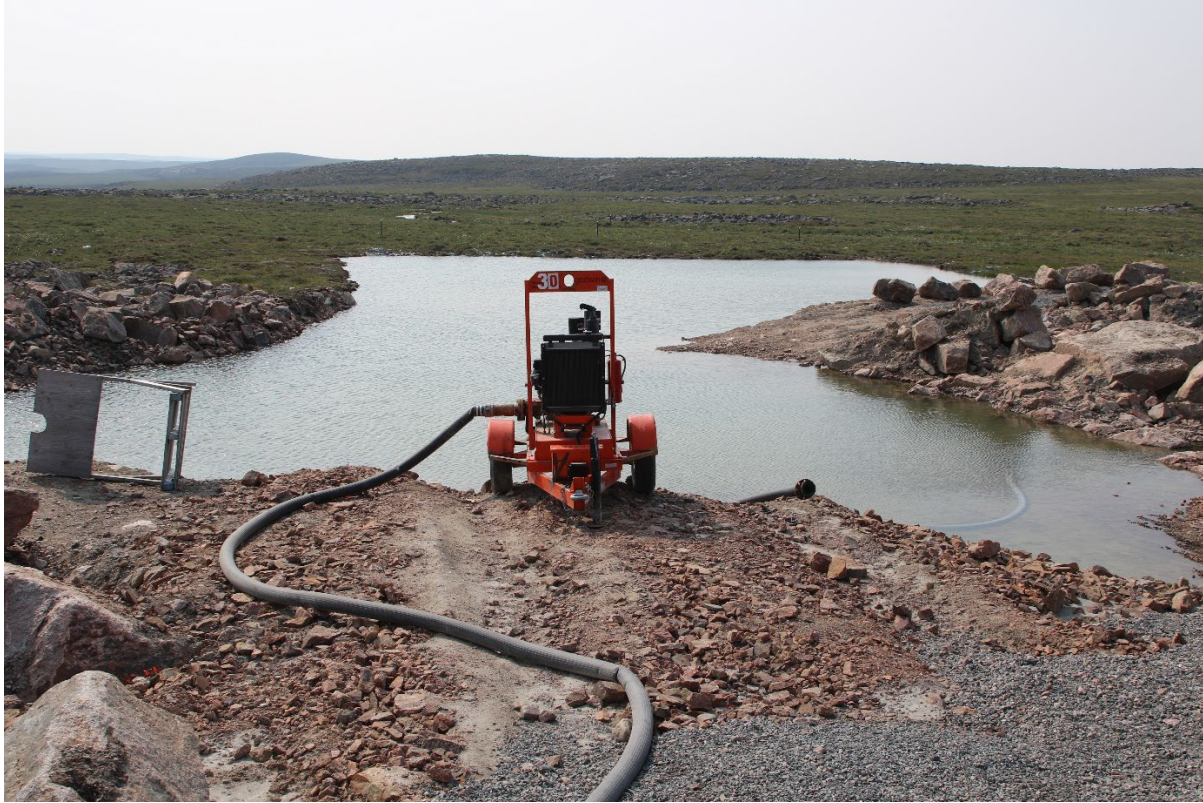
Photo 14: Water pump removing water from a spill cleanup site at kilometer 87 of the AWAR. This was the site of spill in December 2022 and CIRNAC is working with the Proponent on clean-up.
