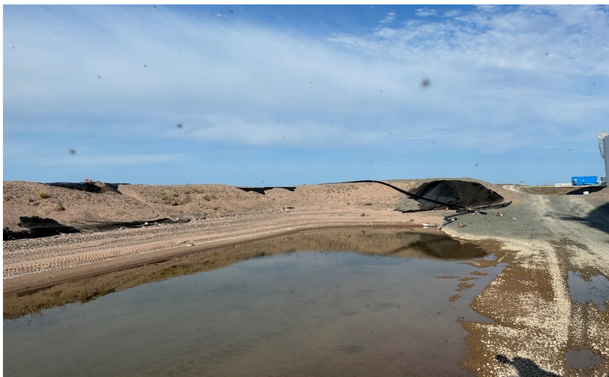
Photo 7: Exposed liner at the Baker Lake Marshalling Facility. Pooled water is pumped out and stored in the Stormwater Management Pond at the Meadowbank Site (2023). Repairs to take place in 2024.
