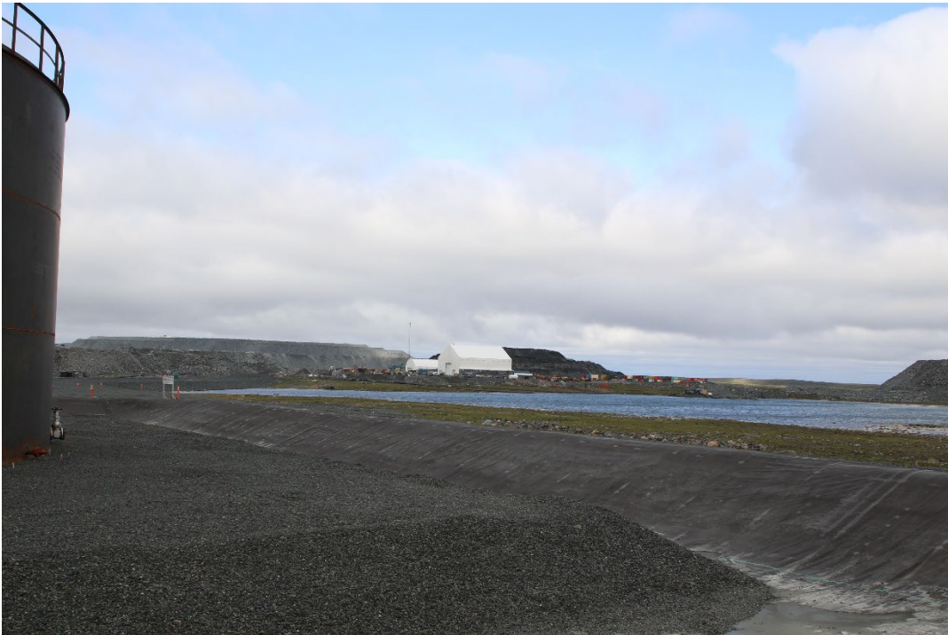
Photo 46: Whale Tail Site tankfarm. A large area of exposed liner is seen in the secondary containment berm.
