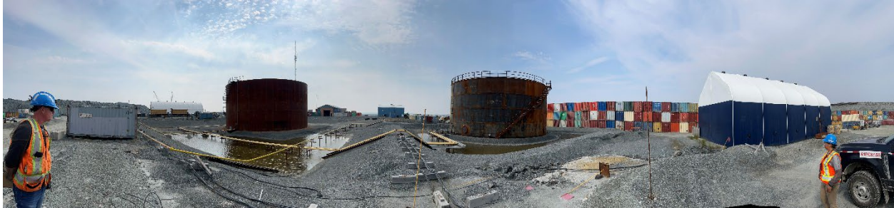
Photo 37: New fuel tank constructed in 2023. The purpose of this tank is to increase onsite fuel storage capacity to reduce reliance on trucking fuel from Baker Lake during caribou migration road closures.
