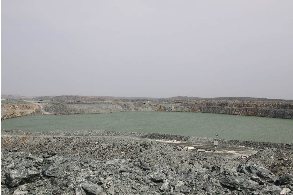
Photo 29: Goose Pit. This pit previously received tailings deposition and is now capped with 35-40 metres of water.
