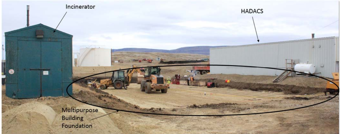
Figure 2.2. Existing Incinerator, HADACS Building and New Multipurpose Building Foundation, August 2015
