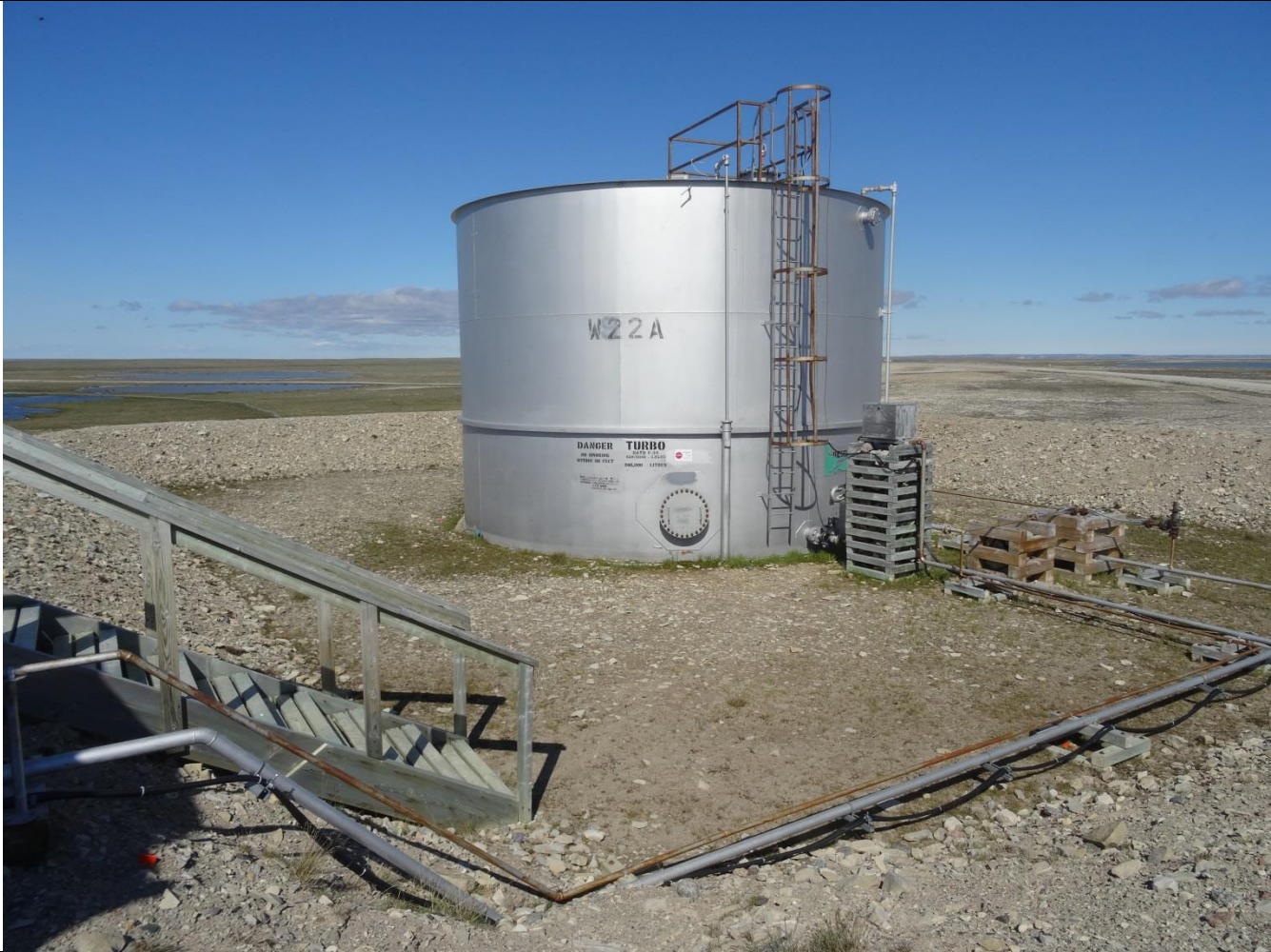
Description: Tank W22A – at NWS Site Area - Well Marked – Berm in Good Condition, Clean and Dry inside
