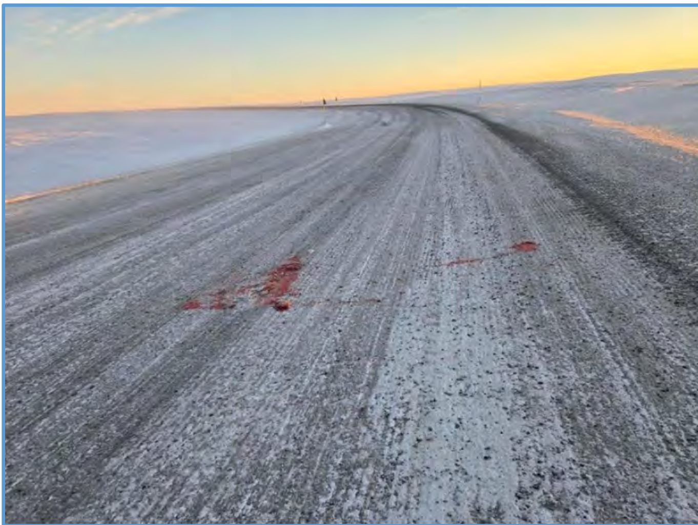
Figure 2: WTHR km 112 (looking SE)
