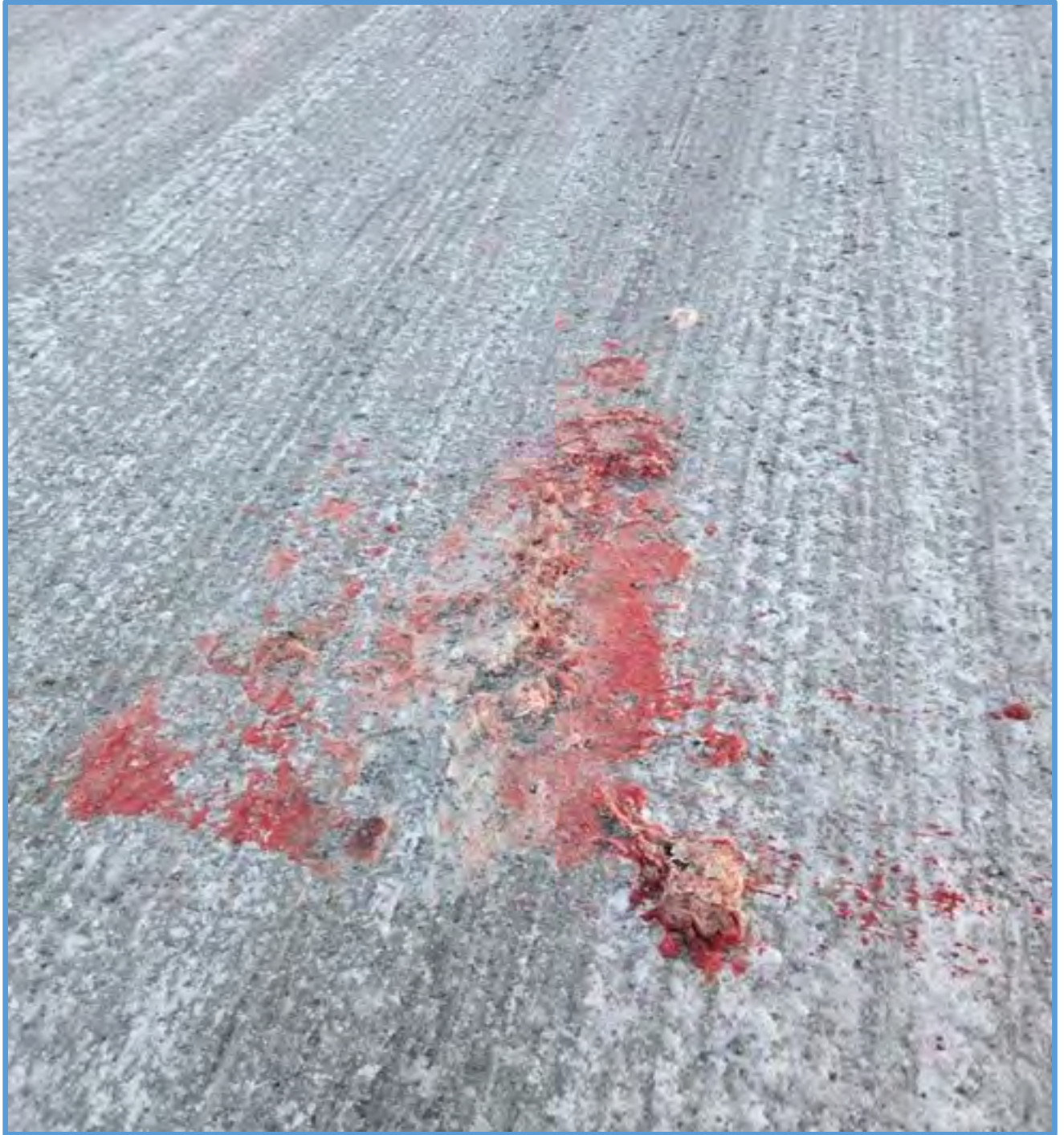
Figure 1:WTHR km 112 (looking SE)
