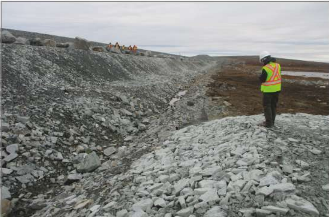
Photo 12: Dike D-CP1 - ground between the dike toe and water collection channel covered with rockfill toe berm.
