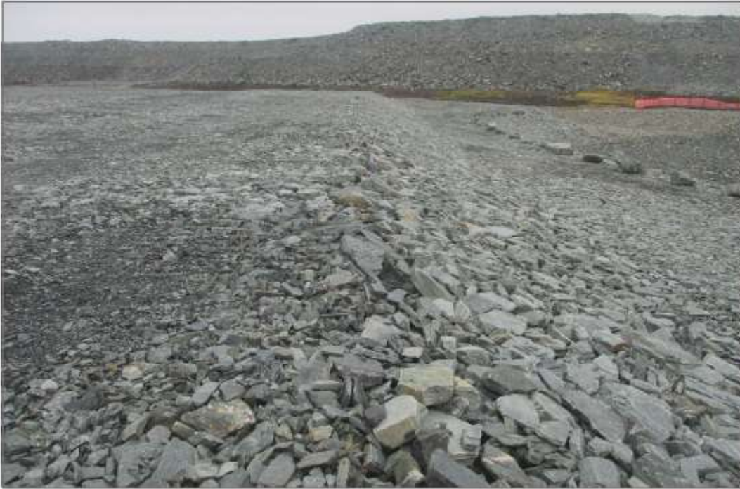
Photo 9: Pond CP4 - Rockfill placed between CP4 slope and berm to reduce thaw subsidence observed in 2021 inspection.
