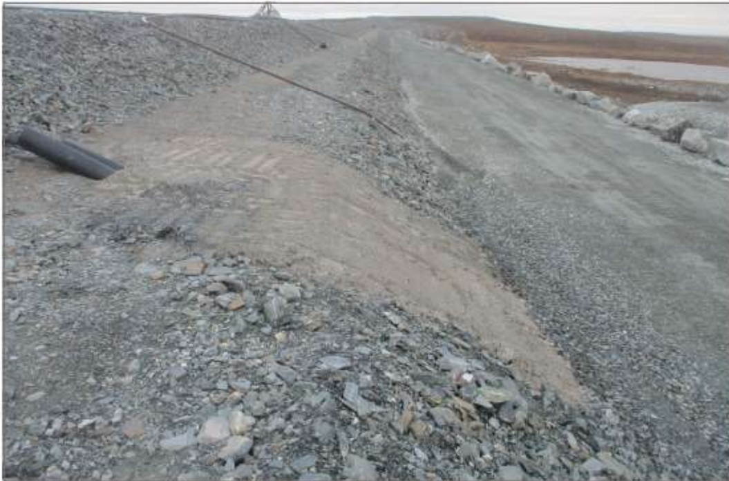
Photo 15: Dike D-CP1 - Buried line along downstream crest of dike for dewatering seepage collection pond.
