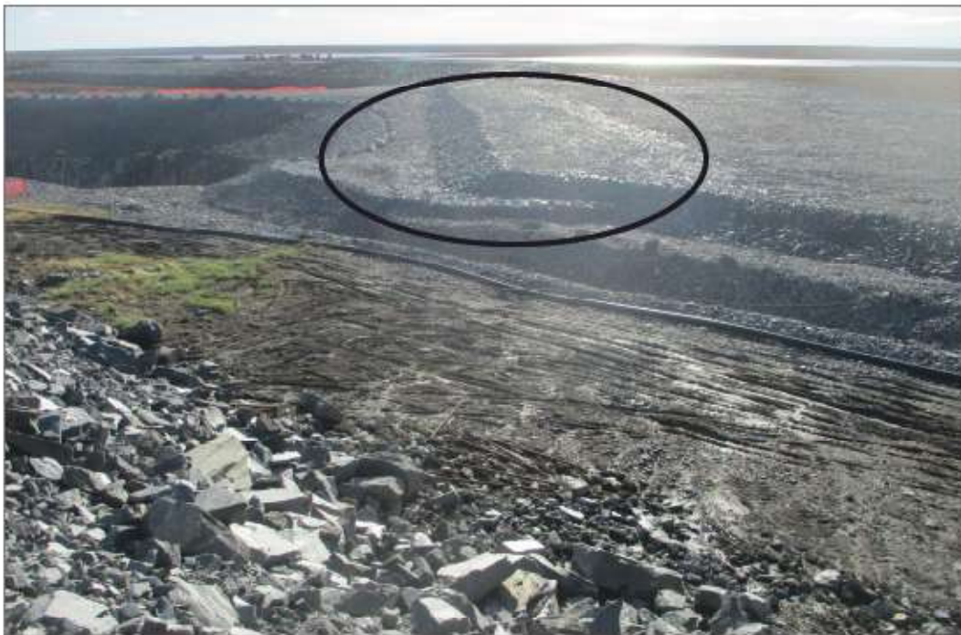
Photo 8: Pond CP4 - North slope, Rockfill placed in area between rockfill covered slope and thermal berm in 2022.
