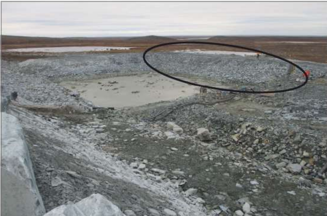
Photo 10: Dike D-CP1 - Seepage collection pond downstream of dike. Deformation of fill at southeast corner of pond has been rebuilt and rockfill cover placed on exposed tundra.
