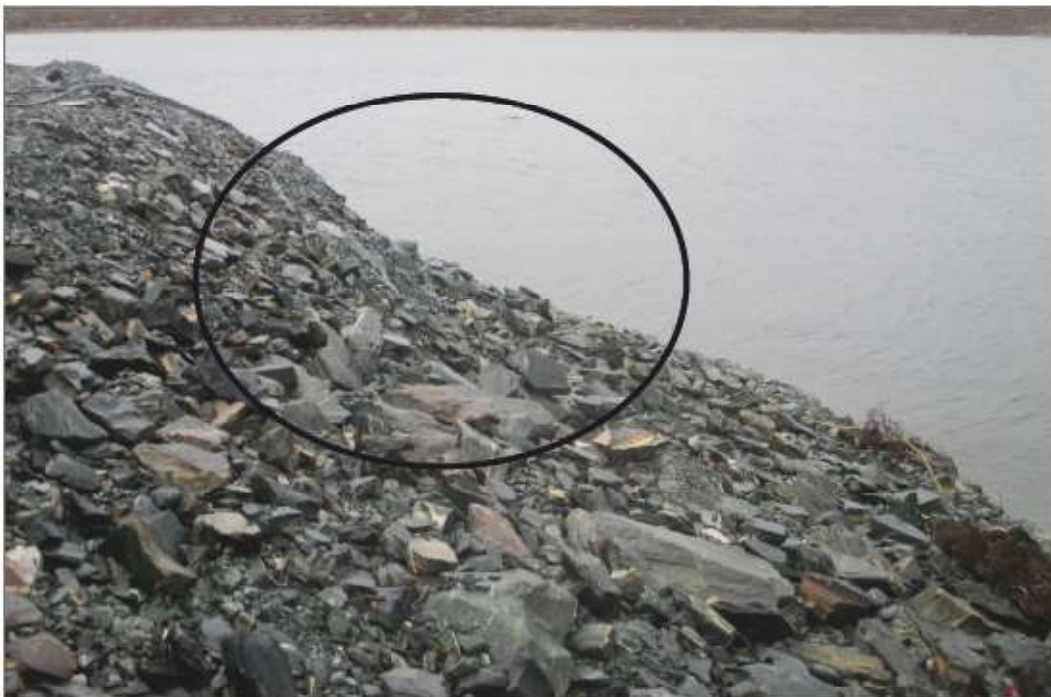
Photo 18: Dike D-CP1 Jetty 1—Erosion at southeast corner—under cutting top portion of fill. No change from previous years.
