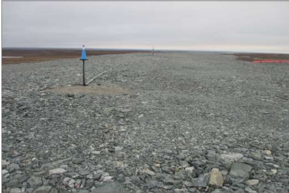
Photo 7: Pond CP6 - Berm CP6 crest. Minimal settlement.
