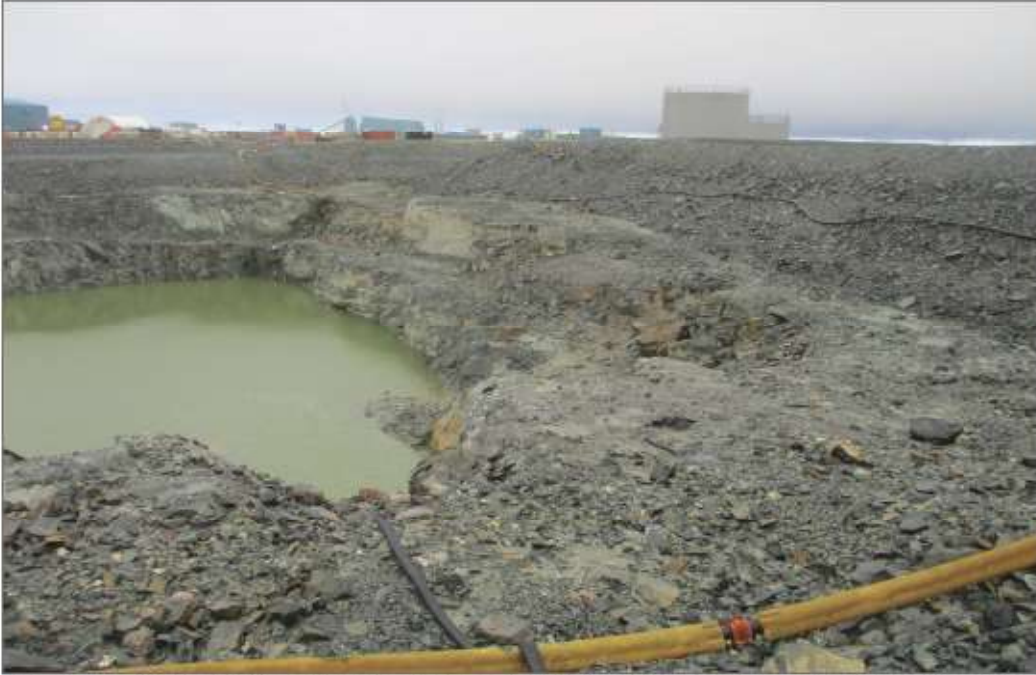
Photo 1: SP1 Saline Pond - looking towards the northwest. Pond in bedrock, ROM covered overburden slopes
