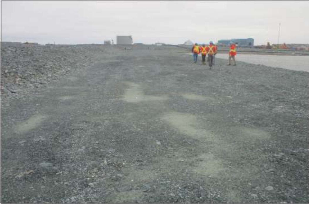
Photo 9: Dike D-CP1 - Upstream crest in good condition.
