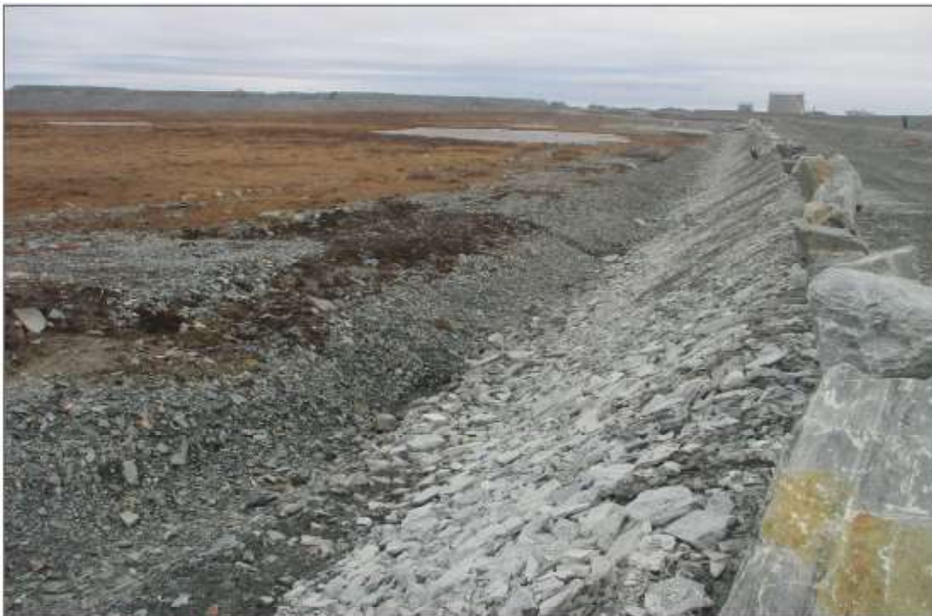
Photo 14: Dike D-CP1 - North end of disturbed ground between dike toe and seepage collection channel.
