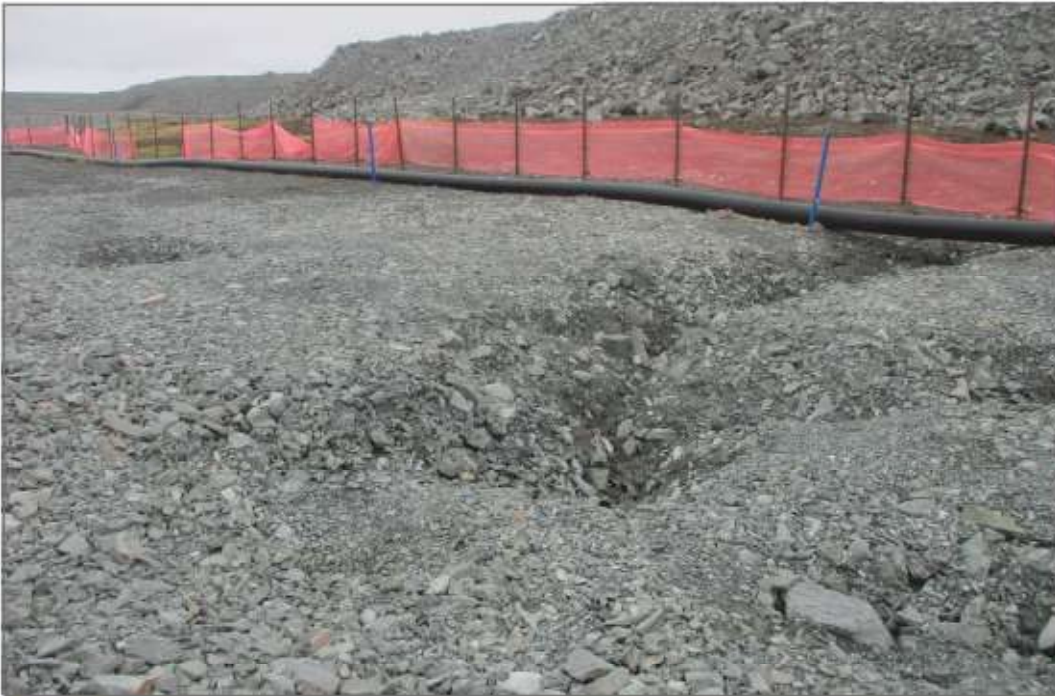
Photo 6: Pond CP4 - Northeast slope, settlement in area between rockfill covered slope on original ground.
