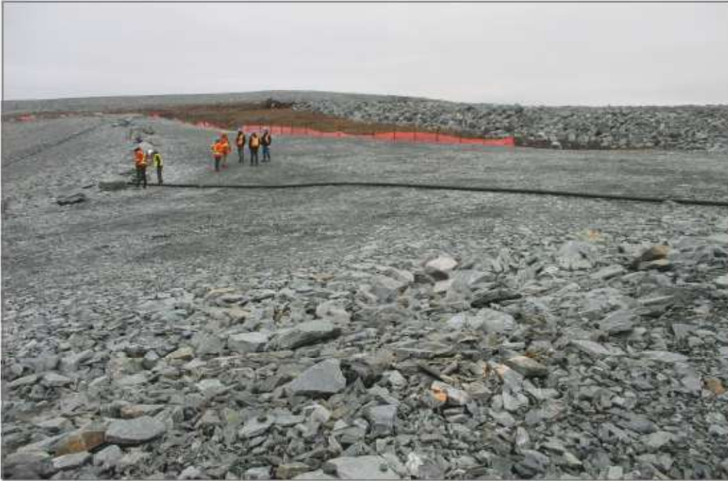
Photo 13: Pond CP4 - Rockfill cover placed over native ground above slopes of CP4.
