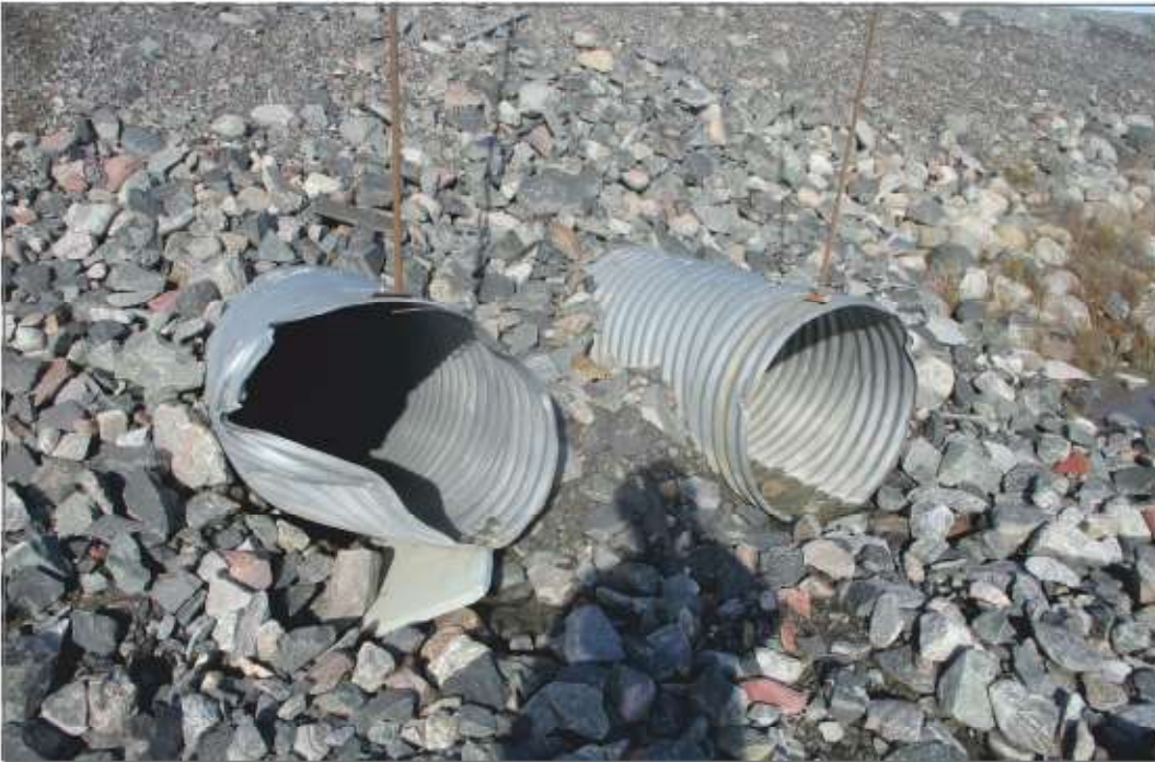
Photo 8: Culvert C13—Damage to culvert,
