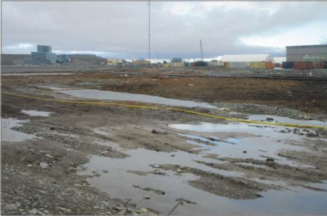
Photo 31: Channel 5—Upper reach, south of Portal2, significant subsidence and cracking along slopes with rip rap settled below water level in channel.
