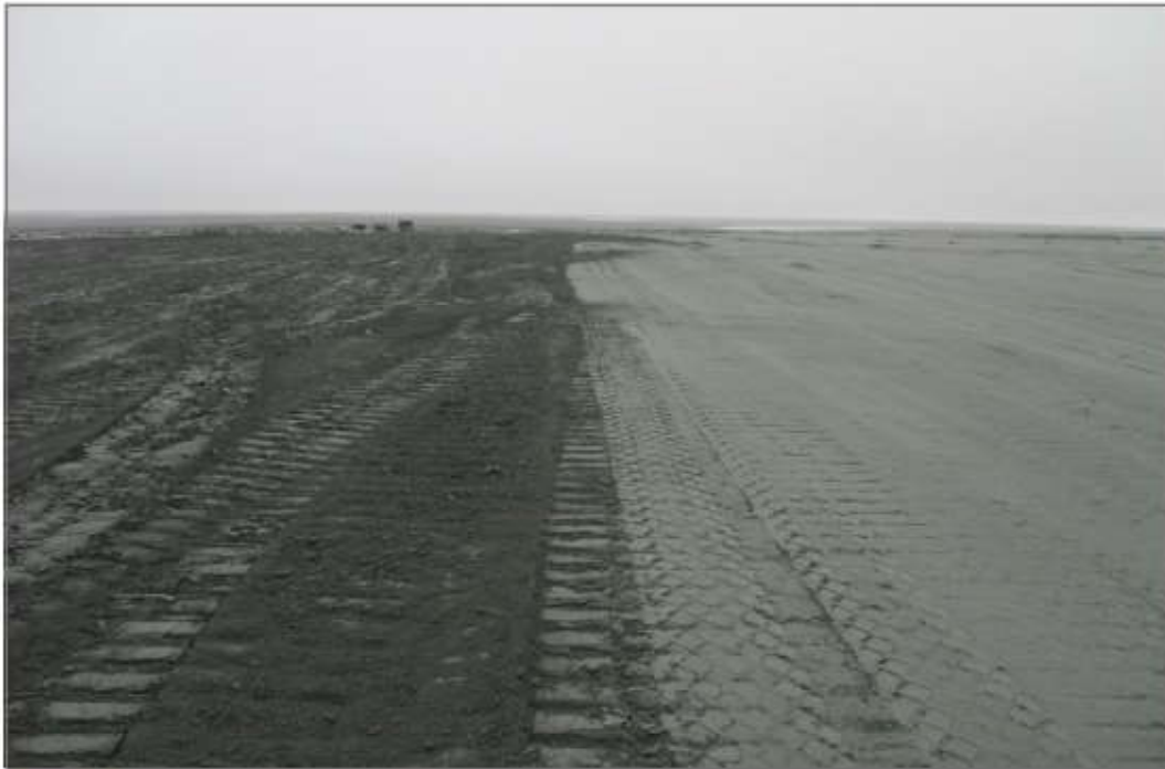
Photo 6: TSF - Compacting tailings.
