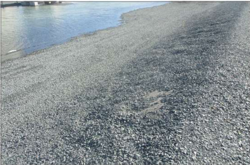
Photo 18: ITIVIA Tankfarm—Exposed geotextile on south berm embankment.
