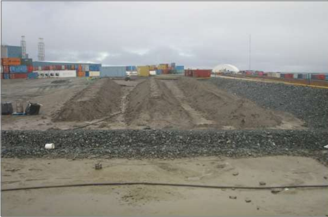
Photo 19: Landfarm— Windrows of contaminated soil.
