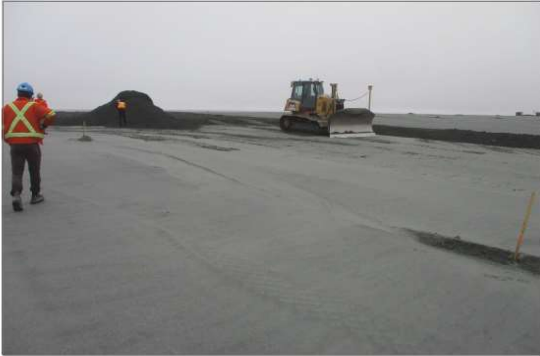
Photo 5: TSF - Spreading tailings.
