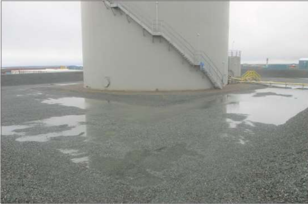
Photo 25: Industrial Fuel Storage Tanks.—Ponded water in tankfarm.
