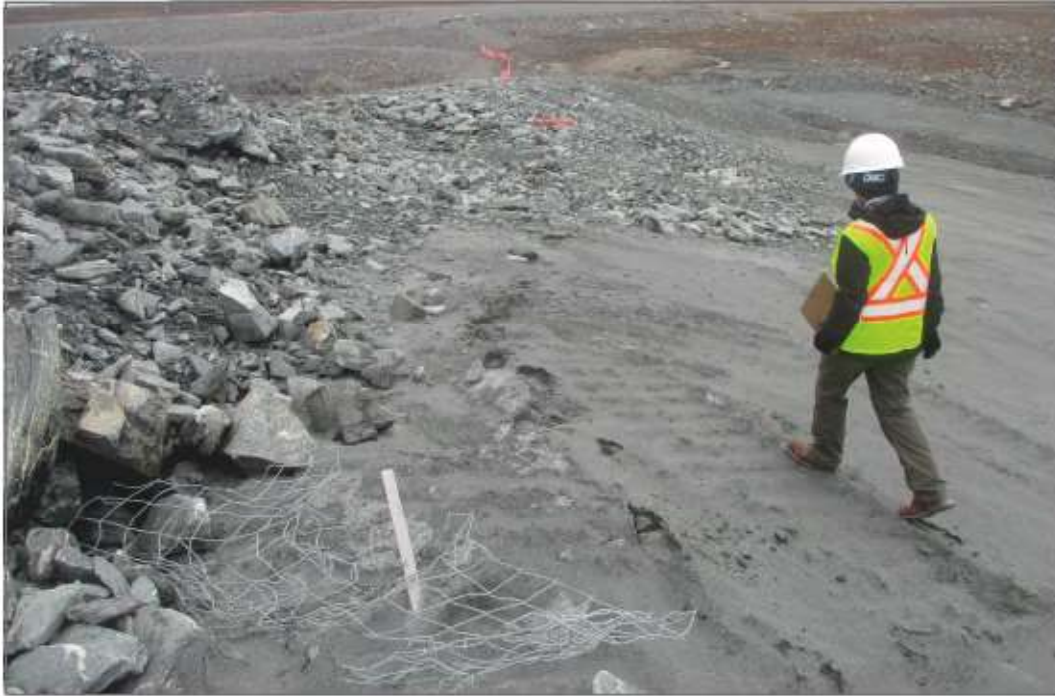
Photo 9: TSF - contact between rockfill cover and tailings at the northwest corner of Cell 1.
