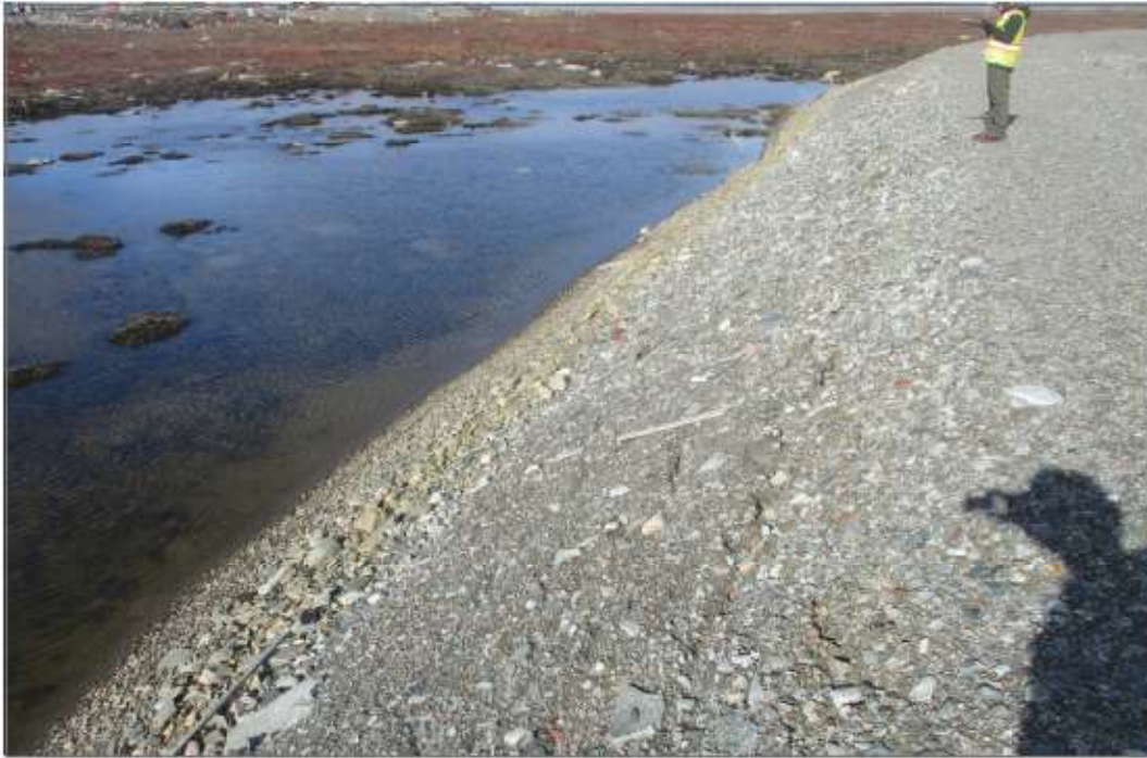
Photo 49: Berm 2—Impounded water against upstream side of Berm 2 with high water mark.
