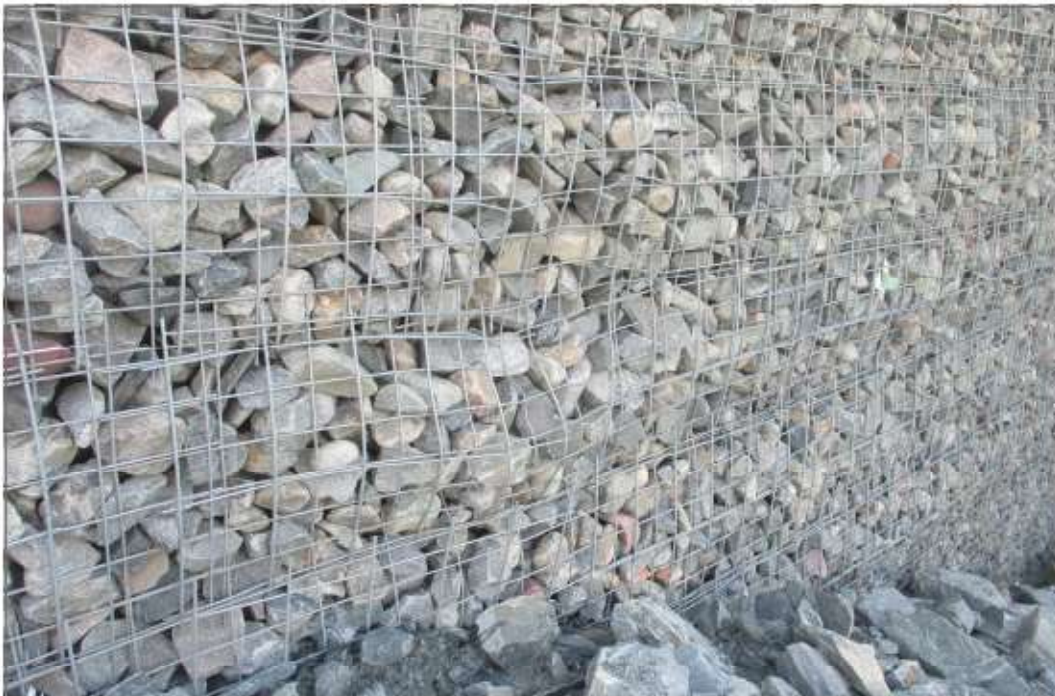
Photo 8: Crusher Pad—MSE wall, north east side. Slight localized bulge and distortion of gabion cage.
