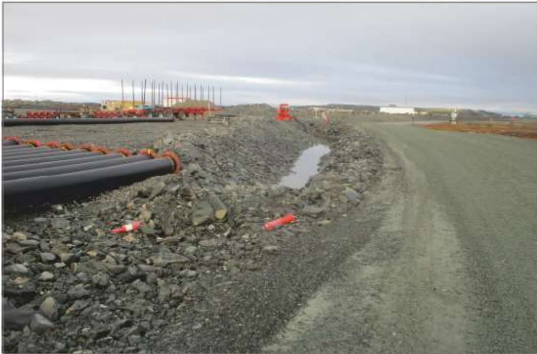
Photo 34: Culvert km 29.6 replaced with sump and pump to water storage in pit
