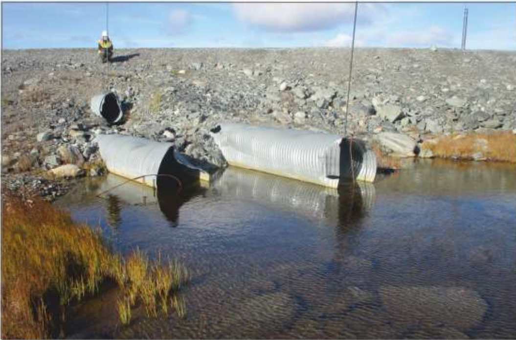
Photo 8: Culvert km 7.4—Damage to culvert inlets
