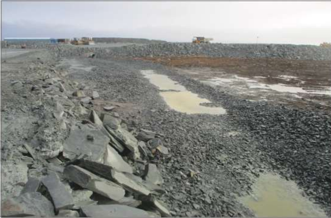
Photo 35: Channel 7—Upper reach, minor subsidence and pooling at bottom of channel, looking north.
