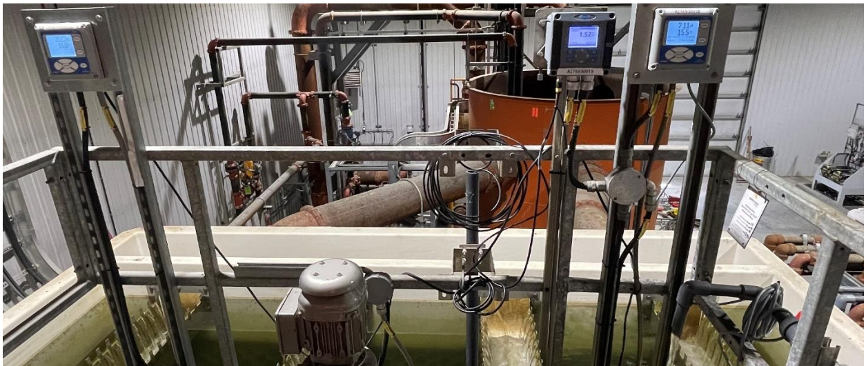
Photo 24: Water treatment complex - contact water is treated to ensure licence parameters are met before discharge into Meliadine Lake.
