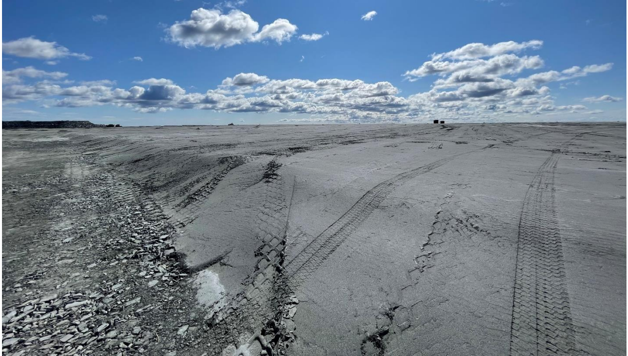
Photo 29: Dry stack tailings storage facility. Agnico Eagle noted that new light sensors are being used to monitor dust from the tailings as well as the use of drones.
