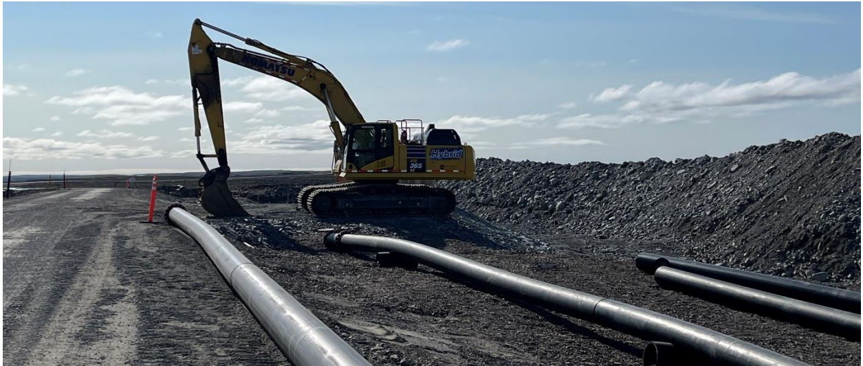
Photo 13: Agnico Eagle constructing the bedding for the waterlines beside the All-weather Access Road.
