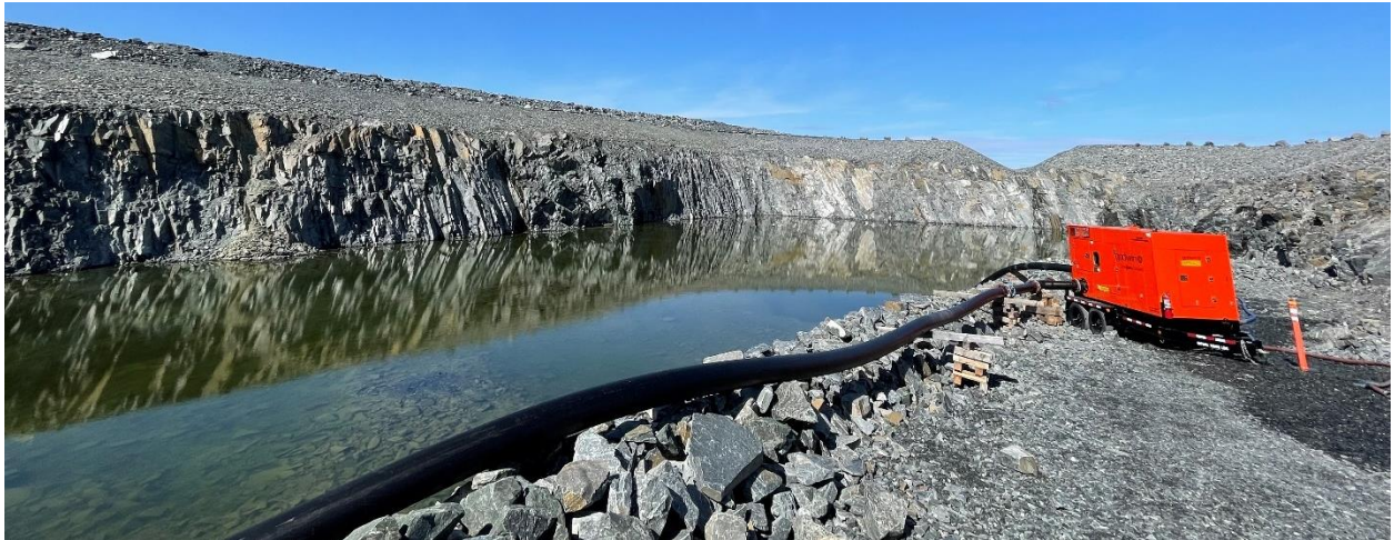
Photo 23: Containment pond 2 – Six (6) containment ponds on site collect site contact water.
