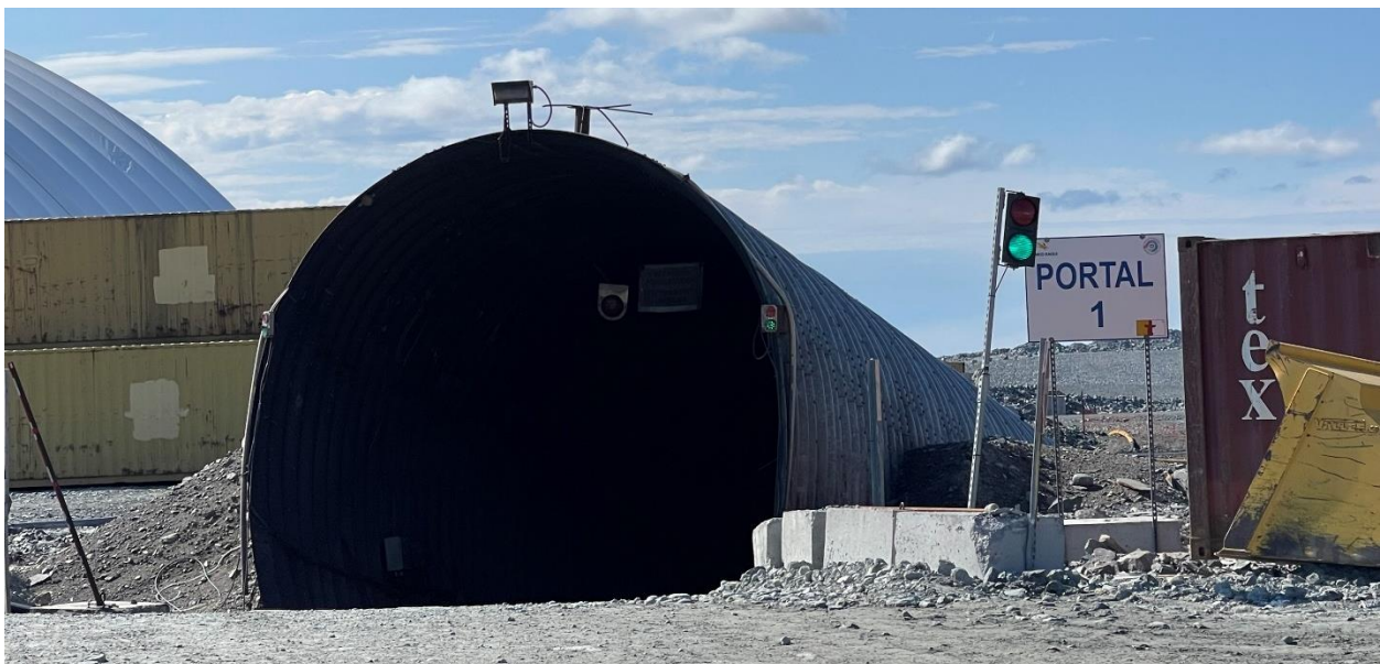
Photo 18: Portal for Tiriganiaq Underground. Actively being mined while the NIRB staff were at site.
