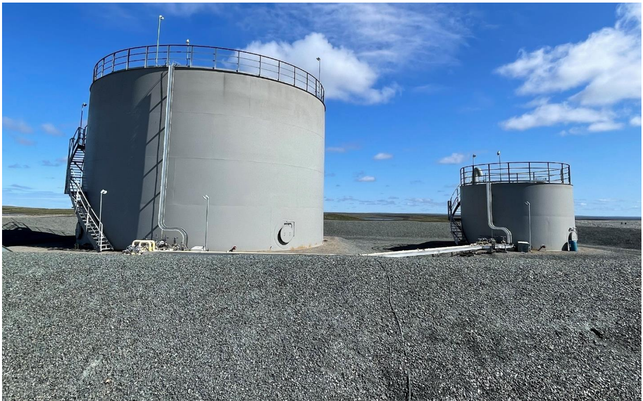
Photo 32: On-site fuel storage in secondary containment. Bird deterrents were removed for caribou migration.
