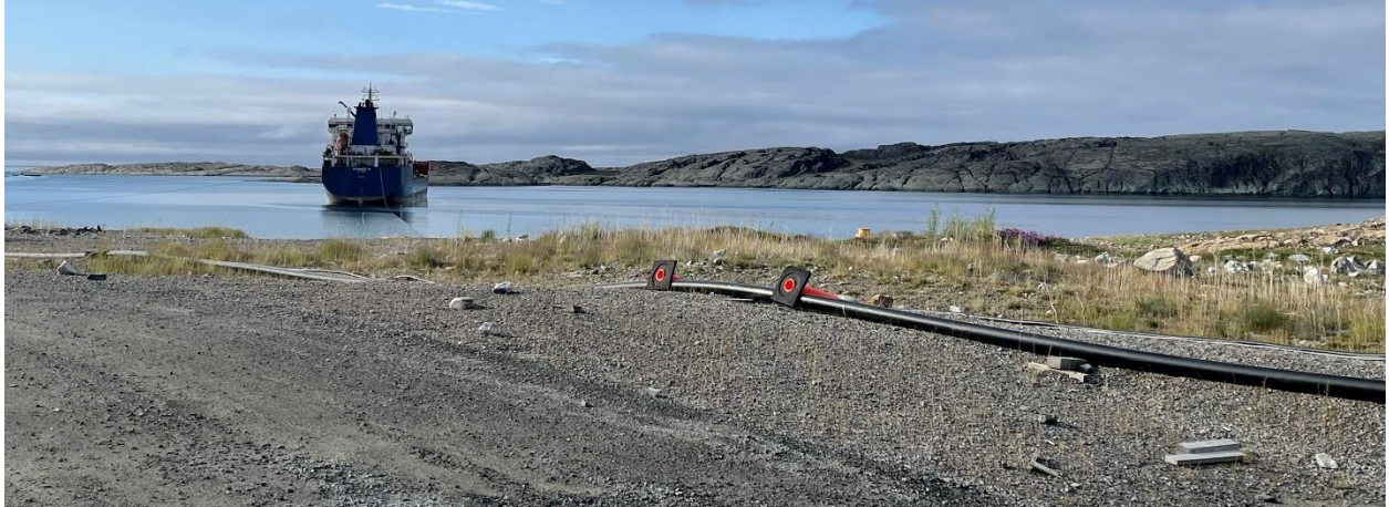
Photo 6: Saline effluent discharge pipeline to the ocean diffuser in Melvin Bay, the seasonal connection to the saline effluent diffuser was not installed in 2023.
