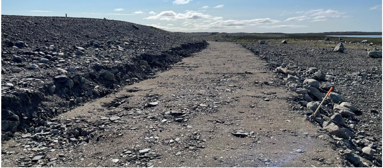
Photo 13: Agnico Eagle constructing the bedding for the waterlines beside the All-weather Access Road.
