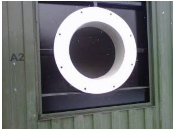
Correctly Installed Gasket
