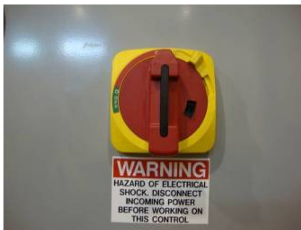
Power is ON in this position
