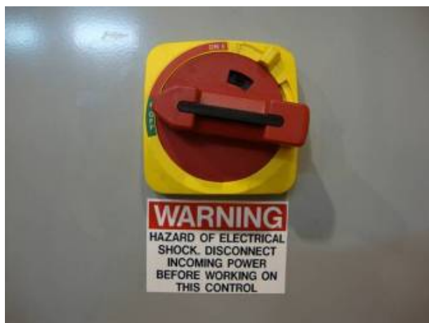
Power is OFF in this position
