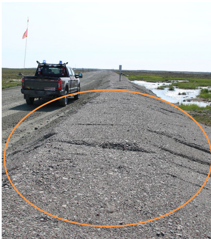
Photo 22: Raised waterline profile, waterline on south side of AWAR with rills/natural settling looking east.
