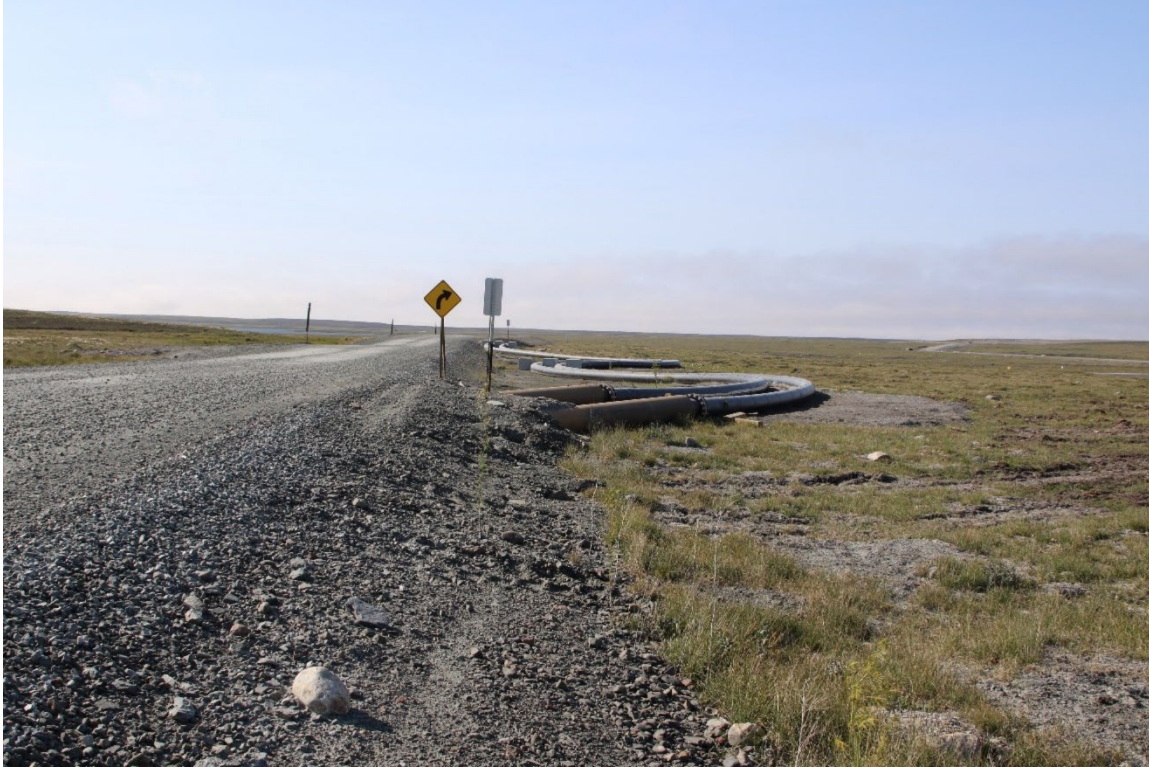
Photo 13: Uncovered waterline crossing on the south side of AWAR same location as previous photo and waterline crosses under AWAR several times.
