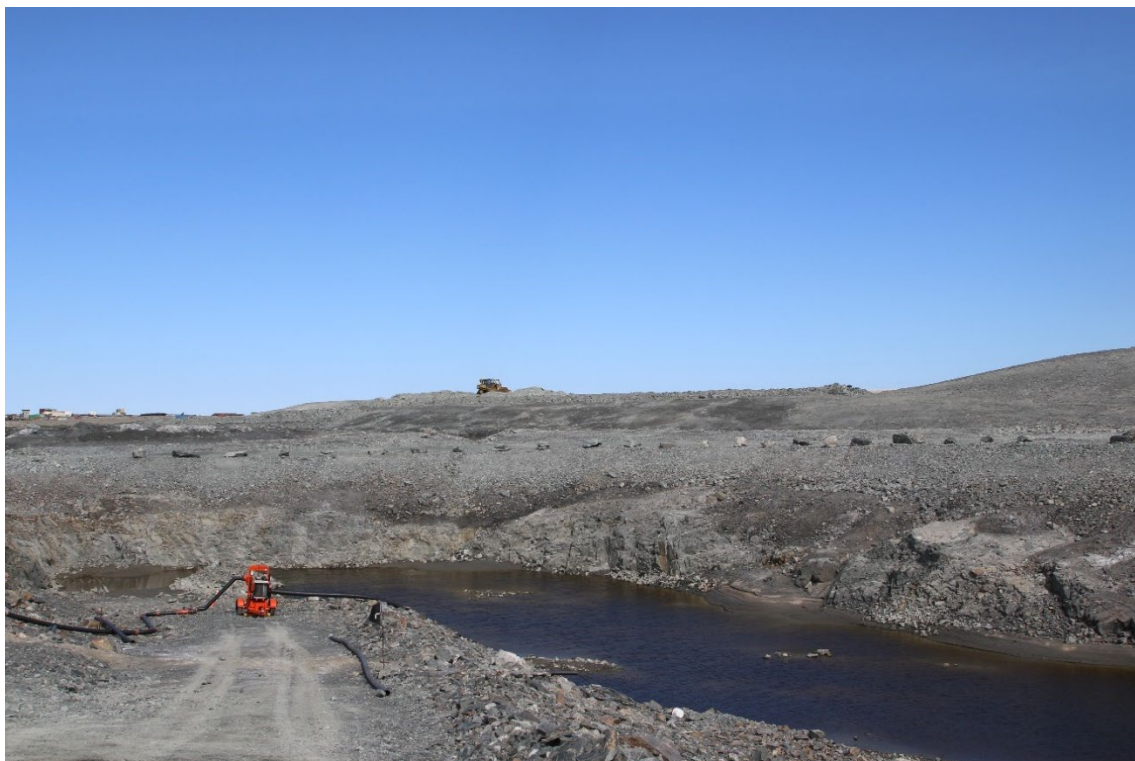
Photo 37: Containment Pond 3 – one of six (6) containment ponds to collect site contact water.
