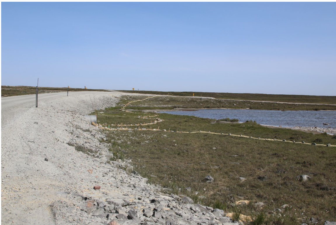
Photo 26: Erosion mitigation north side of AWAR Culvert 14 looking west.
