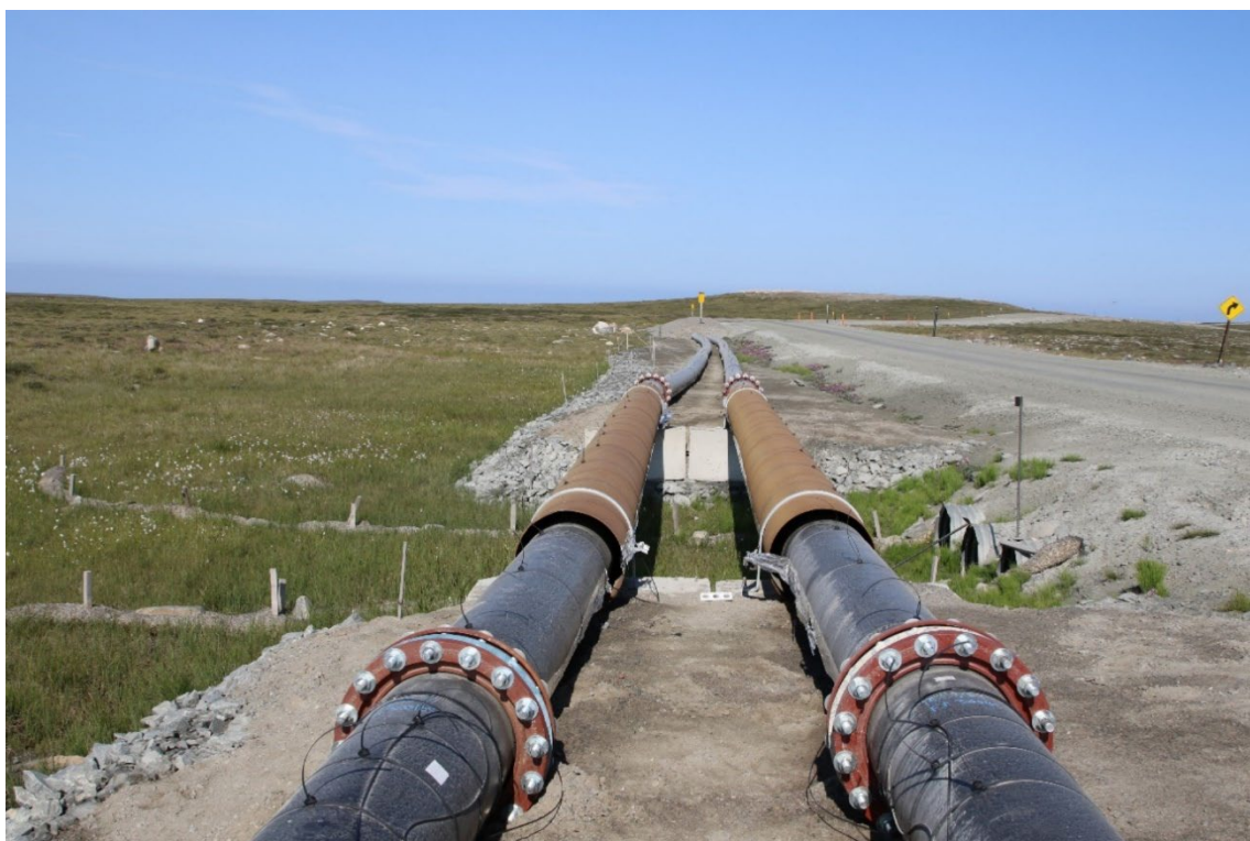
Photo 16: Suspended waterline to maintain waterflow in the area north side of road, view looking west.
