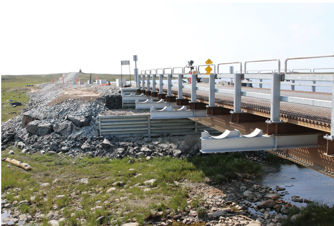
Photo 27: Example of bridge preparation for waterlines installation, south side looking west.
