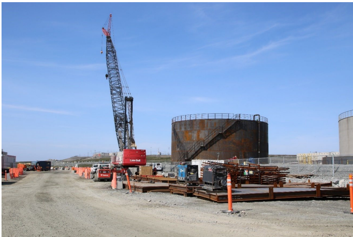
Photo 4: Construction of new fuel tank at Itivia Harbour.
