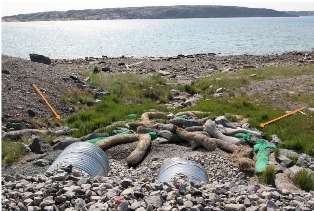
Photo 2: Sediment management at Laydown Area to Itivia Harbour.
