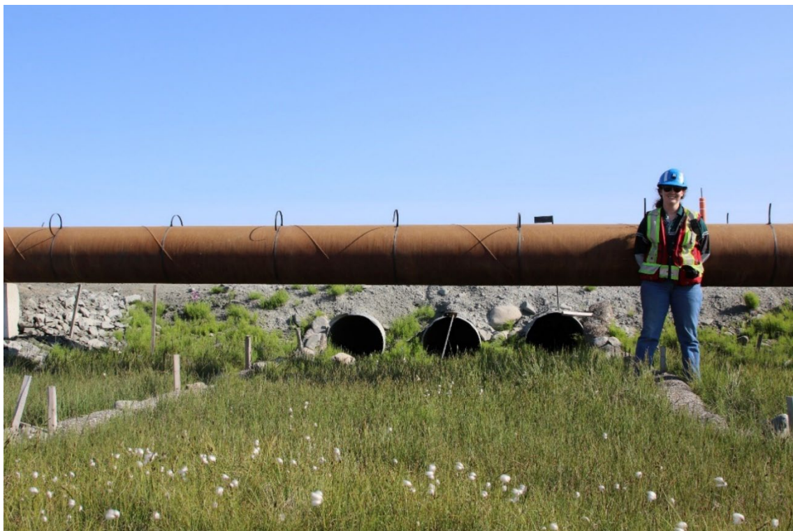
Photo 17: Suspended waterline to maintain waterflow in the area on south side of AWAR, same location as previous photo.
