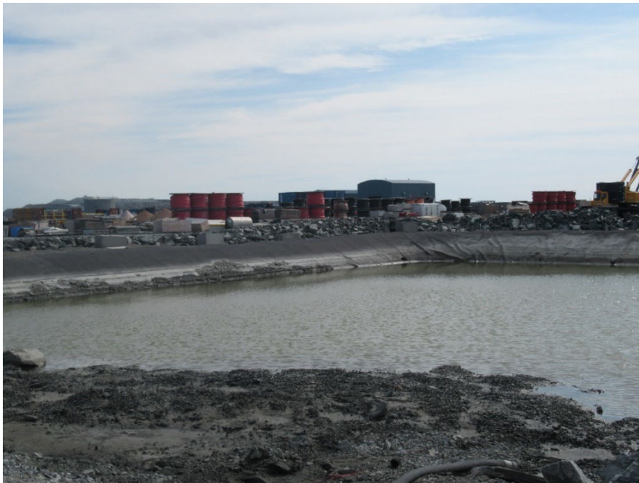
Photo 36: Saline Pond 3 – not used for saline effluent discharge in 2024; however, it is used for site contact water transferred to CP1 for treatment before release.
