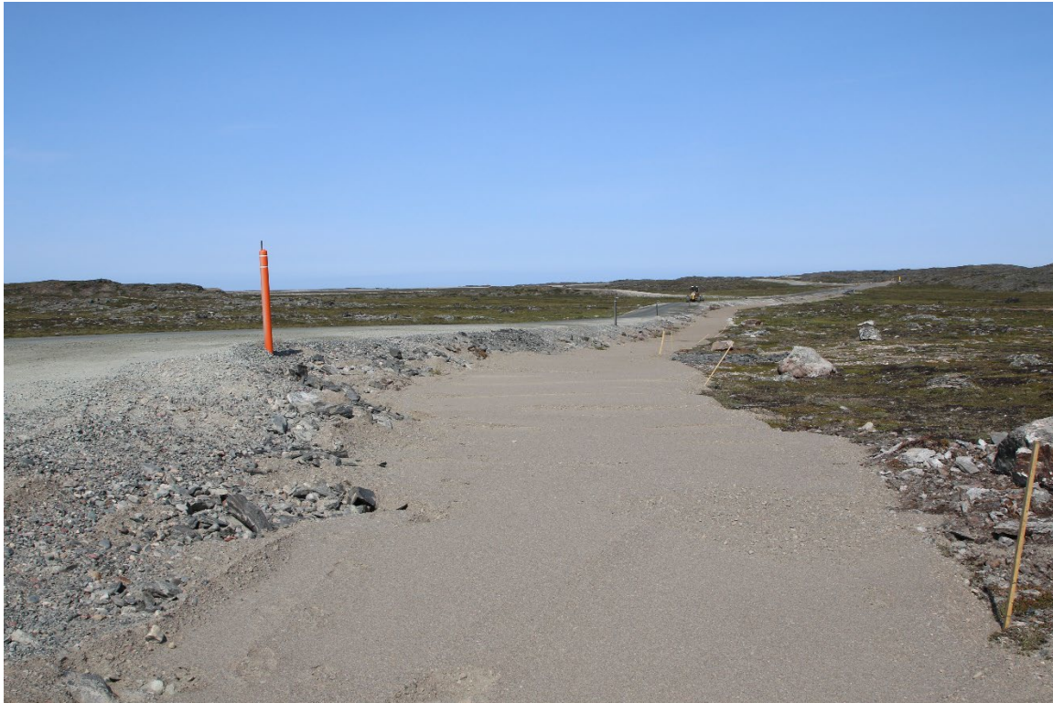
Photo 23: Installation of bedding for the waterlines, north side AWAR looking west.
