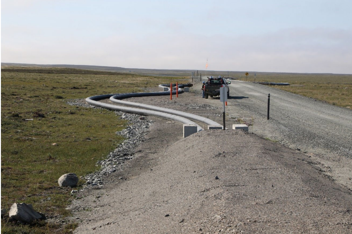
Photo 11: Looking west at raised waterline and the crossing under the AWAR same location as Photo 9.
