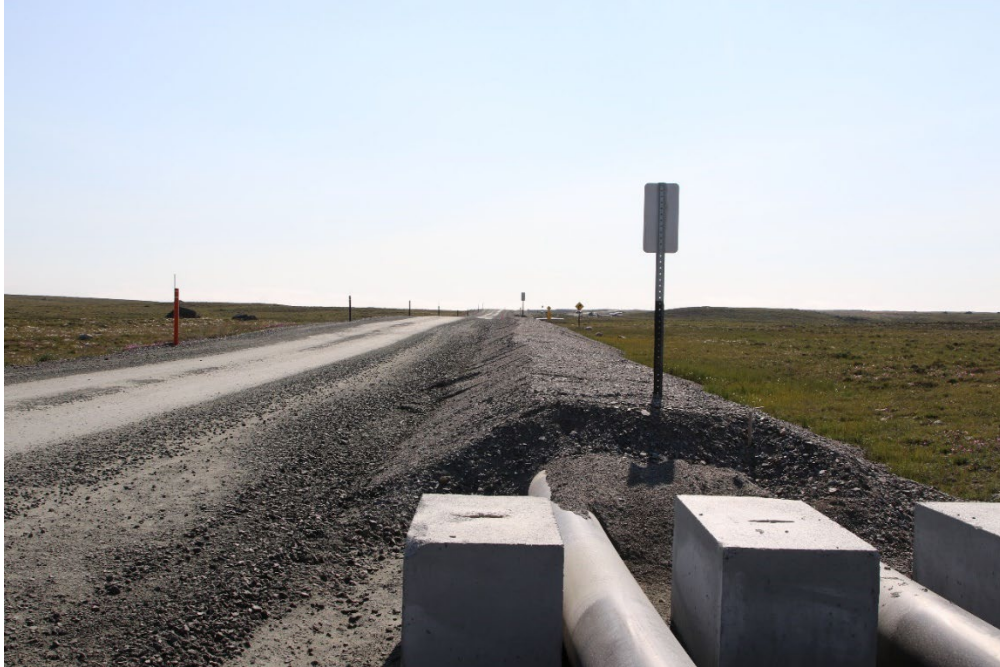
Photo 21: Raised waterline profile, waterline on south side of AWAR looking east.
