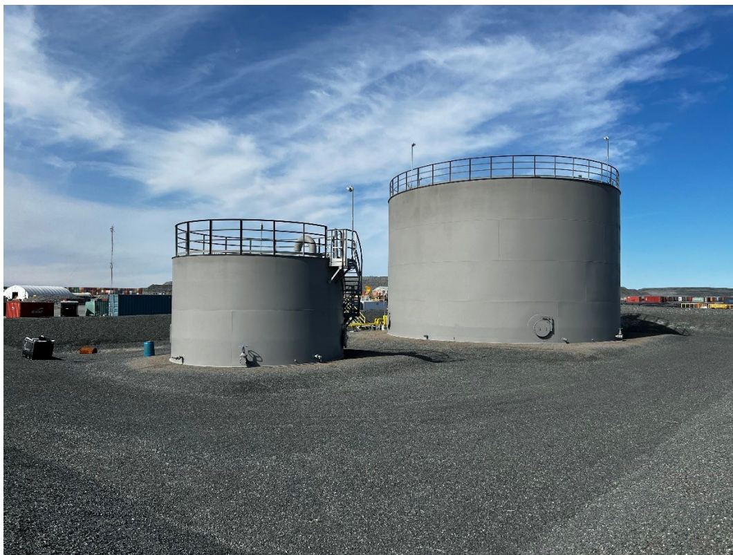
Photo 45: On-site fuel storage in secondary containment.
