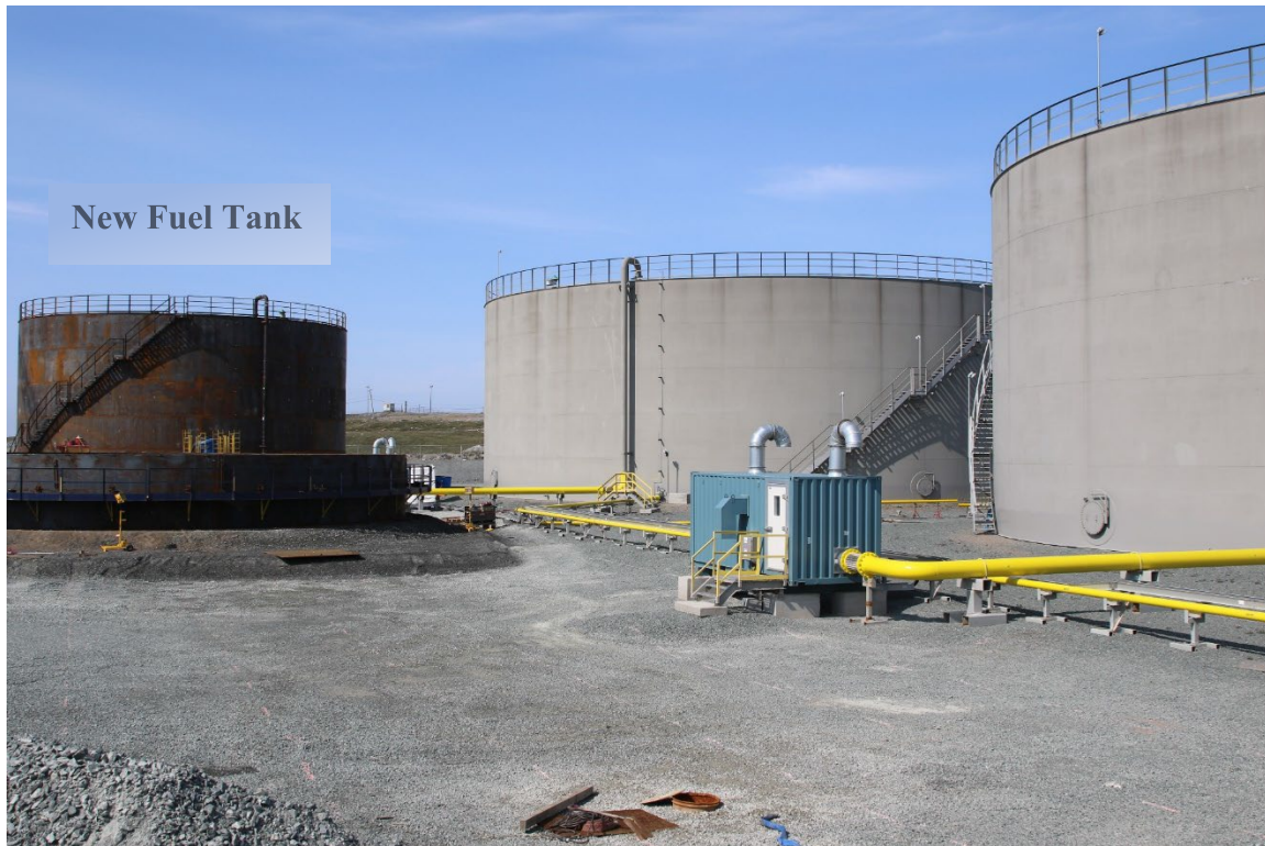
Photo 3: Fuel tanks at Itivia Harbour within secondary containment.
