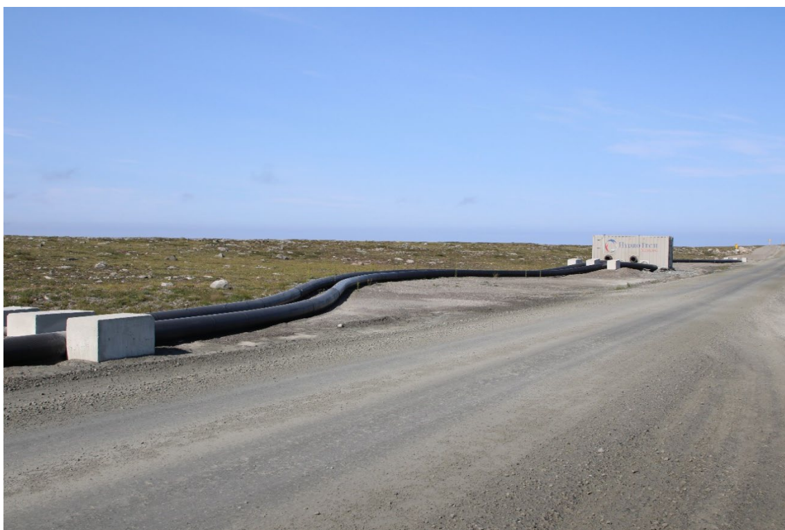
Photo 18: One of several lift stations along AWAR to help send saline effluent to Itivia Harbour.
