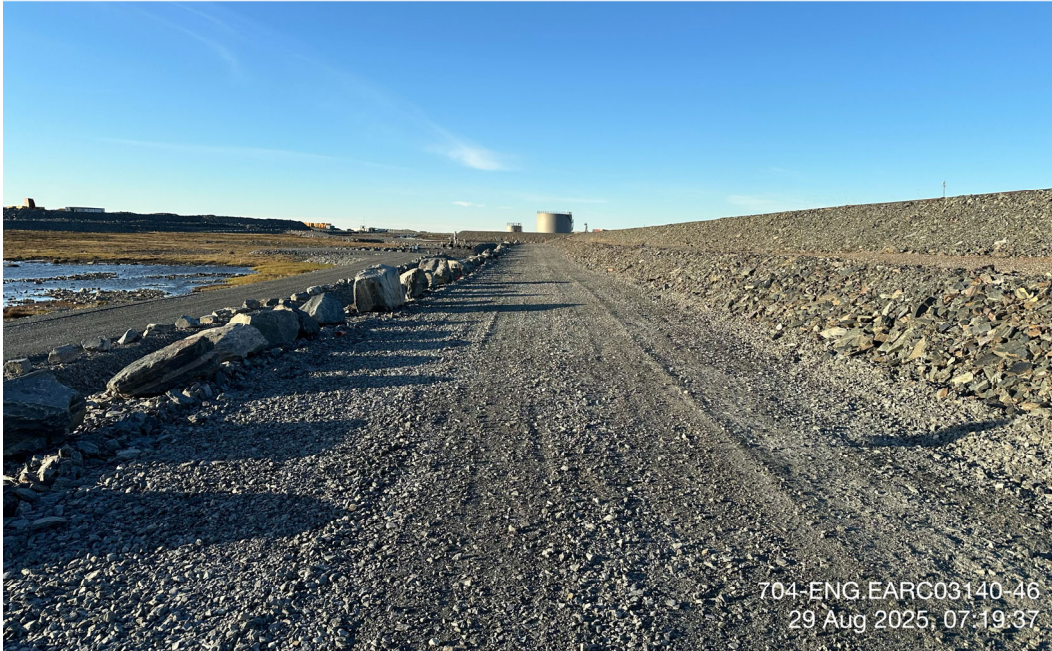
D-CP1 - Photo 7: Dike D-CP1: Dike downstream toe berm view. Facing south.
