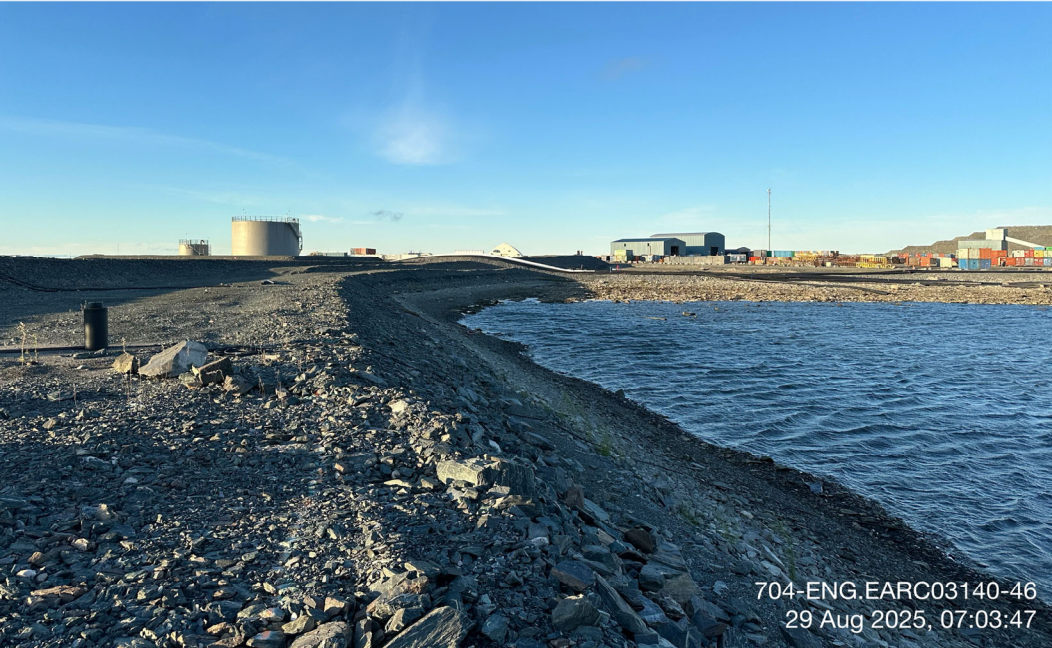
D-CP1 - Photo 6: Dike D-CP1: Dike upstream crest - minor cracking, no change from previous years. Facing southwest.
