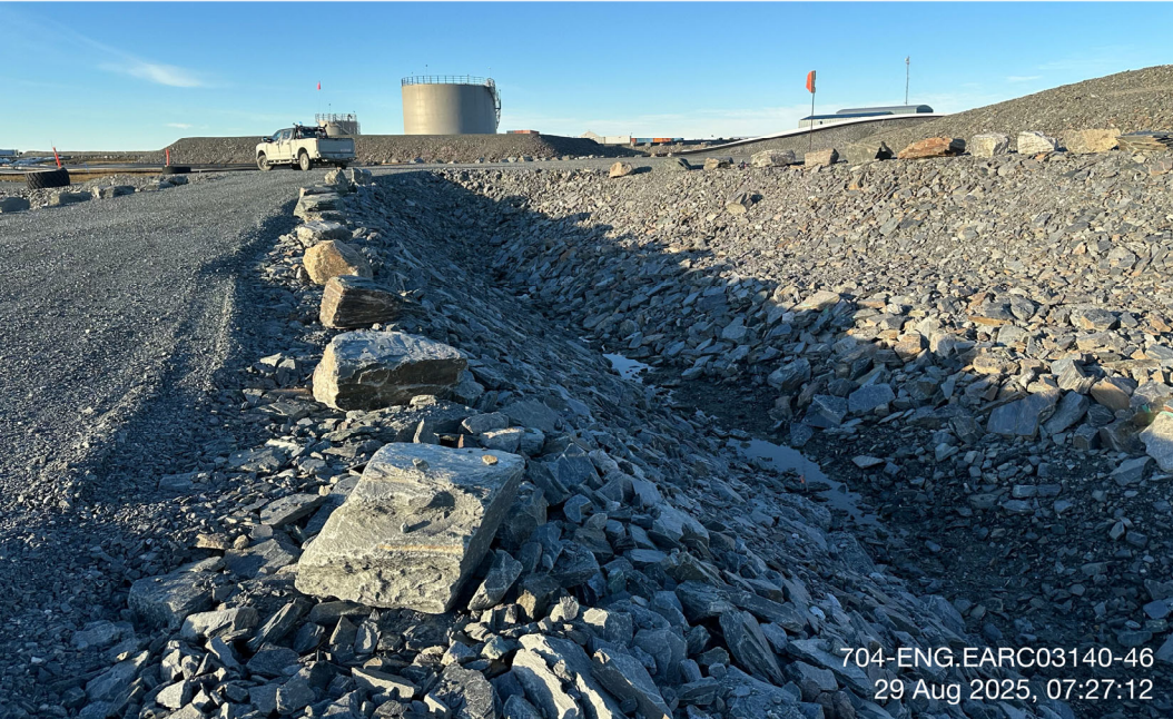
D-CP1 - Photo 10: Dike D-CP1: Dike downstream runoff/seepage collection south ditch. Facing south.
