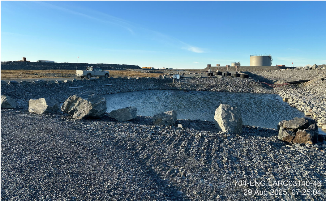
D-CP1 - Photo 12: Dike D-CP1: Dike downstream collection sump. Facing south.
