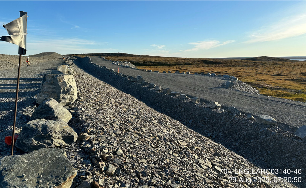
D-CP1 - Photo 8: Dike D-CP1: Dike downstream runoff/seepage collection north ditch. Facing northeast.
