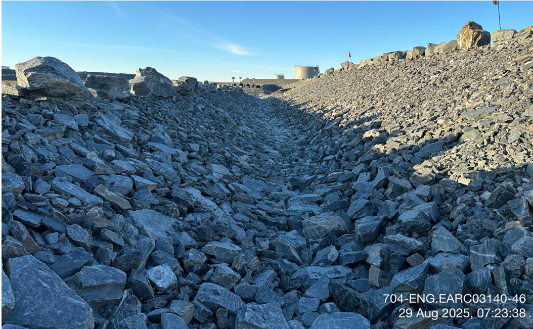
D-CP1 - Photo 9: Dike D-CP1: Dike downstream runoff/seepage collection north ditch. Facing south.
