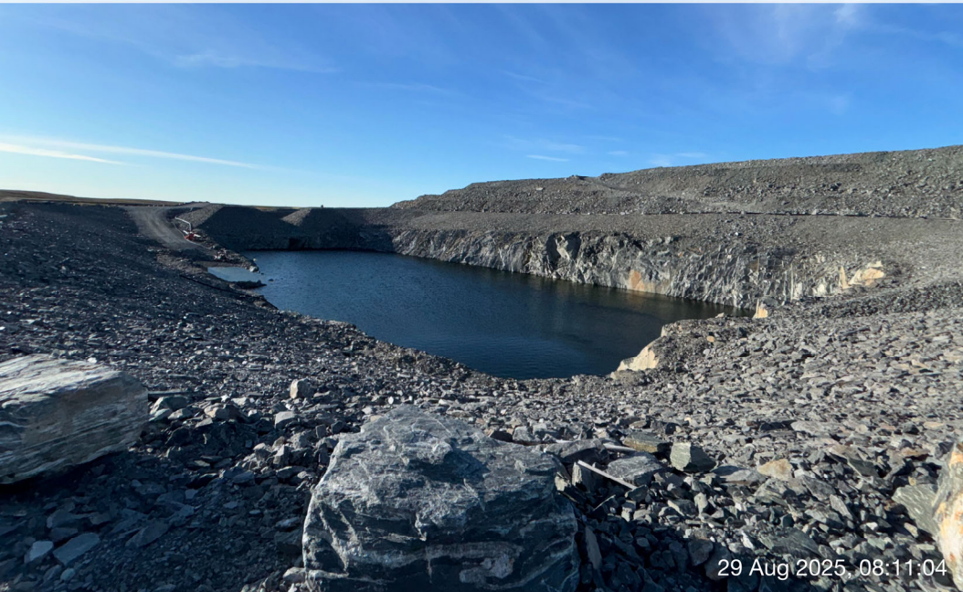
CP2 - Photo 2: CP2: Water stored in CP2. Facing south.
