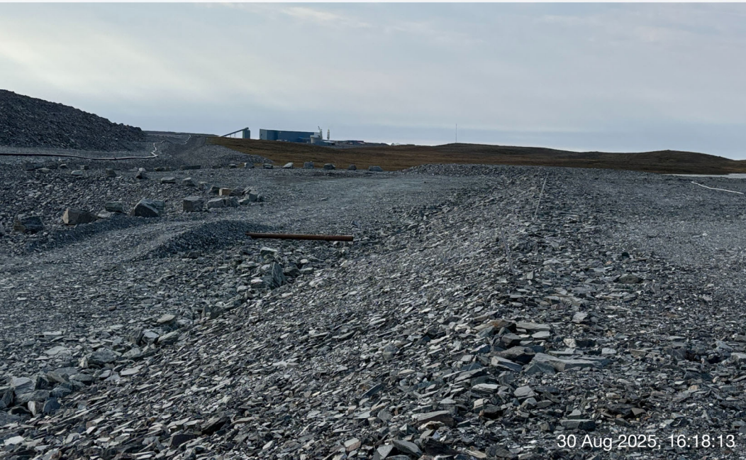
CP2 Thermal Berm - Photo 6: CP2 Thermal Berm: Upstream of thermal berm and area of additional ROM cover placed in 2024. Facing northwest.
