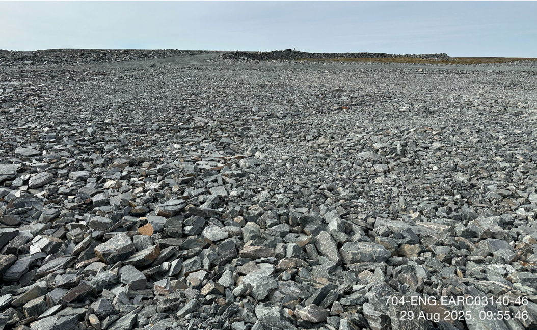
CP4 Thermal Berm - Photo 4: CP4 Thermal Berm: Overview of crest, performing well, no stability concern. Facing southwest.
