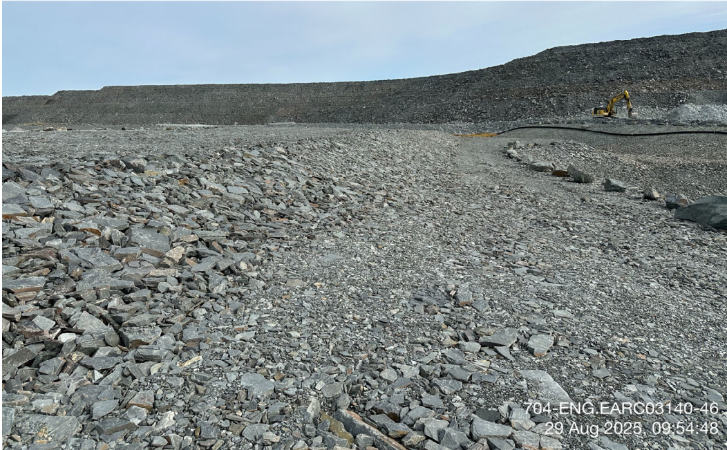
CP4 Thermal Berm - Photo 7:
