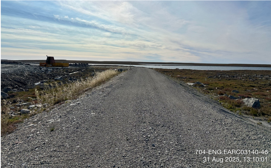
Berm2 - Photo 9: Berm2: Overview of Berm2 north portion, slope and crest, performing well, no stability concern. Facing southwest.
