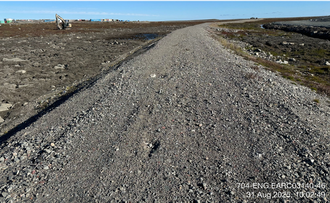
Berm2 - Photo 10: Berm2: Overview of Berm2 middle portion, slope and crest, performing well, minor cracking observed on crest and slopes, no stability concern, ponded water on both sides. Facing north.
