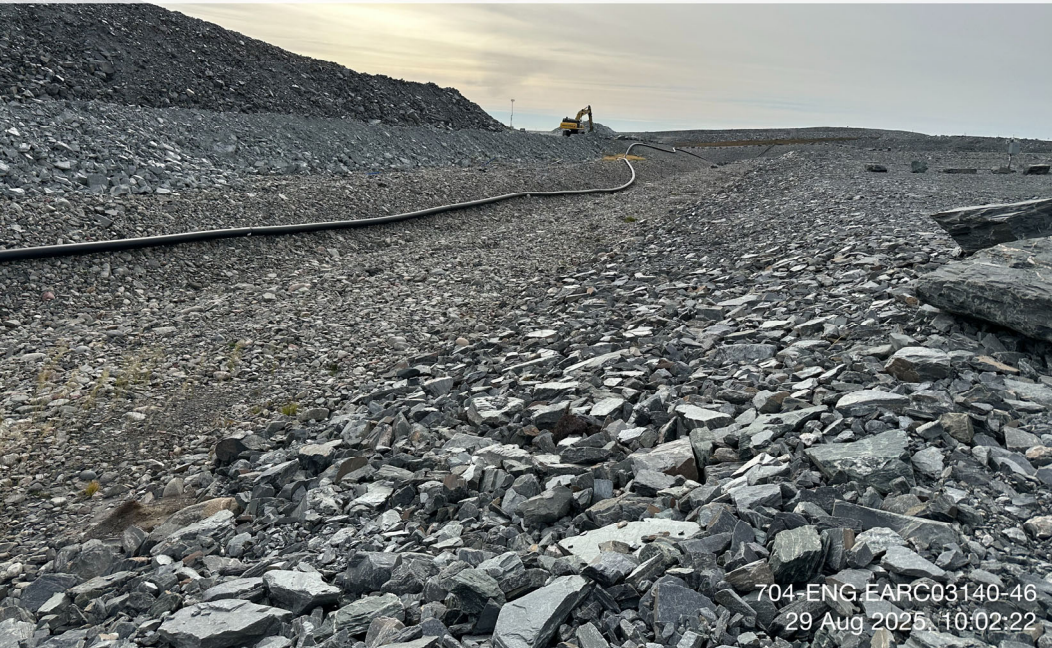
CP4 Thermal Berm - Photo 8:
