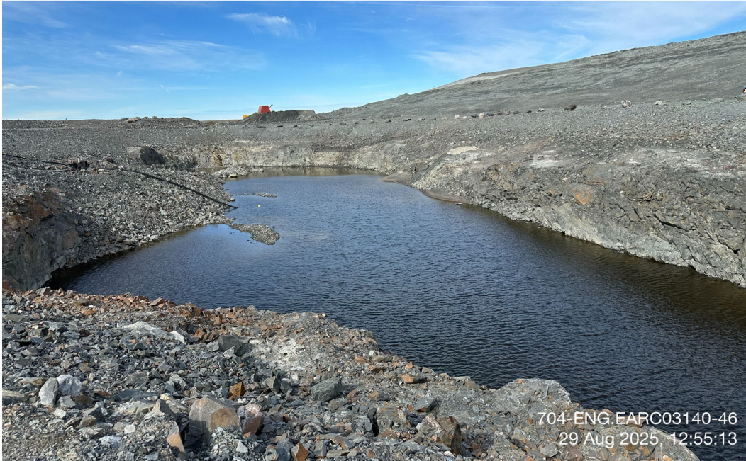
CP3 - Photo 1: CP3: Small amount of water stored in CP3, bedrock slopes with fractured rock, no stability concern. Facing north.
