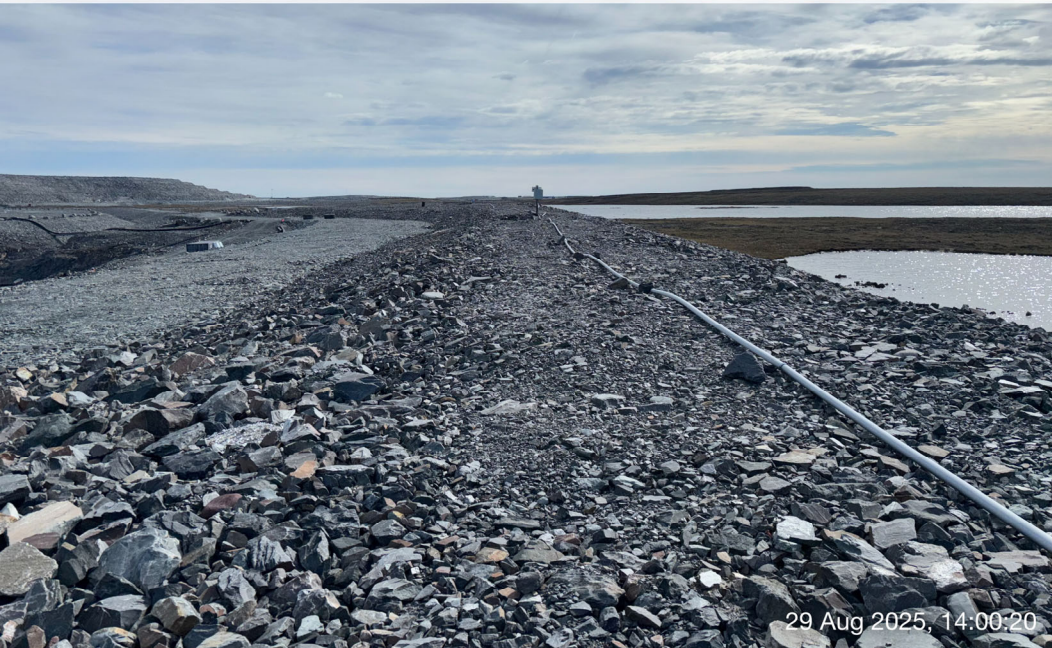
CP3 Thermal Berm - Photo 4: CP3 Thermal Berm: Crest of CP3 Thermal Berm, minor thaw settlement observed, similar conditions to the previous year. Facing southeast.
