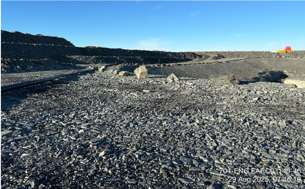
CP6 - Photo 5: CP6: View of east side perimeter, cover placed between CP6 and WRSF3. Facing west.
