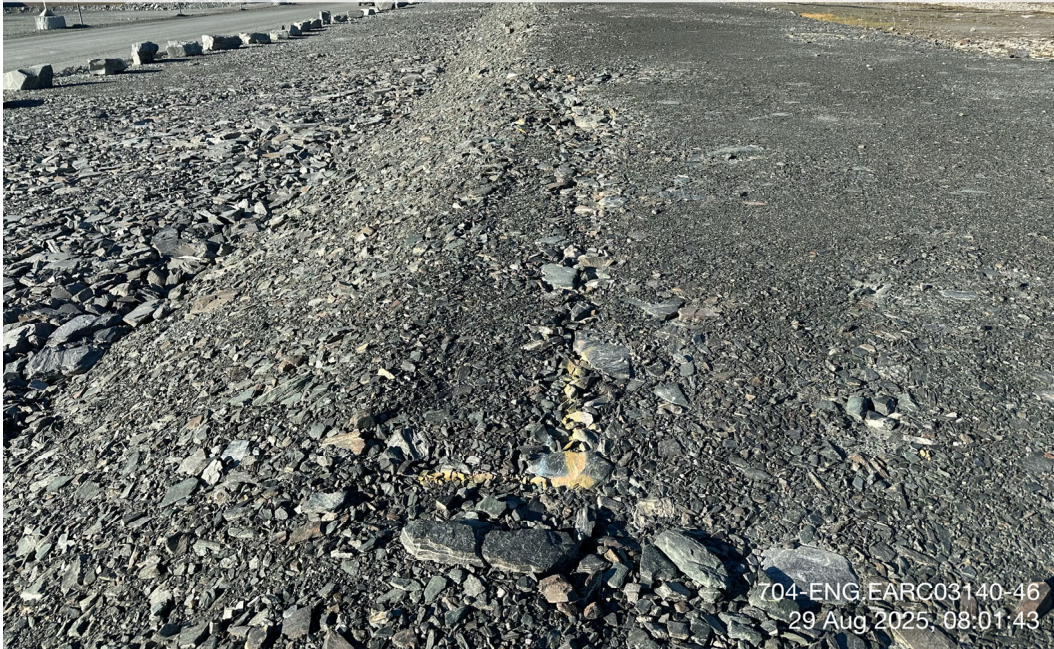
D-CP5 - Photo 4: Dike D-CP5: Overview of D-CP5 downstream side slope, minor cracking observed similar to previous years. Facing southwest.
