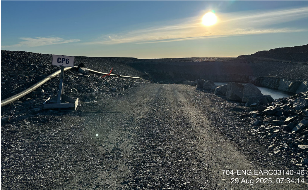
CP6 - Photo 1: CP6: Overview of ramp entering CP6. Facing east.
