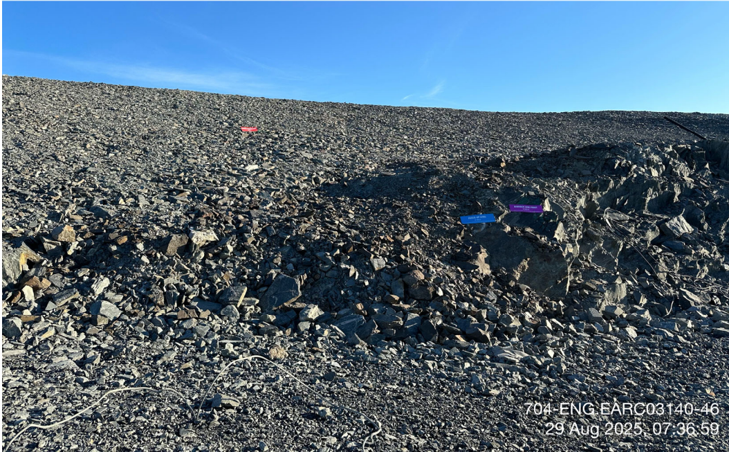
CP6 Thermal Berm - Photo 9:
