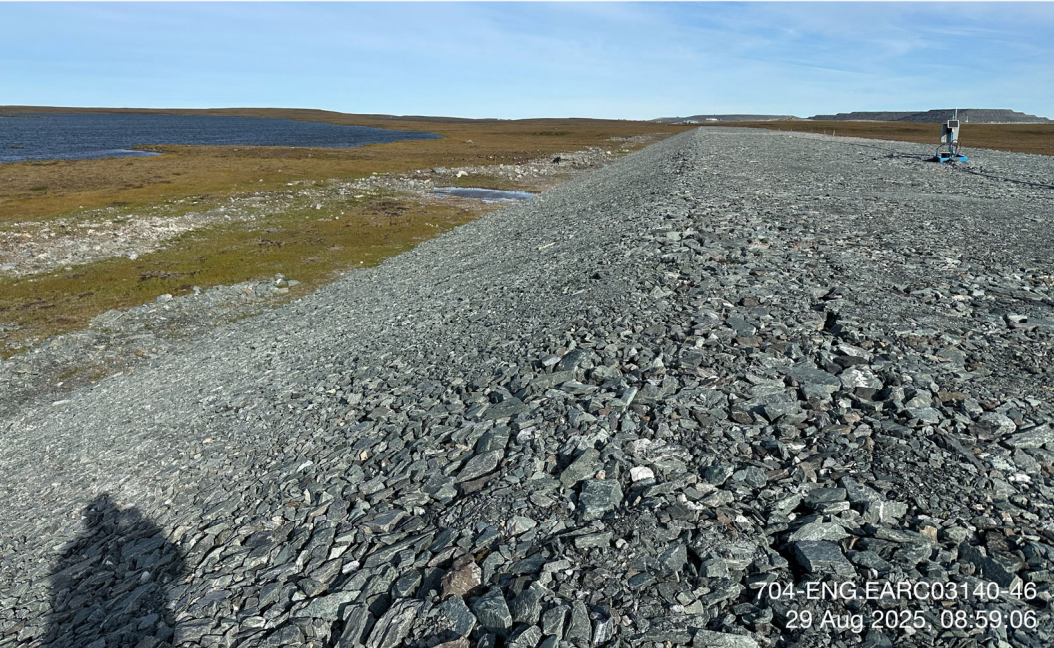
CP9 Thermal Berm - Photo 2:
