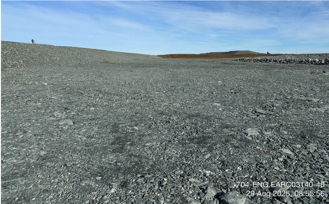
CP9 Thermal Berm - Photo 1:
