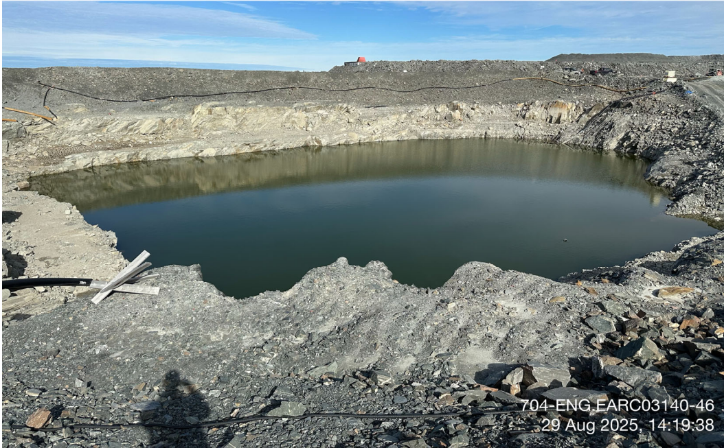
SP1 - Photo 1: SP1 Saline Pond: Overview of SP1, pond in bedrock, rockfill covered overburden slopes. Facing Northeast.
