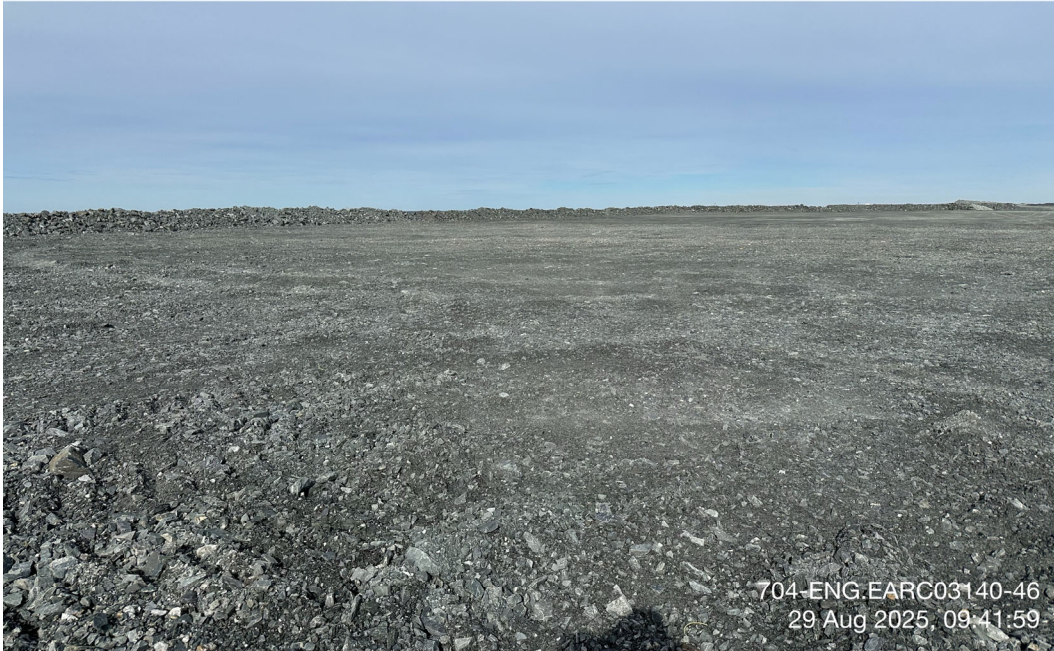
WRSF1 - Photo 1: WRSF1: Overview of WRSF1 crest. Facing northwest.
