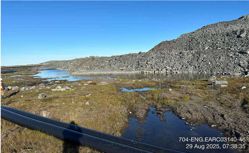
WRSF3 - Photo 4: WRSF3: Overview of ponded water observed at southwest corner of WRSF3. Facing west.
