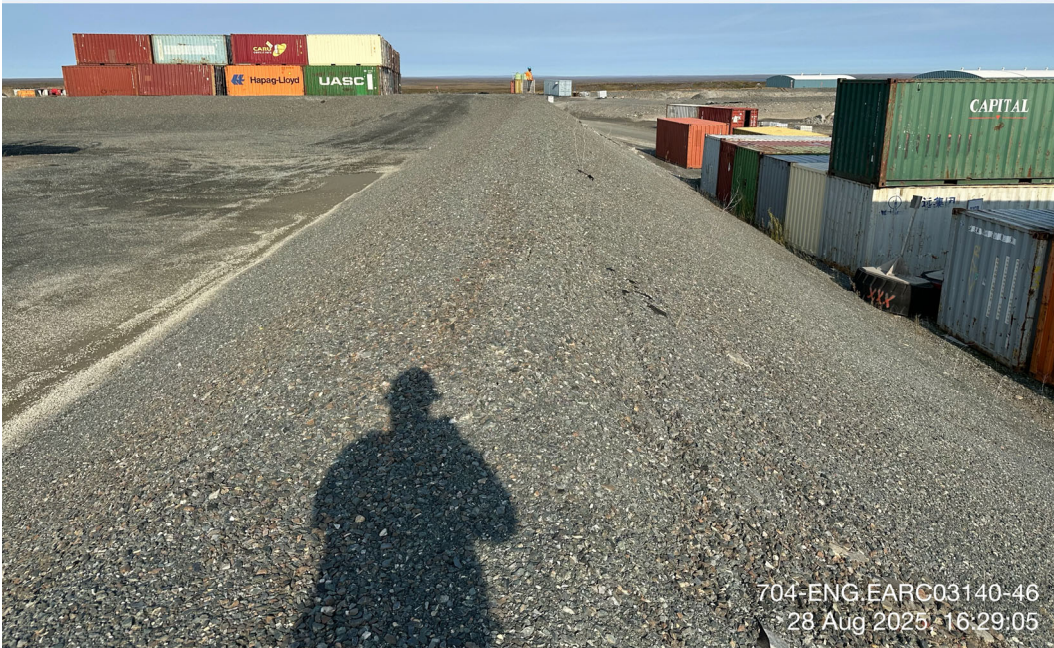
Industrial Fuel Tank Farm - Photo 22: Industrial Fuel Tank Farm: South side berm overview, cracking on crest. Facing northeast.
