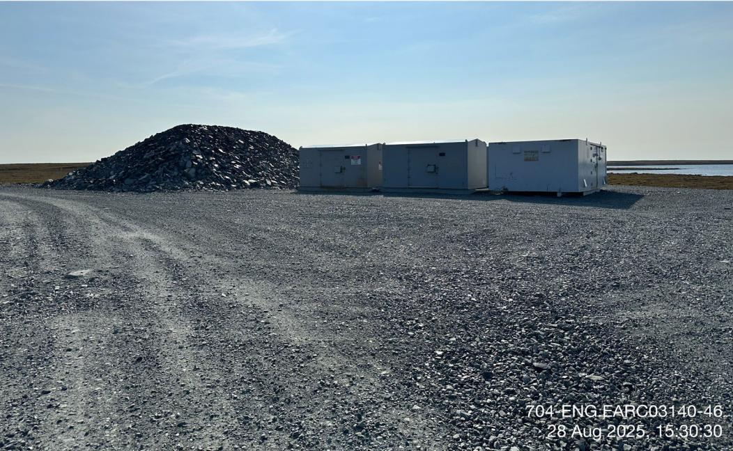
Emulsion Plant Pad - Photo 12: Emulsion Storage Pad: Overview of pad and storage. Facing south.
