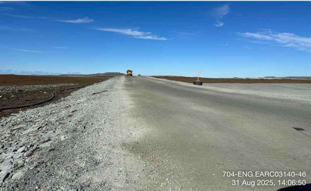
Site Road - Photo 10:
