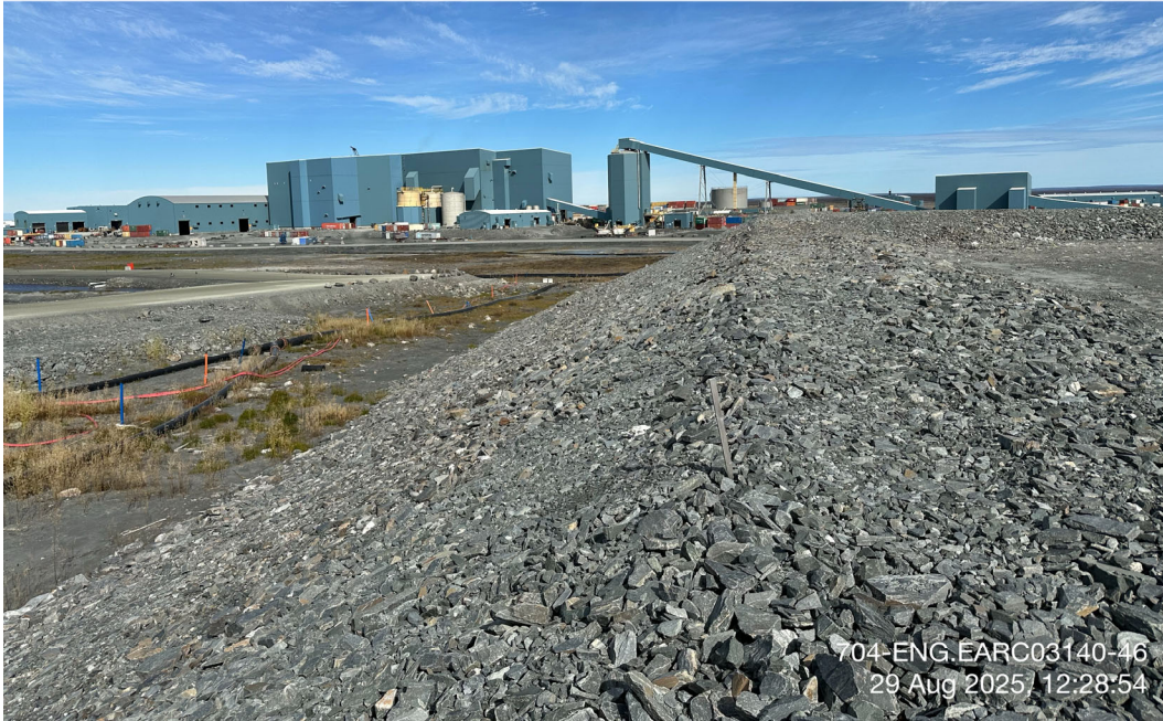
Landfill - Photo 7: WRSF1 Landfill: Landfill north side slope overview, minor settlement on crest/slope, minor cracking on crest. Facing northeast.
