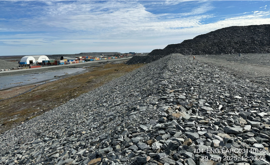
Landfill - Photo 6: WRSF1 Landfill: Landfill east side slope overview. Facing southeast.
