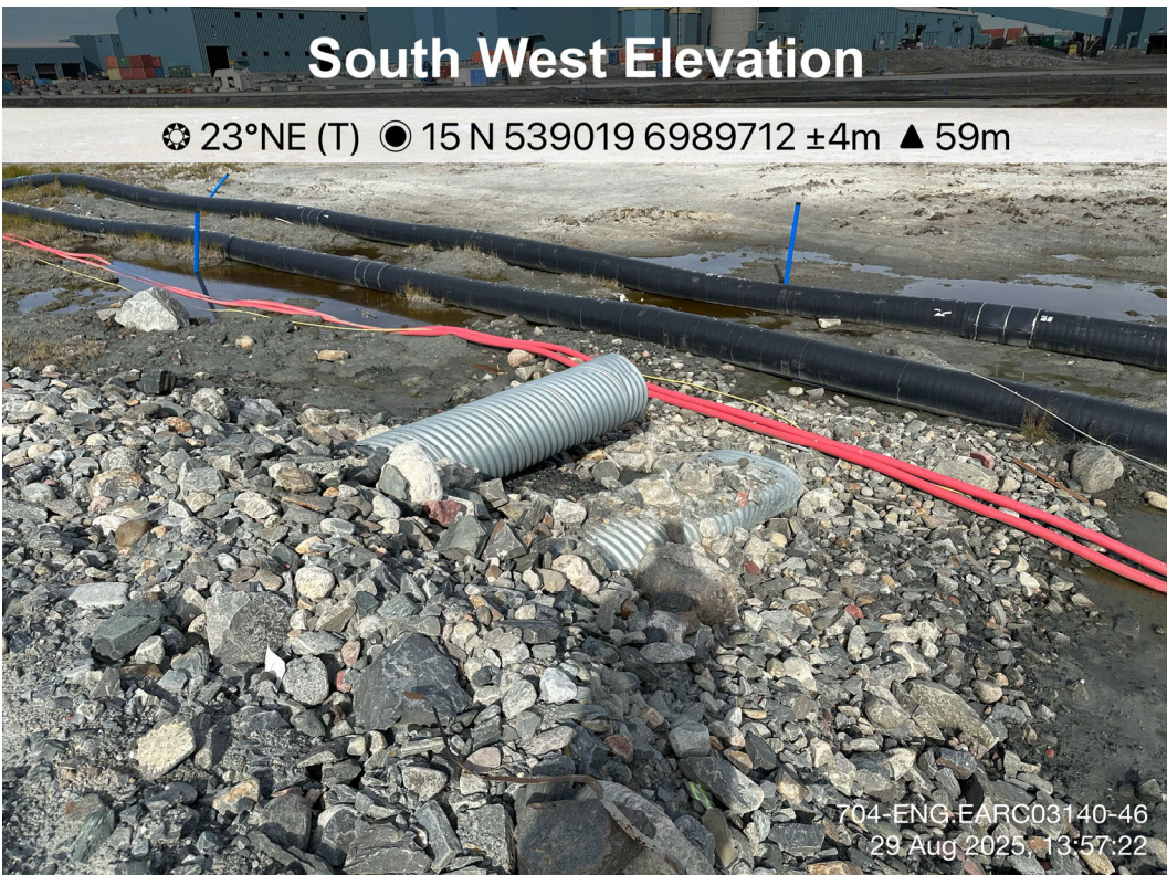
Site Road - Photo 14:
