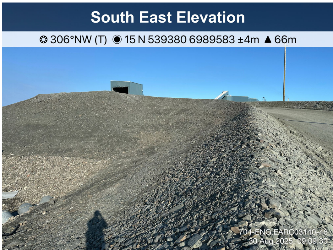
Crusher Ramp - Photo 2: Crusher Ramp: Ramp side slope overview. Facing northwest.
