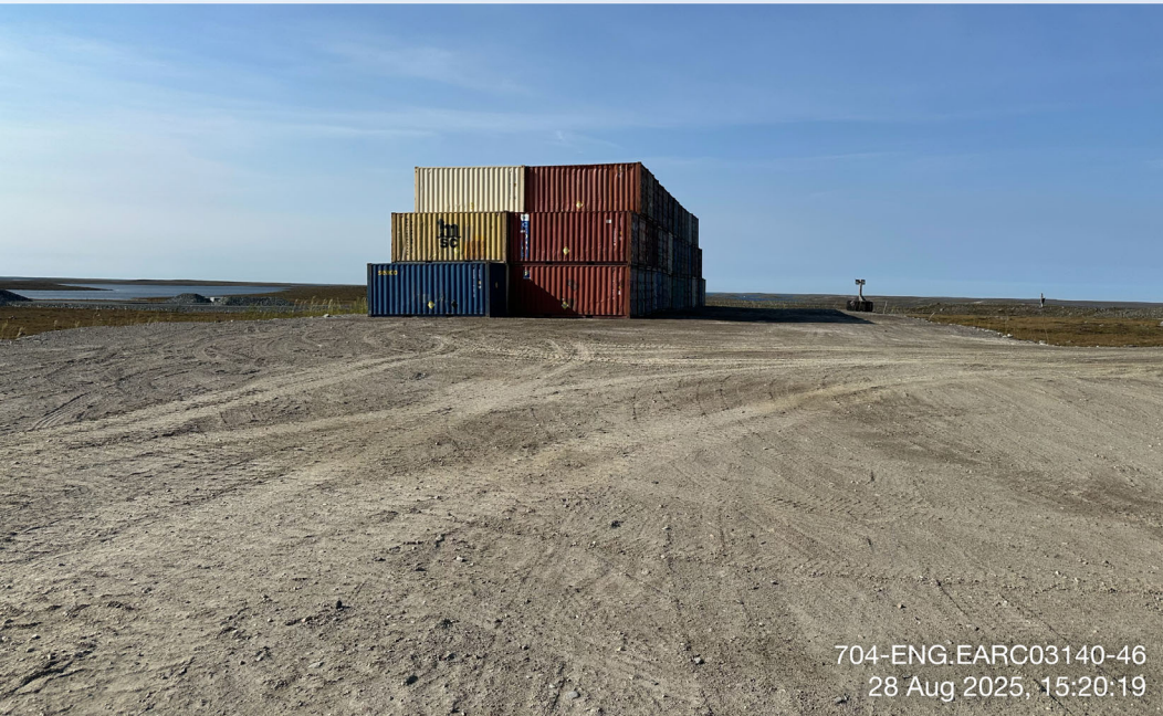
Emulsion Plant Pad - Photo 10: Emulsion Plant Pad: Overview of pad, small depressions and ponding water. Facing northwest.
