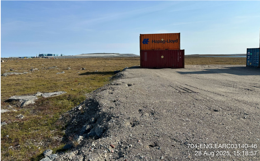
Emulsion Plant Pad - Photo 9: Emulsion Plant Pad: Overview of pad. Facing southeast.
