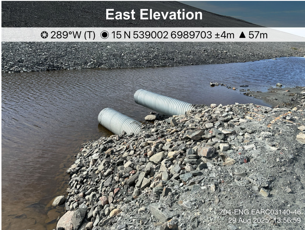
Site Road - Photo 13:
