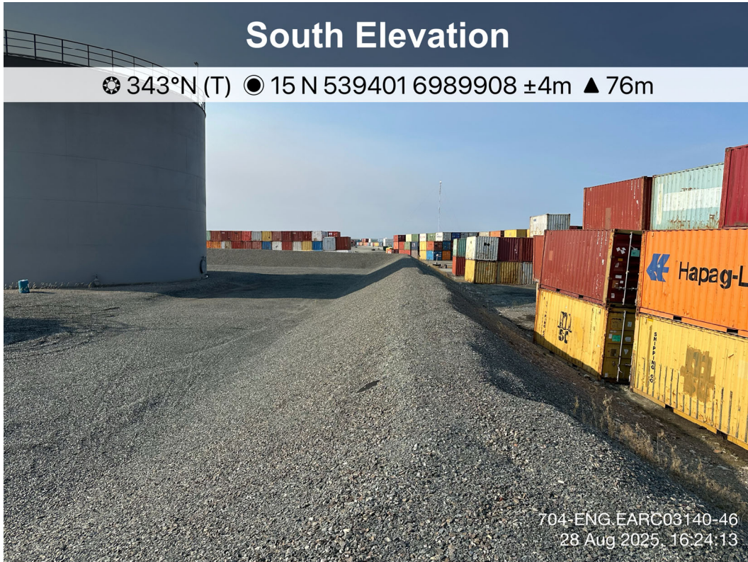
Industrial Fuel Tank Farm - Photo 19:
