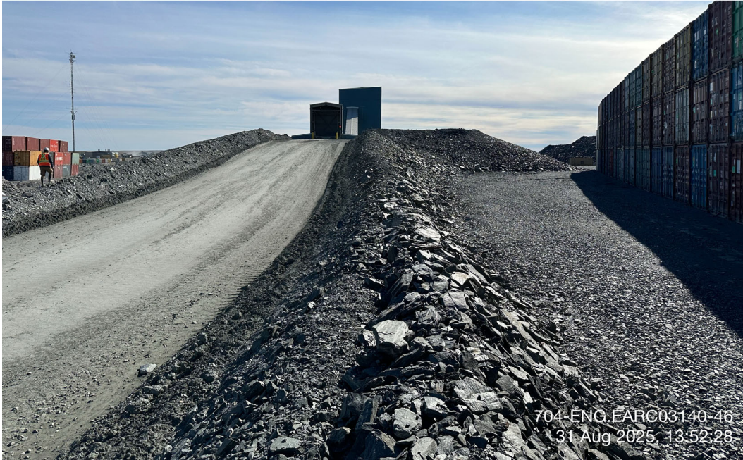
Site Road - Photo 9:
