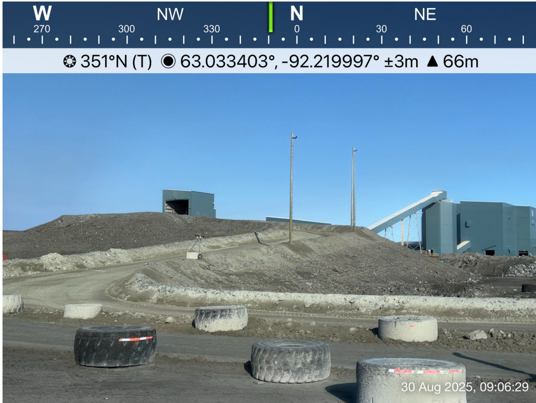
Crusher Ramp - Photo 1: Crusher Ramp: Overview of crusher ramp. Facing north.
