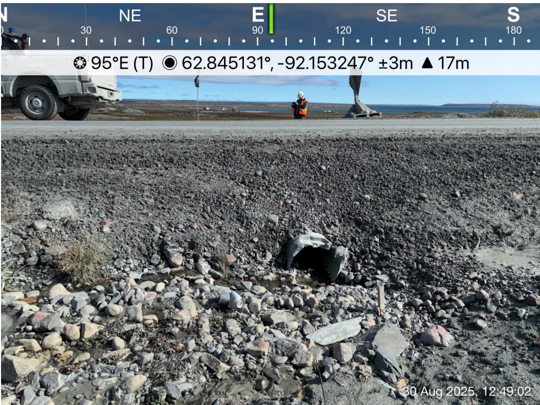
AWAR Road/ Culvert - Photo 4: Culvert KM 4.1: Inlet.
