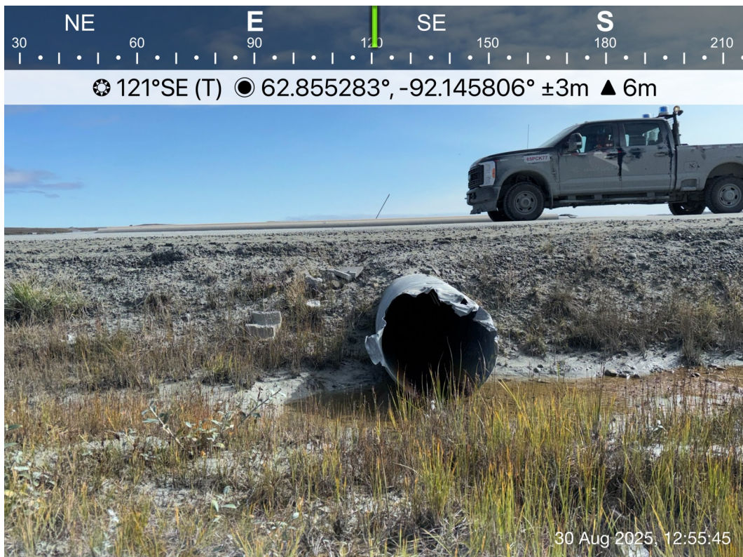
AWAR Road/ Culvert - Photo 8: Culvert KM 5.4: Inlet.
