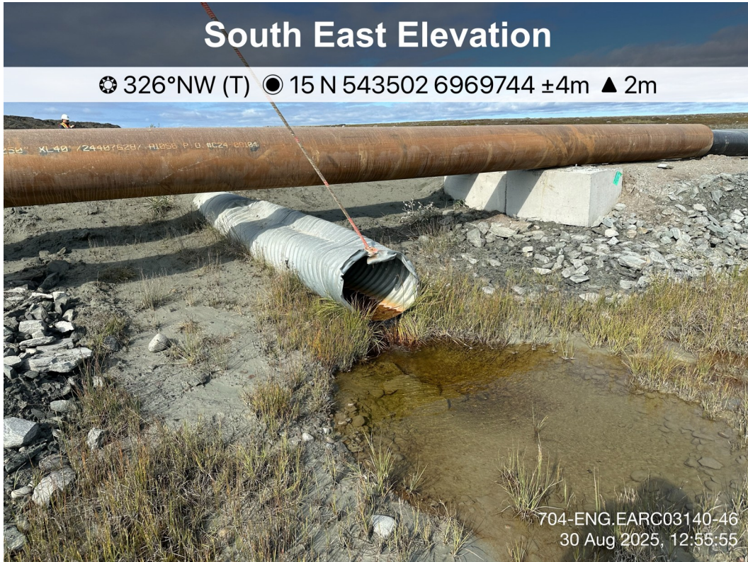
AWAR Road/ Culvert - Photo 7: Culvert KM 5.4: Outlet.
