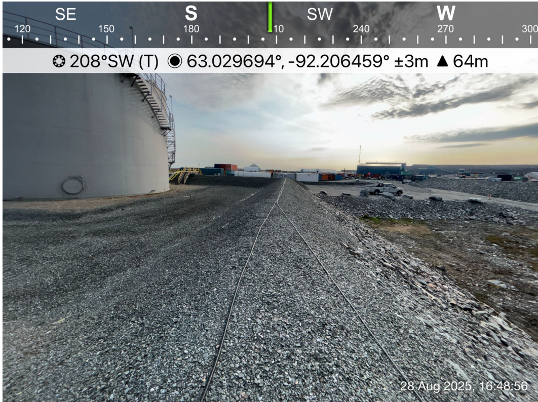
Mine Site Fuel Tank Farm - Photo 33:
