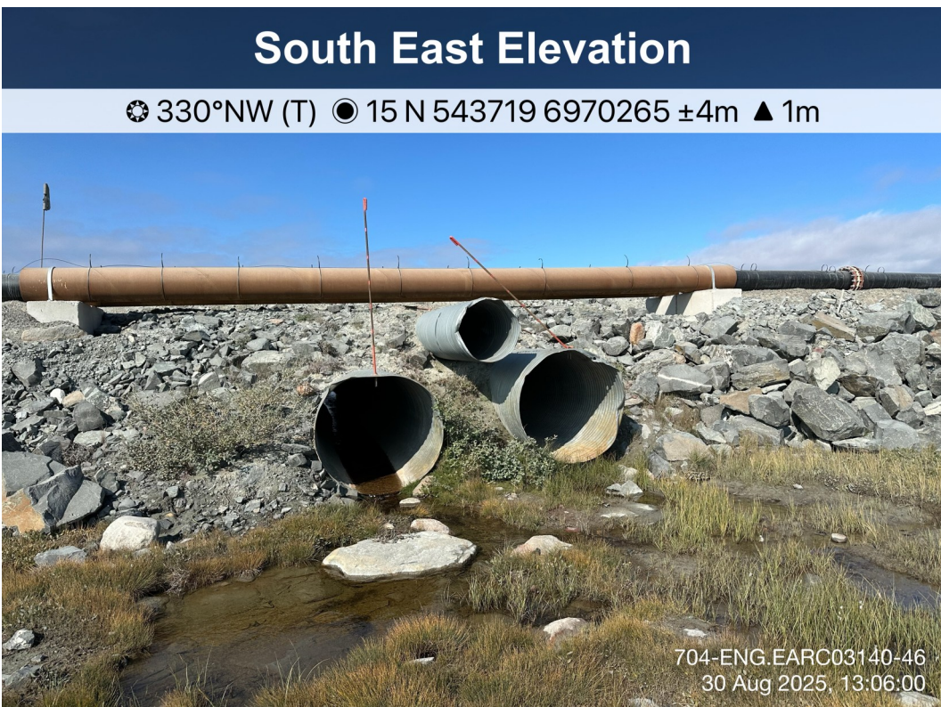
AWAR Road/ Culvert - Photo 12: Culvert KM 6.1: Outlet.
