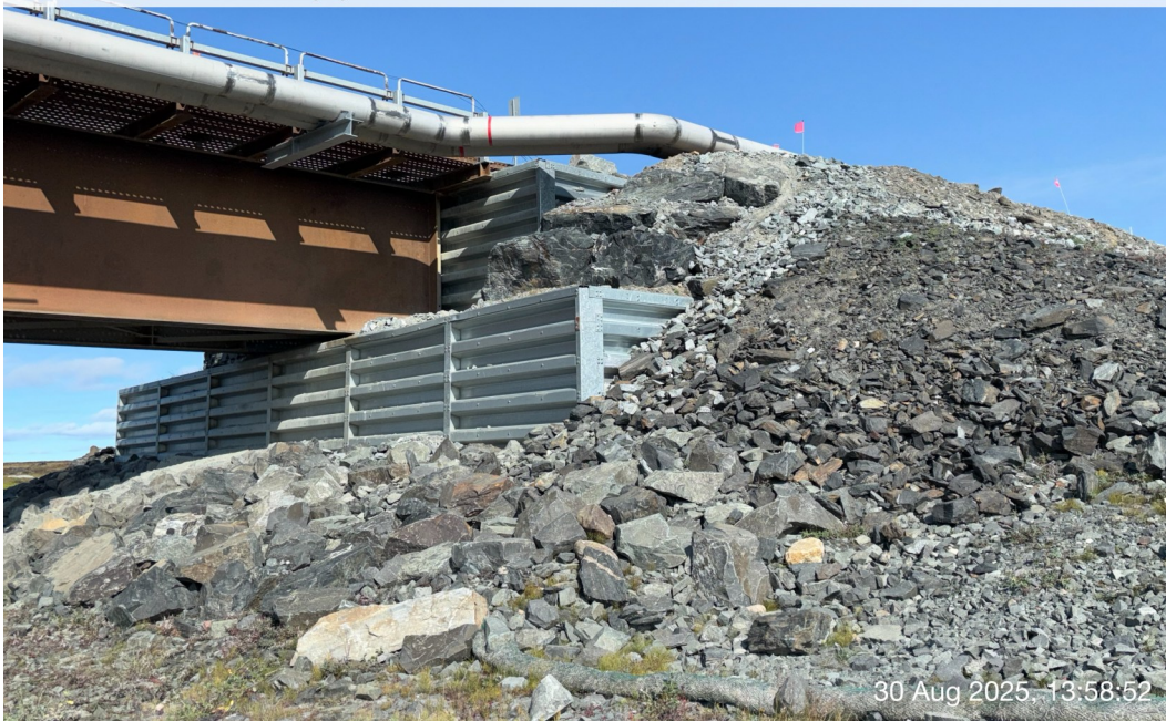
AWAR Road/ Culvert - Photo 22: Meliadine River Bridge KM 8.0: East abutment.
