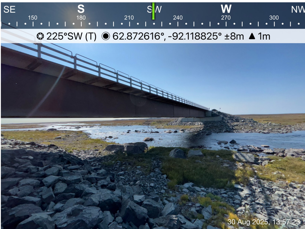
AWAR Road/ Meliadine River Bridge KM 8.0. Culvert - Photo 20:
