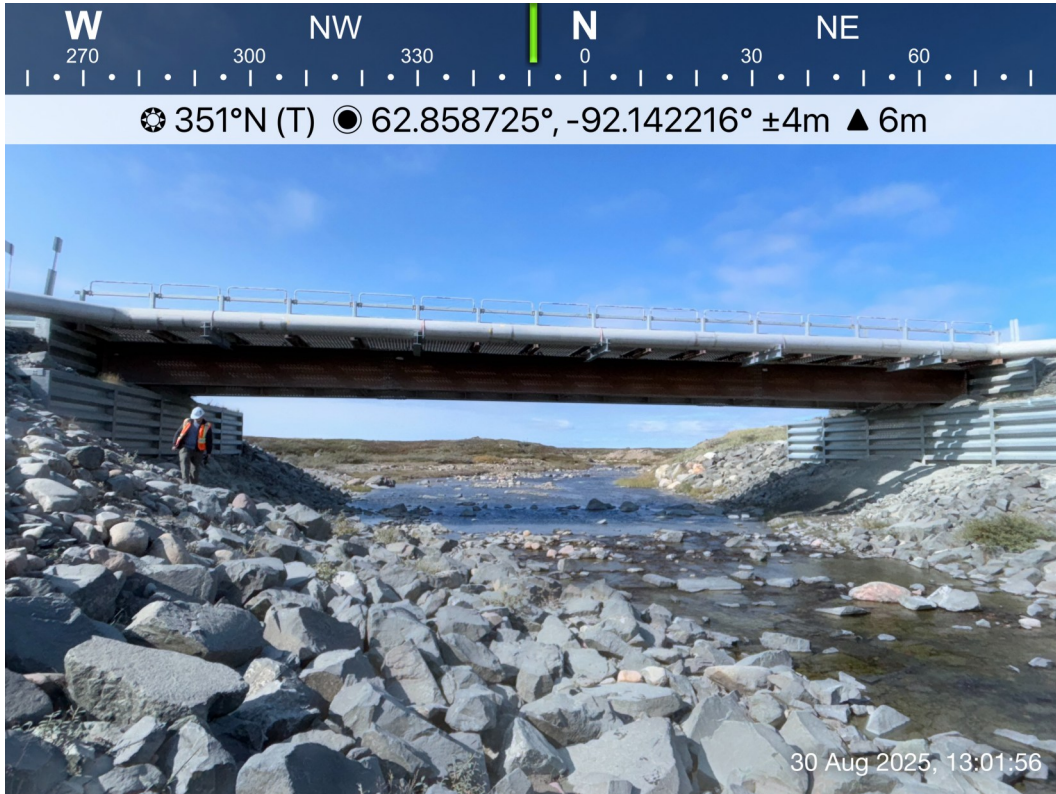
AWAR Road/ Culvert - Photo 9: Char River Bridge KM 6.0: Overview.
