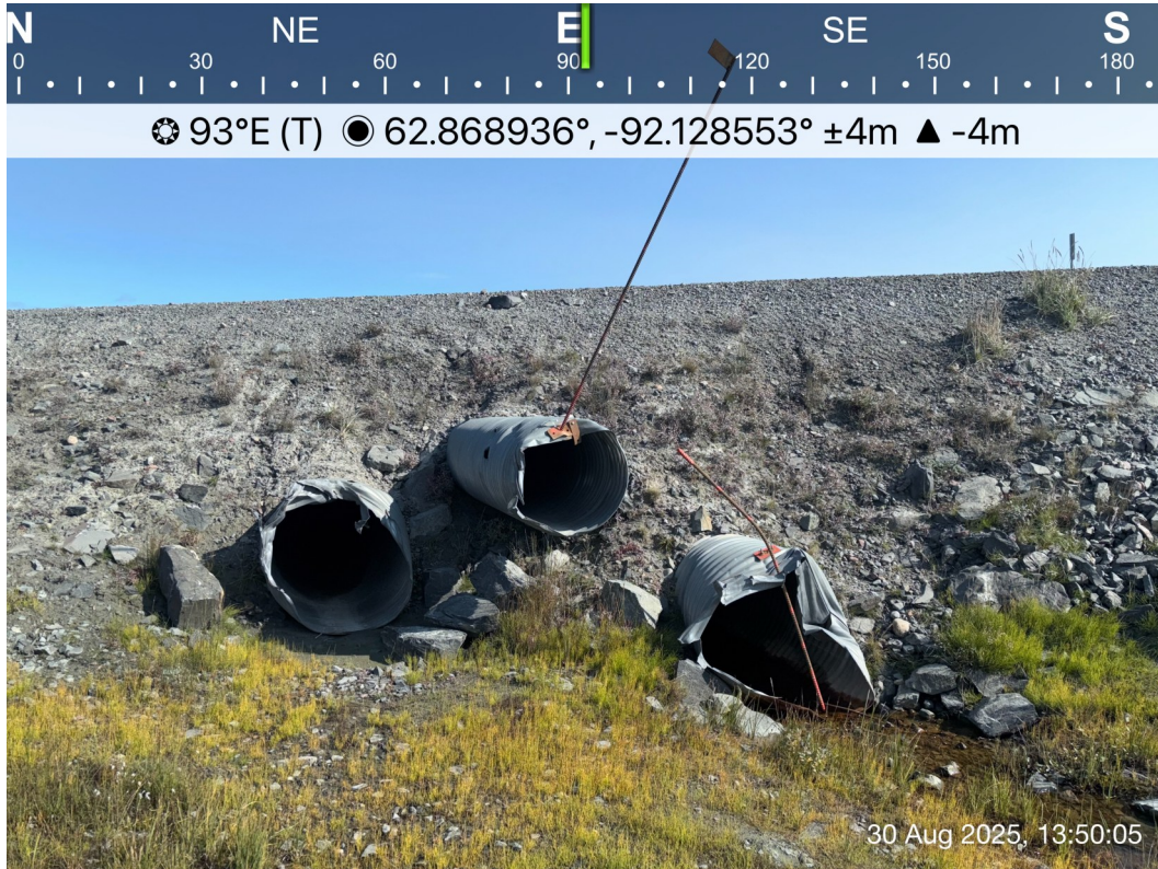
AWAR Road/ Culvert KM 7.35: Inlet. Culvert - Photo 19:
