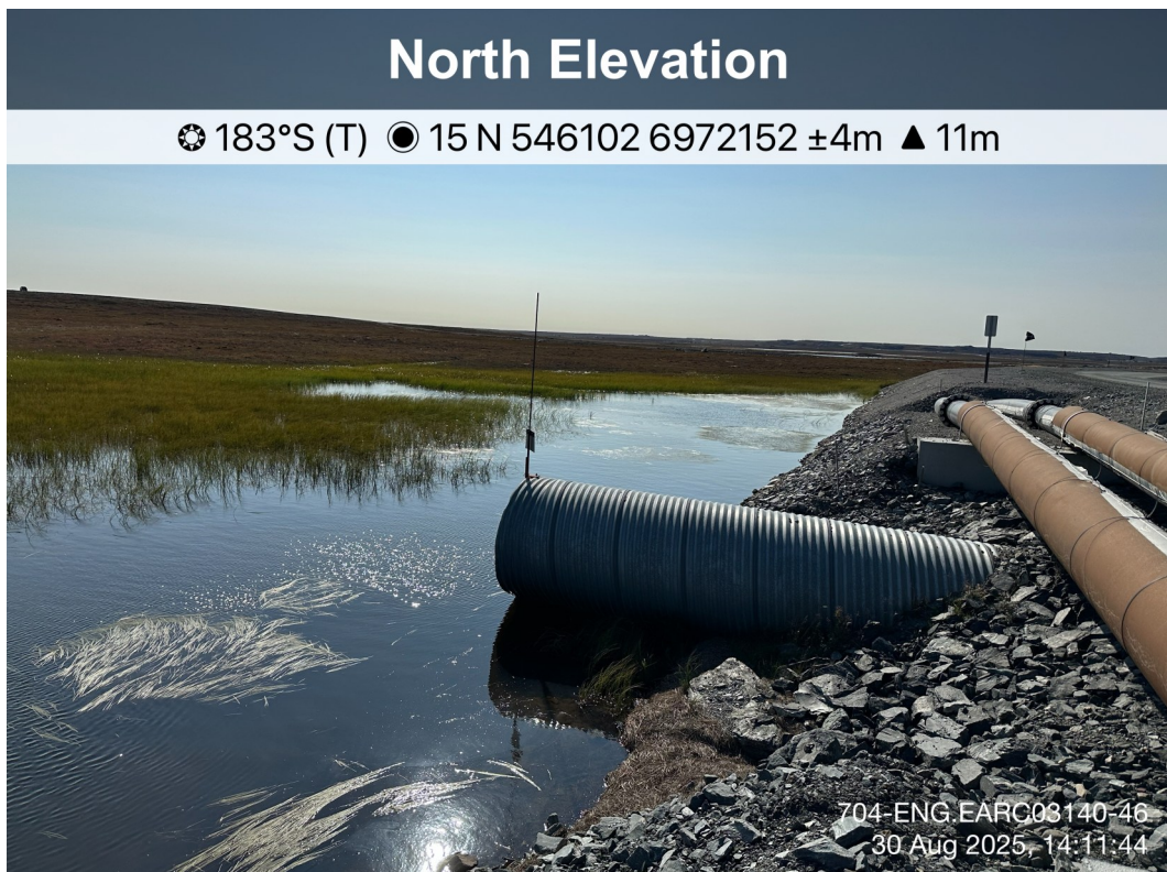
AWAR Road/ Culvert KM 9.6: Inlet. Culvert - Photo 30:
