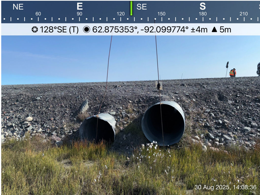
AWAR Road/ Culvert KM 9.3: Inlet. Culvert - Photo 29:
