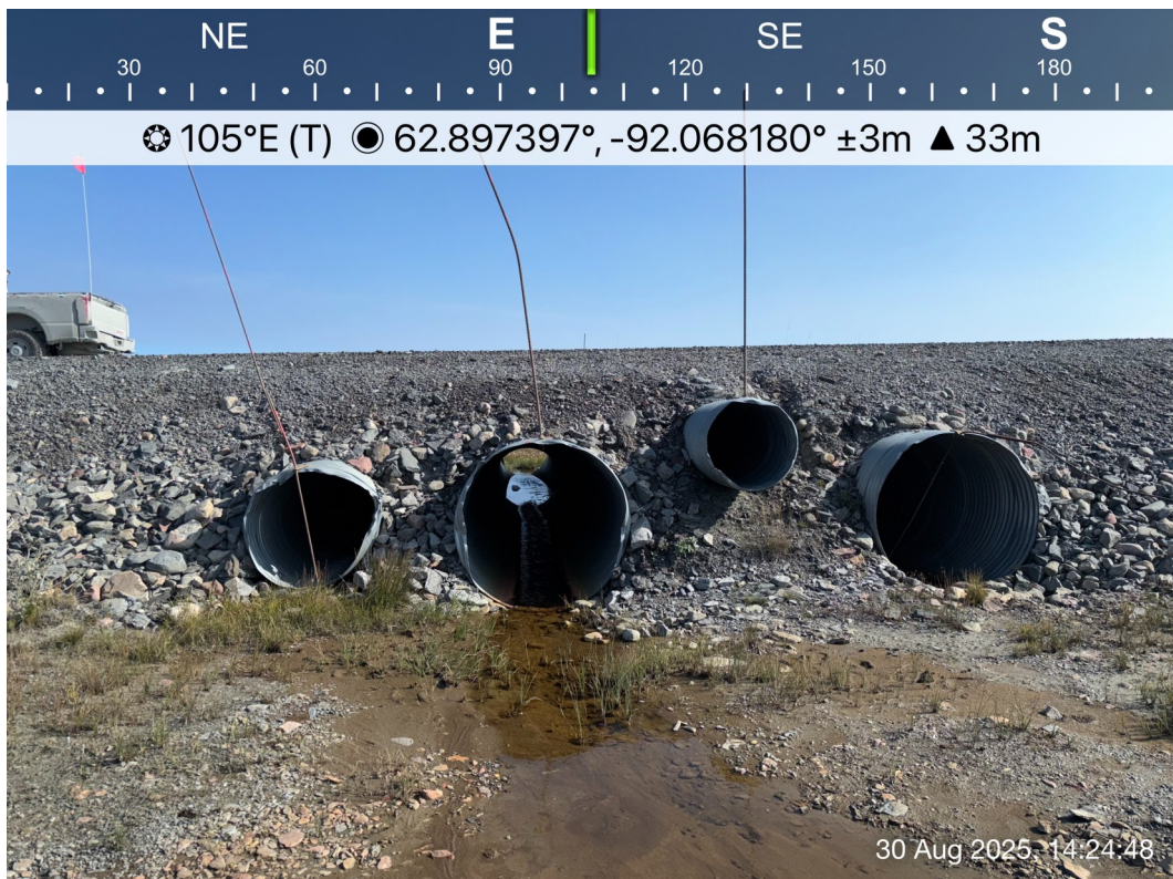
AWAR Road/ Culvert KM 12.2: Outlet. Culvert - Photo 36:
