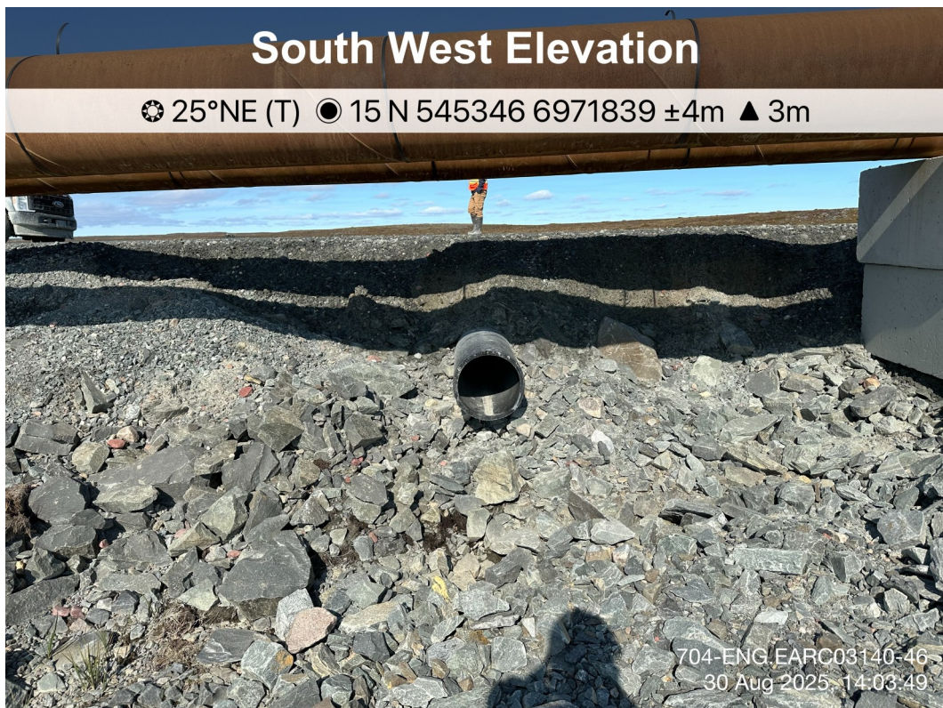
AWAR Road/ Culvert - Photo 24: Pipe Sleeve KM 8.7: Outlet.
