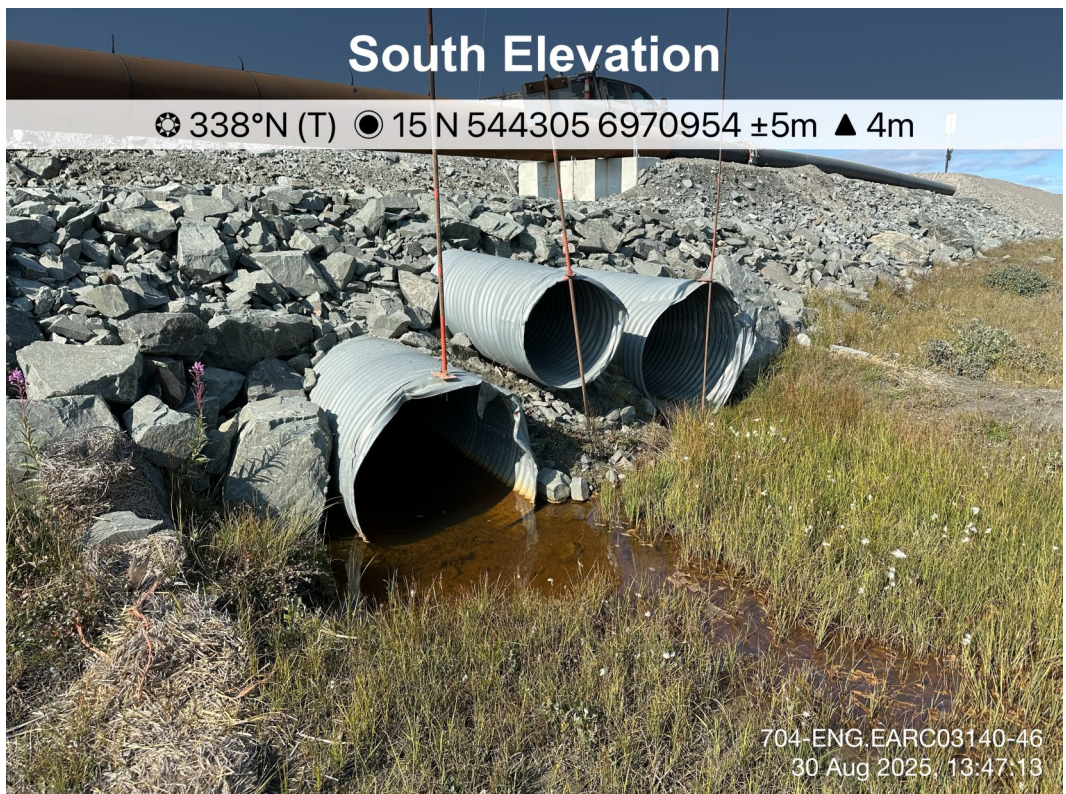
AWAR Road/ Culvert - Photo 16: Culvert KM 7.0: Outlet.
