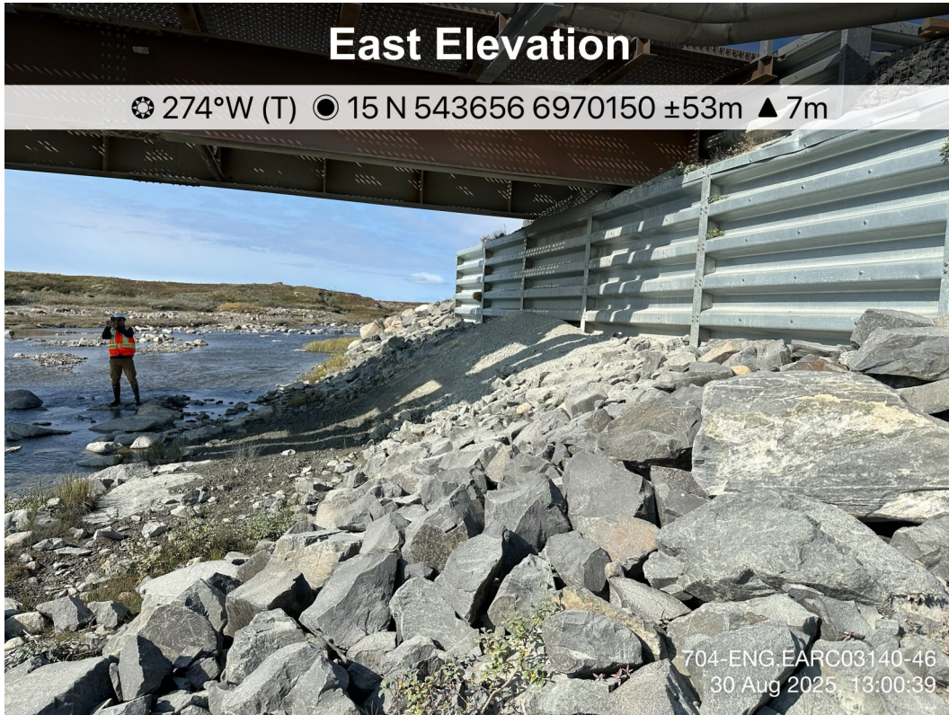
AWAR Road/ Culvert - Photo 11 Char River Bridge KM 6.0: North Abutment.
