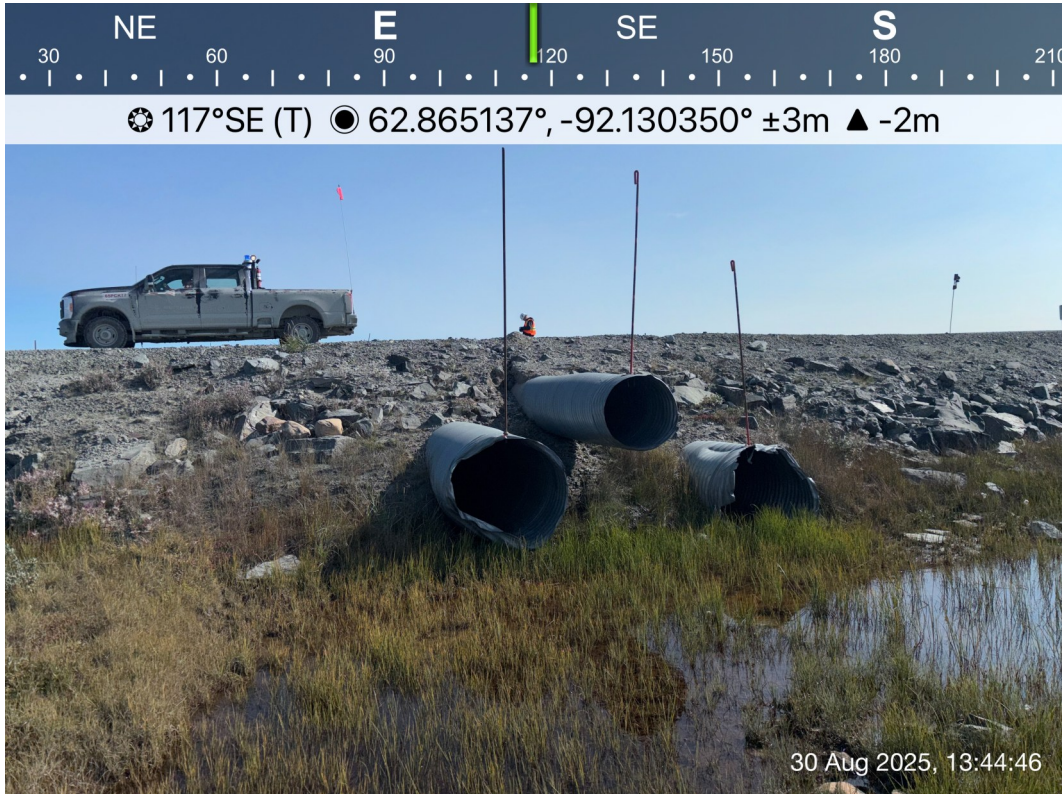
AWAR Road/ Culvert - Photo 15: Culvert KM 6.9: Inlet.
