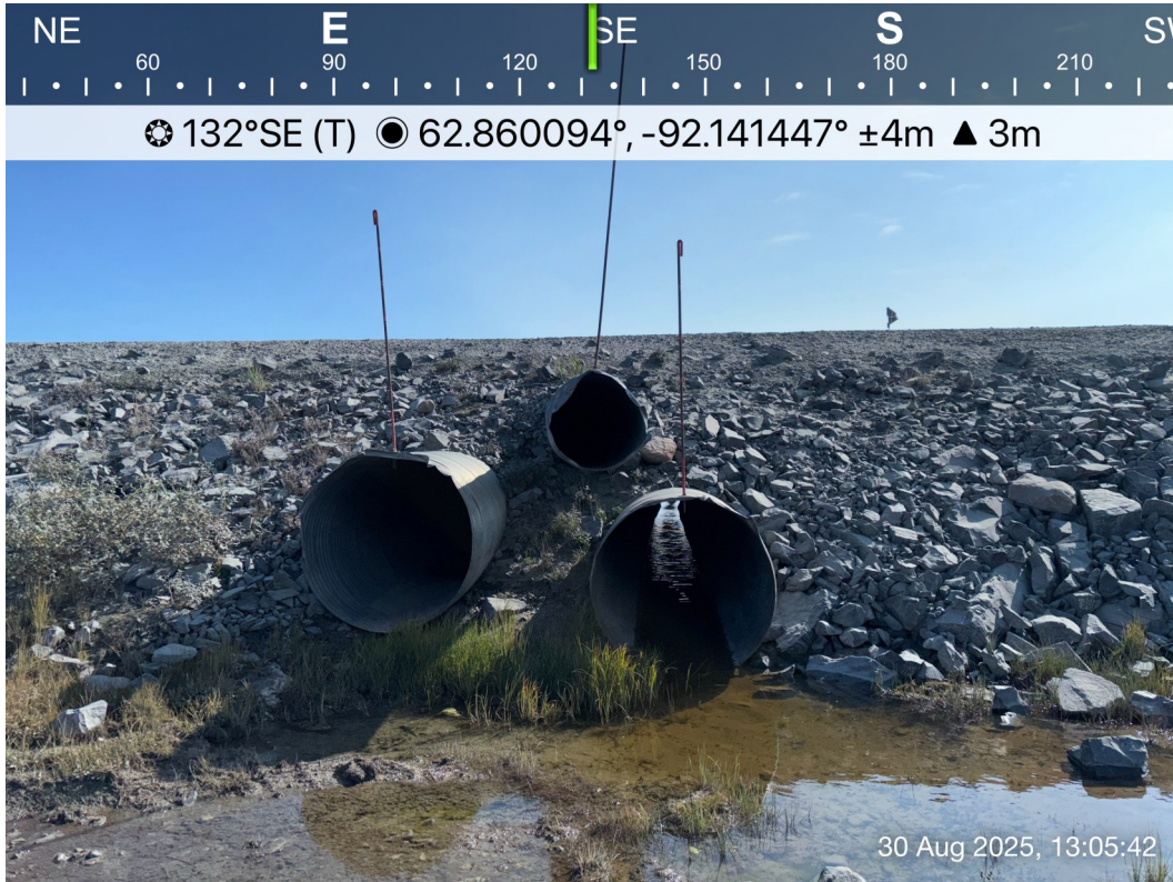
AWAR Road/ Culvert KM 6.1: Inlet. Culvert - Photo 13
