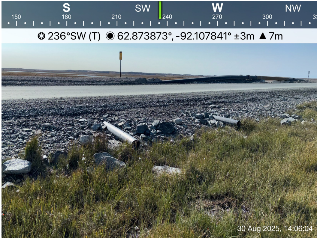
AWAR Road/ Culvert - Photo 27: Pipe Sleeve KM 8.8: Inlet.
