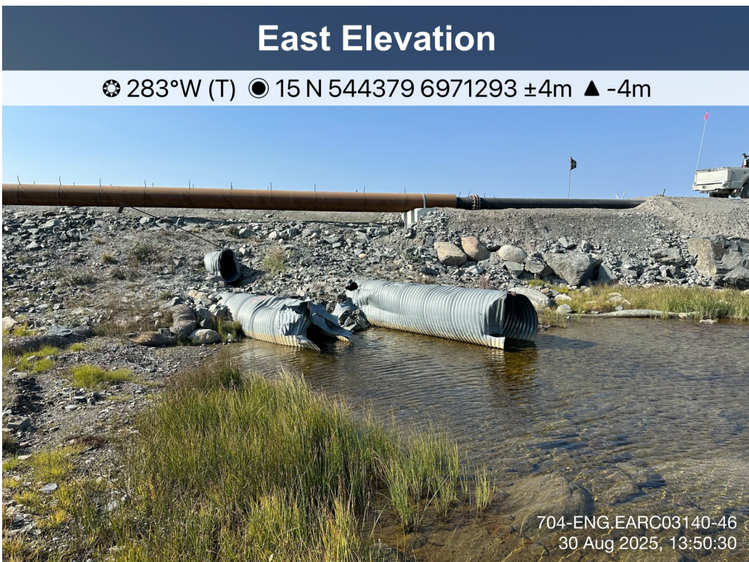
AWAR Road/ Culvert KM 7.35: Outlet. Culvert - Photo 18:
