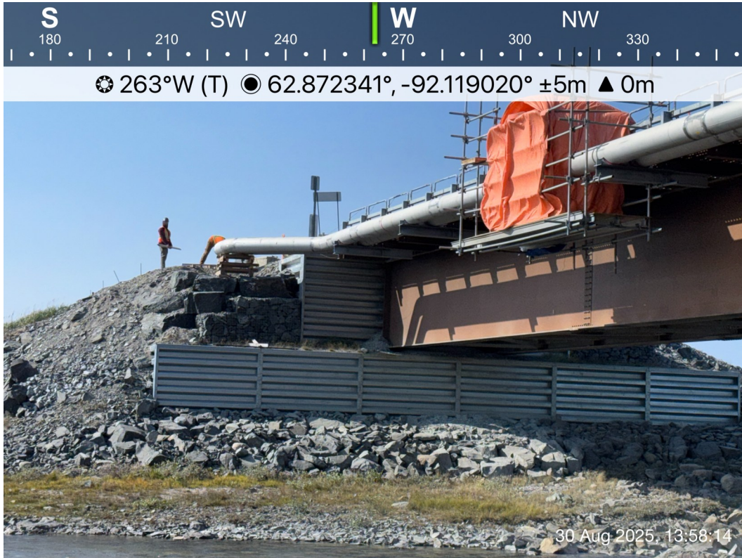
AWAR Road/ Culvert - Photo 23: Meliadine River Bridge KM 8.0: West abutment.
