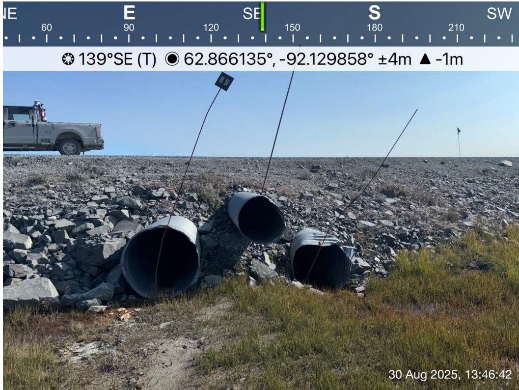
AWAR Road/ Culvert KM 7.0: Inlet. Culvert - Photo 17:
