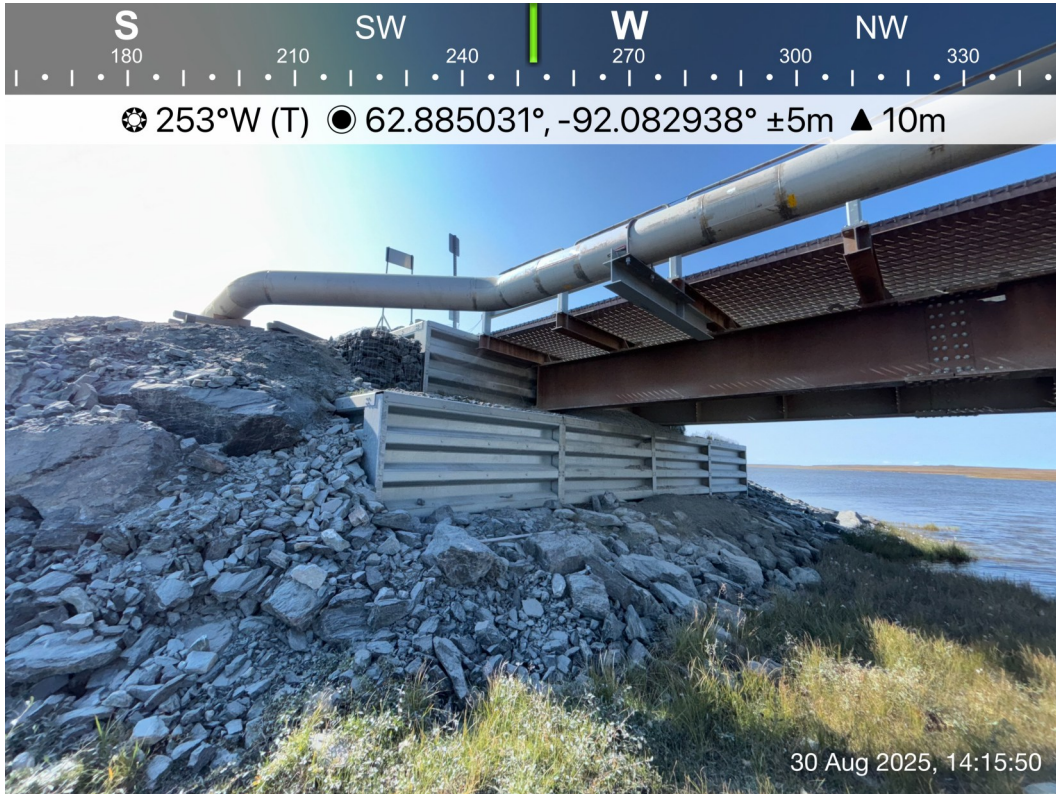
AWAR Road/ Culvert - Photo 33: M-5 Bridge KM 10.5: South abutment.
