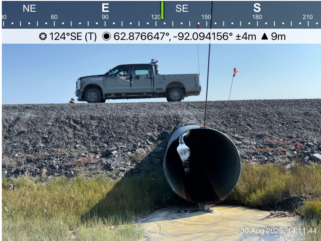
AWAR Road/ Culvert - Photo 31: Culvert KM 9.6: Outlet.
