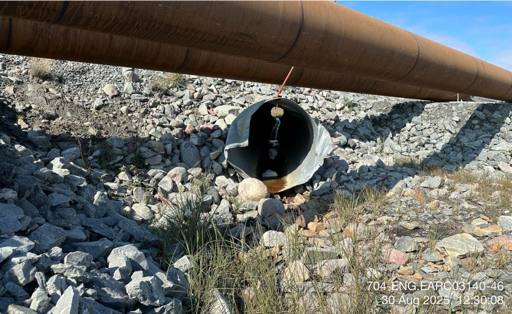
Itivia Bypass Road/ Culvert - Photo 40:
