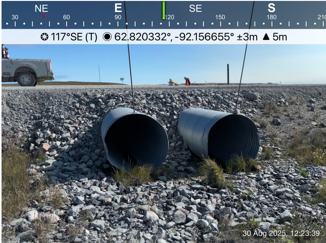
Itivia Bypass Road/ Culvert - Photo 35:
