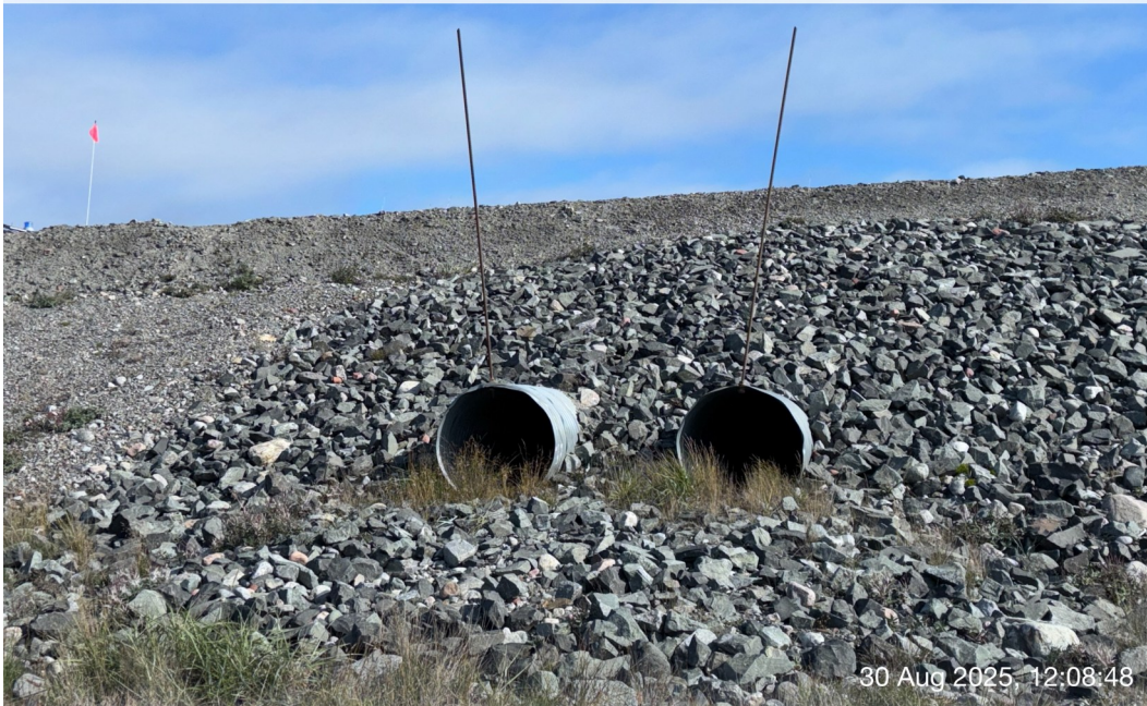
Itivia Bypass Road/ Culvert - Photo 26:
