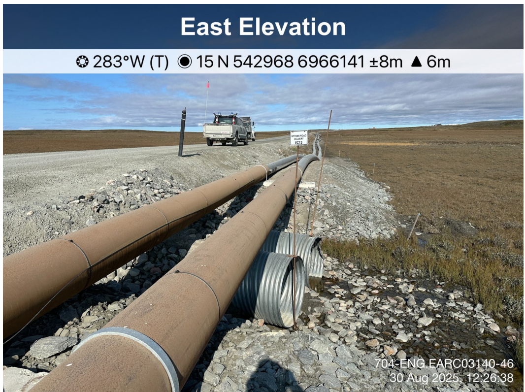
Itivia Bypass Road/ Culvert - Photo 36:
