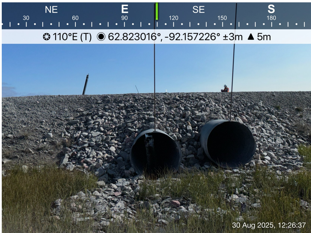
Itivia Bypass Road/ Culvert - Photo 38:
