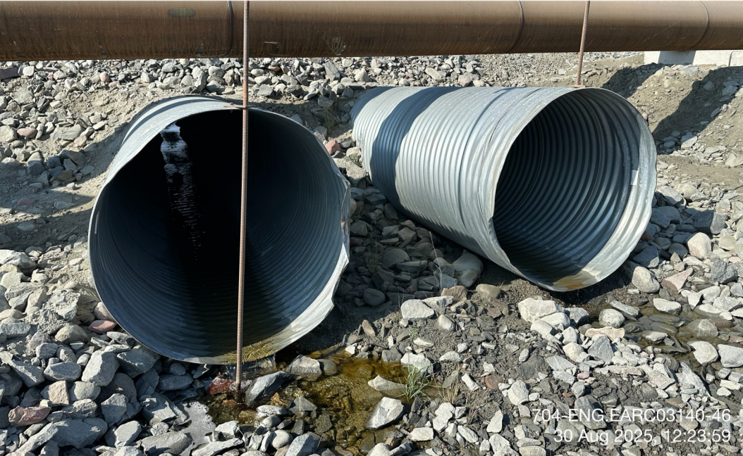
Itivia Bypass Road/ Culvert - Photo 34:
