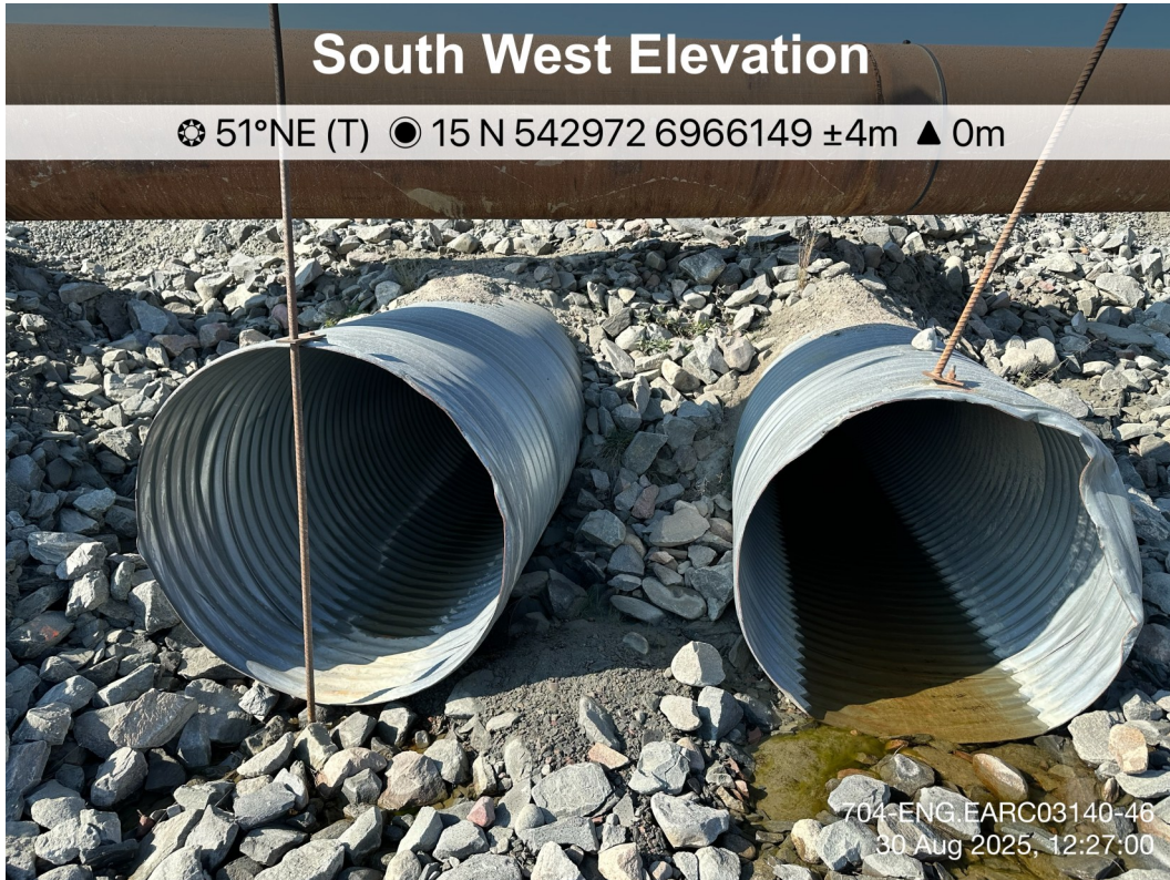
Itivia Bypass Road/ Culvert - Photo 37:
