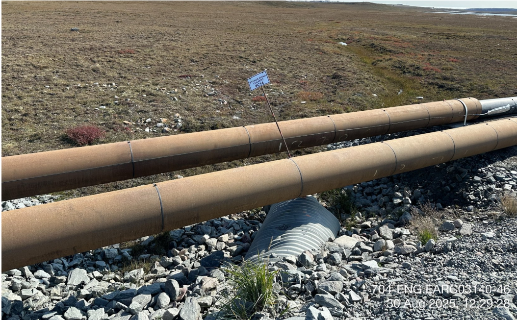
Itivia Bypass Road/ Culvert - Photo 39:
