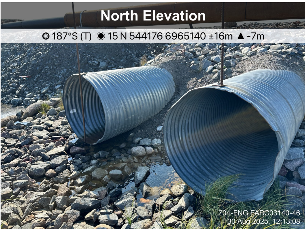
Itivia Bypass Road/ Culvert - Photo 28:
