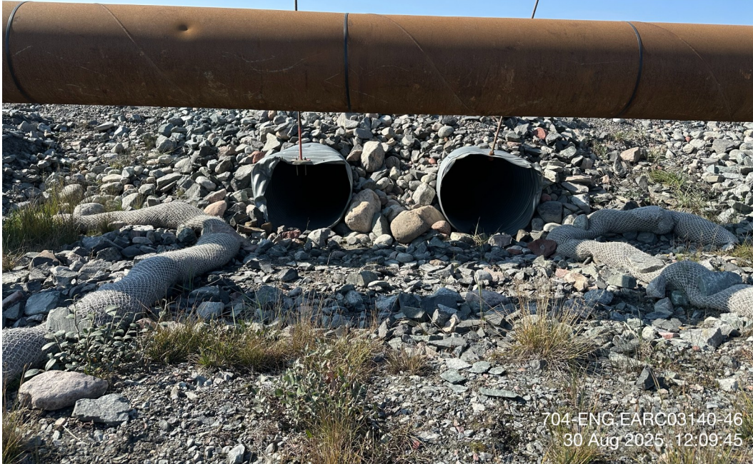
Itivia Bypass Road/ Culvert - Photo 25:
