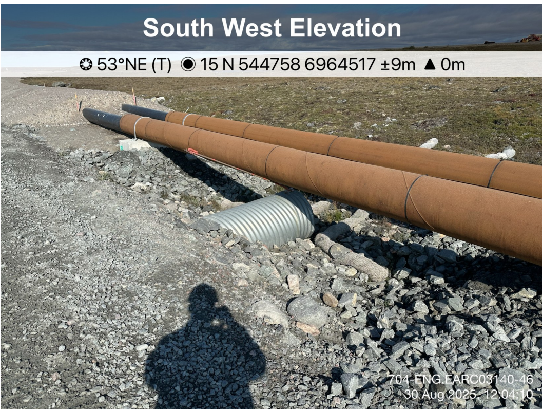
Itivia Bypass Road/ Culvert - Photo 18:
