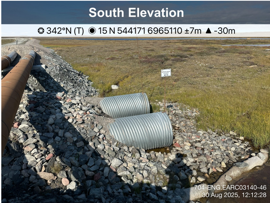
Itivia Bypass Road/ Culvert - Photo 27:
