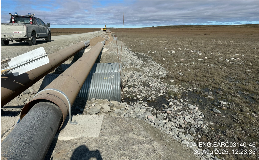
Itivia Bypass Road/ Culvert - Photo 33:
