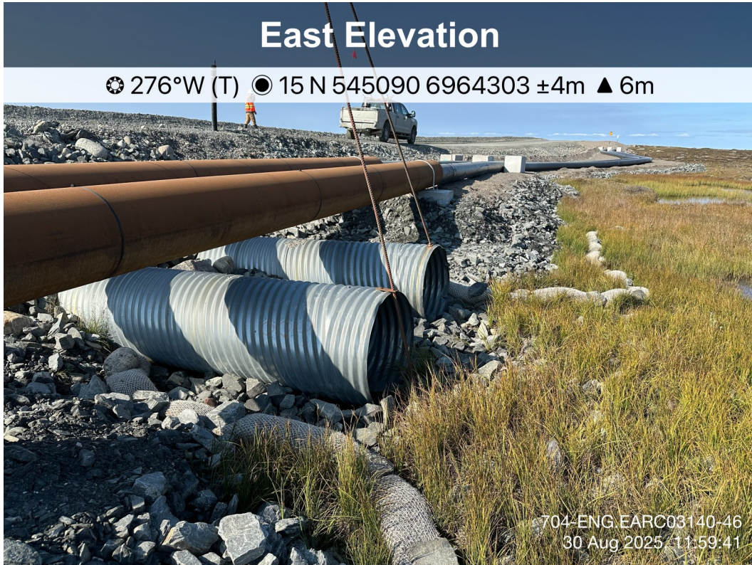
Itivia Bypass Road/ Culvert - Photo 13:
