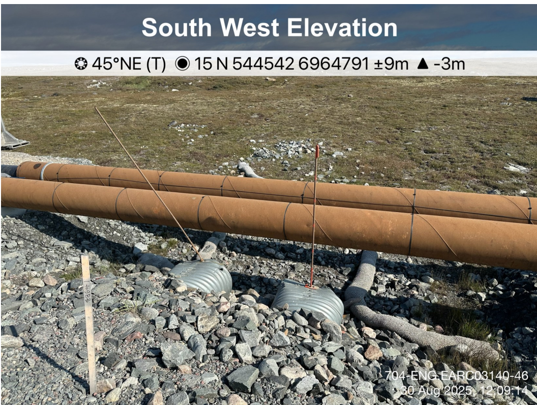
Itivia Bypass Road/ Culvert - Photo 24:
