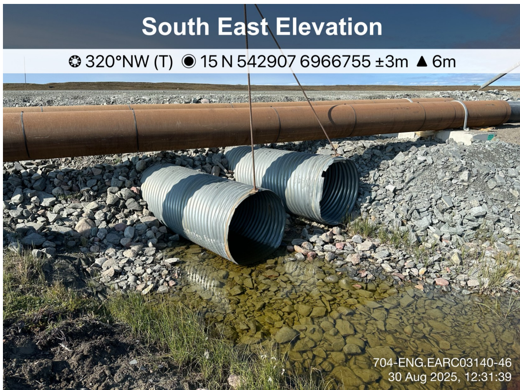
Itivia Bypass Road/ Culvert - Photo 42:
