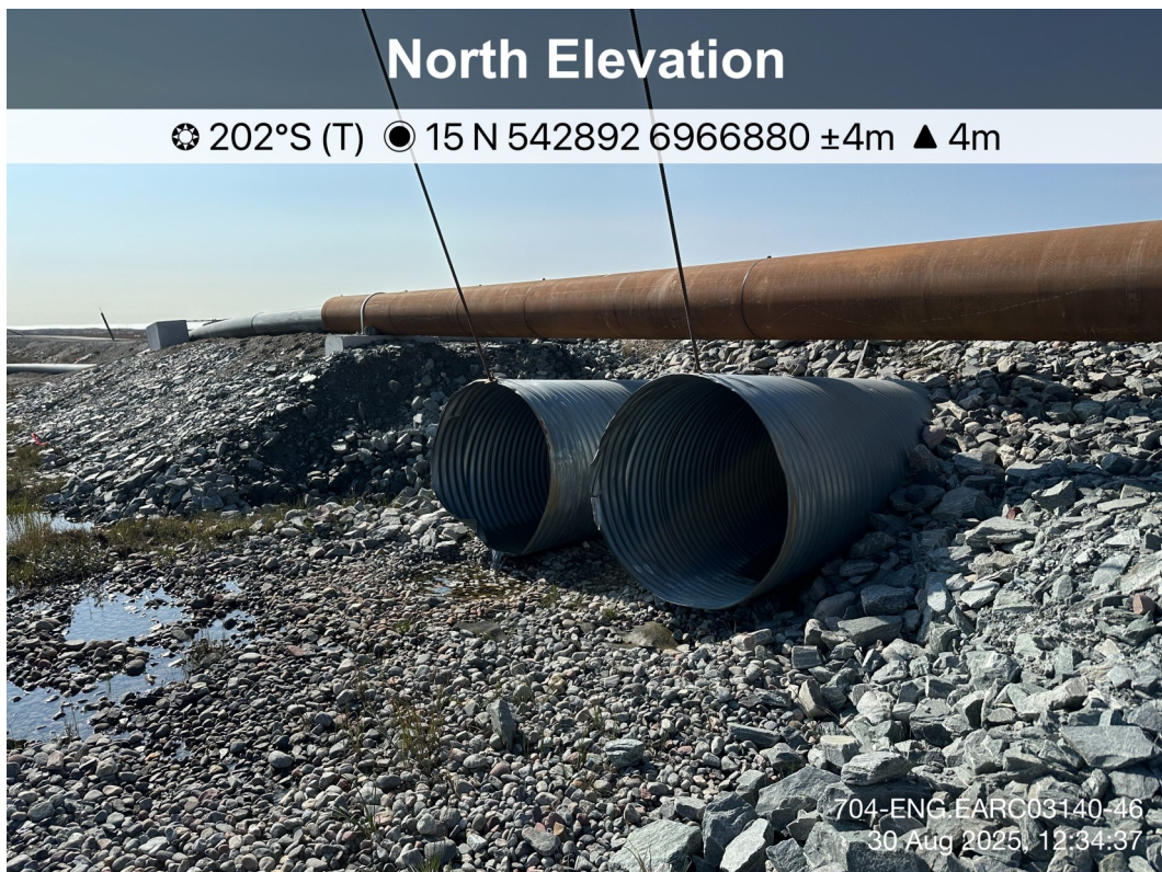
Itivia Bypass Road/ Culvert - Photo 44:
