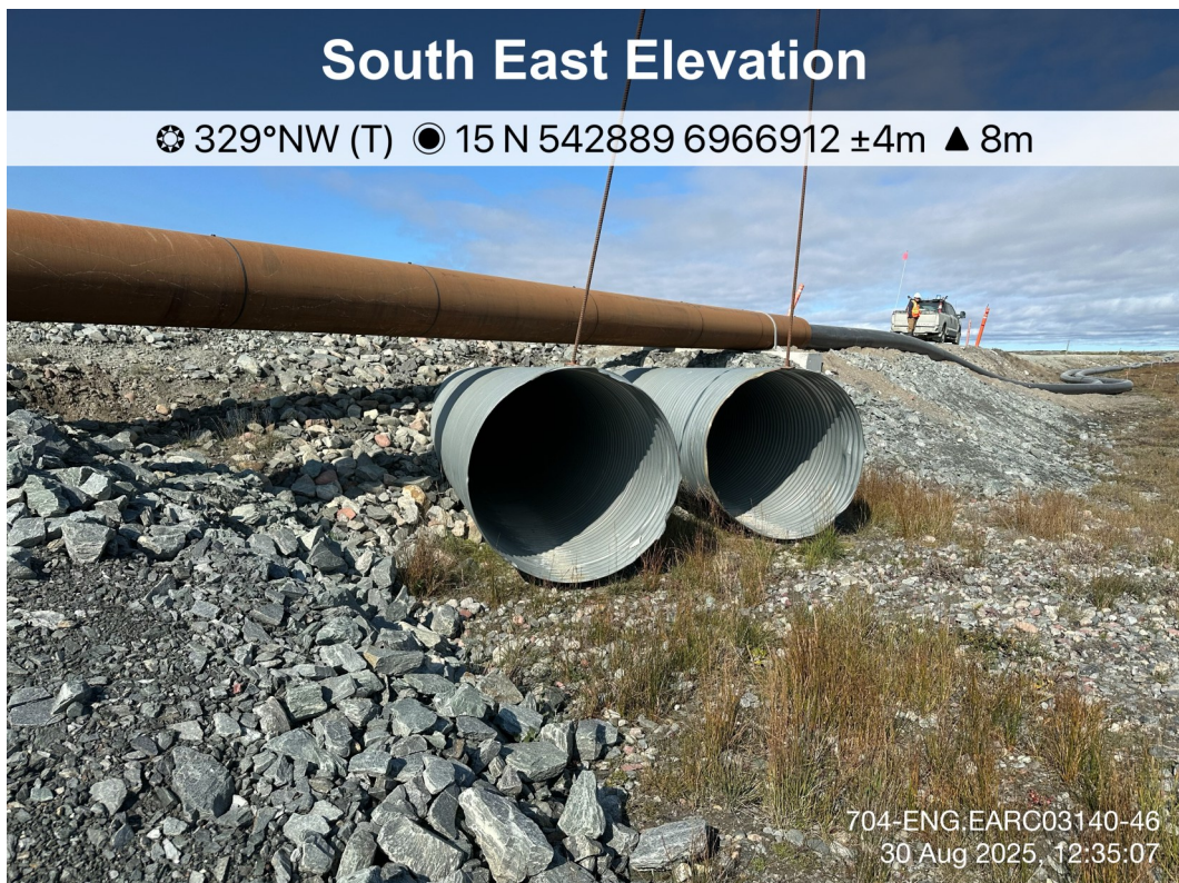
Itivia Bypass Road/ Culvert - Photo 46:
