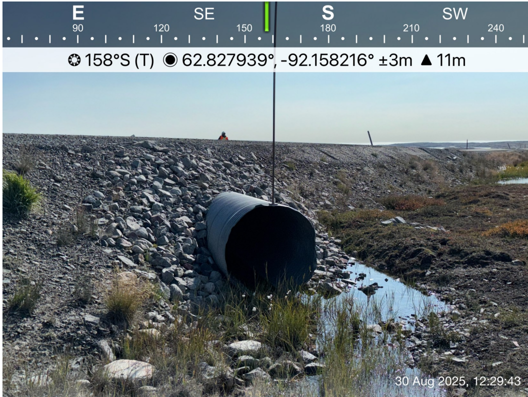
Itivia Bypass Road/ Culvert - Photo 41:
