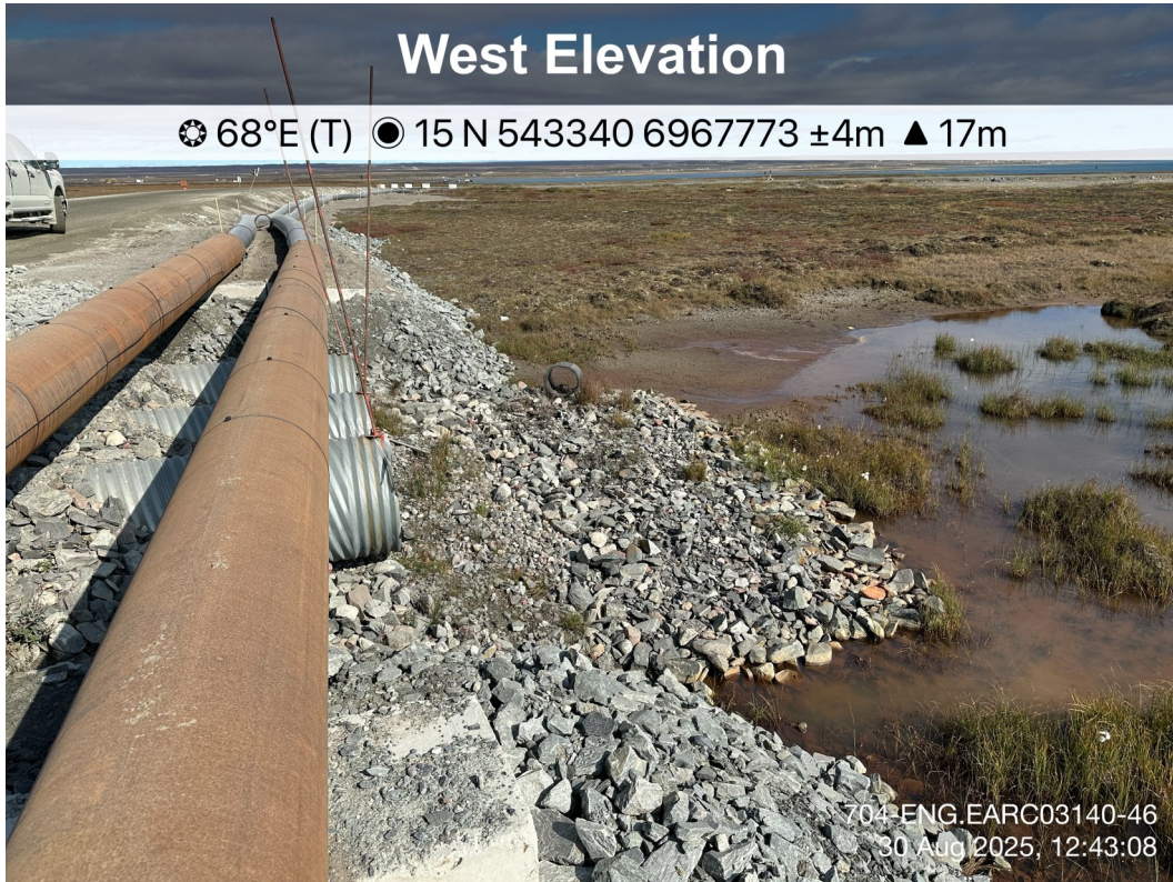
Itivia Bypass Road/ Culvert - Photo 51:
