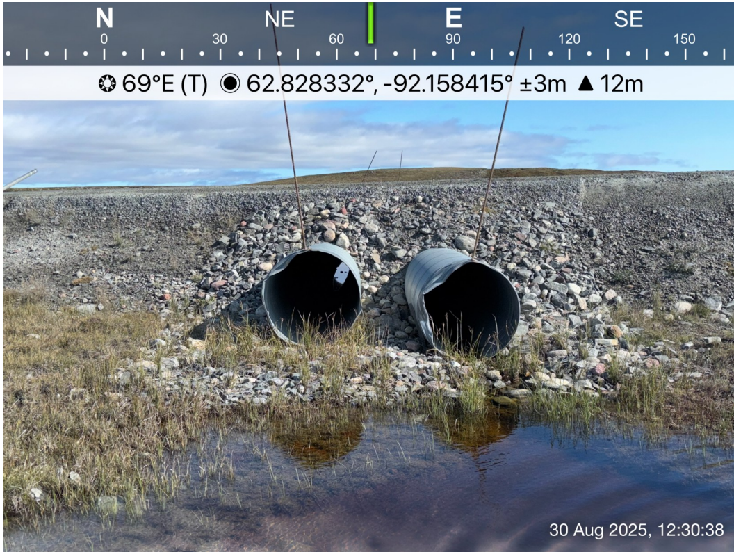
Itivia Bypass Road/ Culvert - Photo 43:
