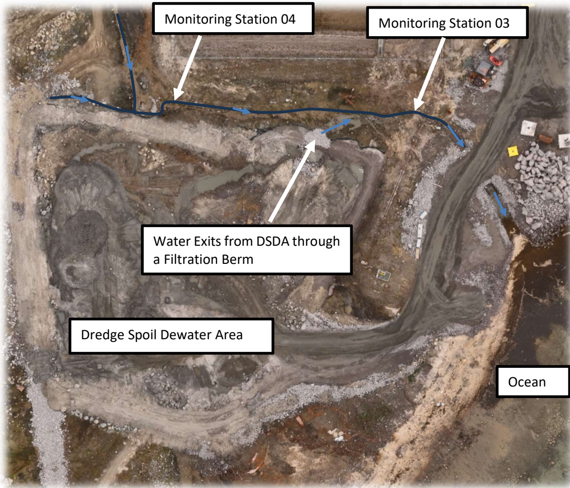
Location of Monitoring stations 03 and 04, Dredge Spoil Dewatering Area
