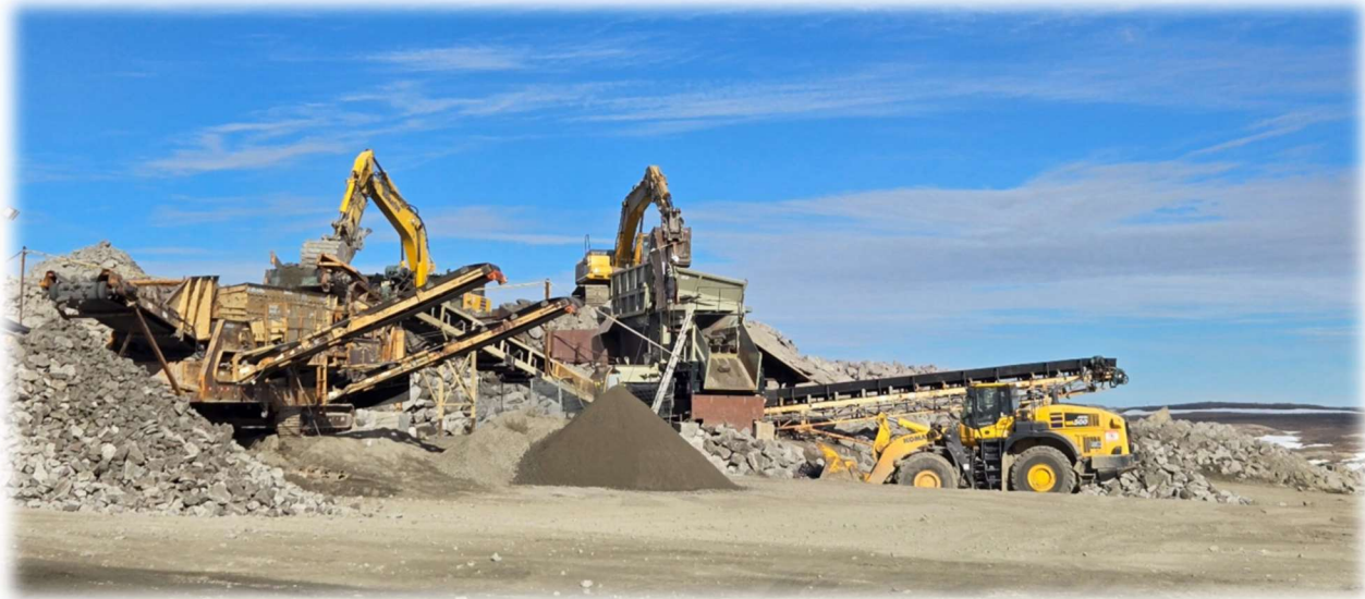
Quarry and Material Processing Area
