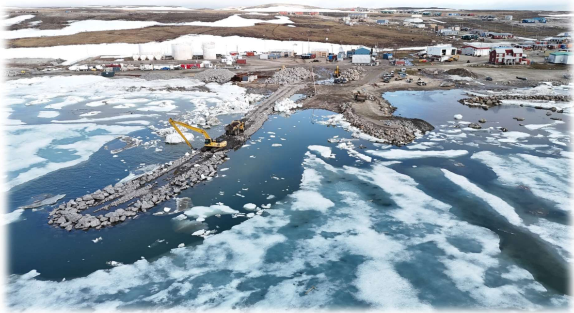
Northeast Breakwater Construction
