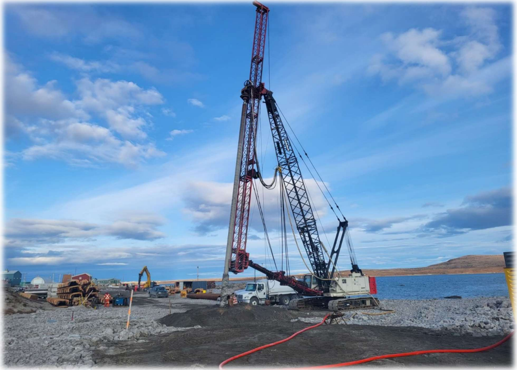
New Mooring Bollard Installation
