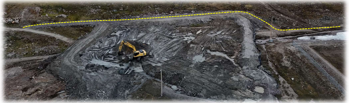
ATV access road built for ATV
