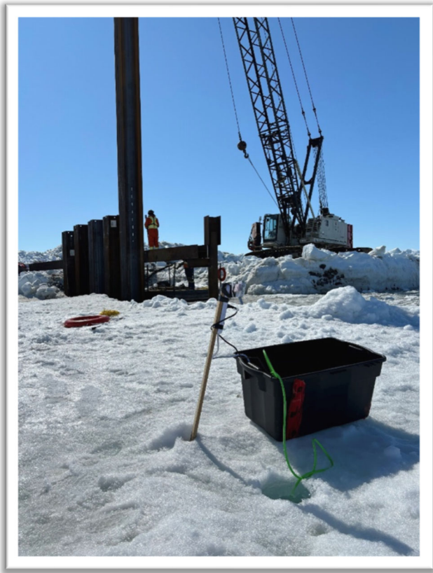
Monitoring Station 01 Located at 10 m from the Piling Site
