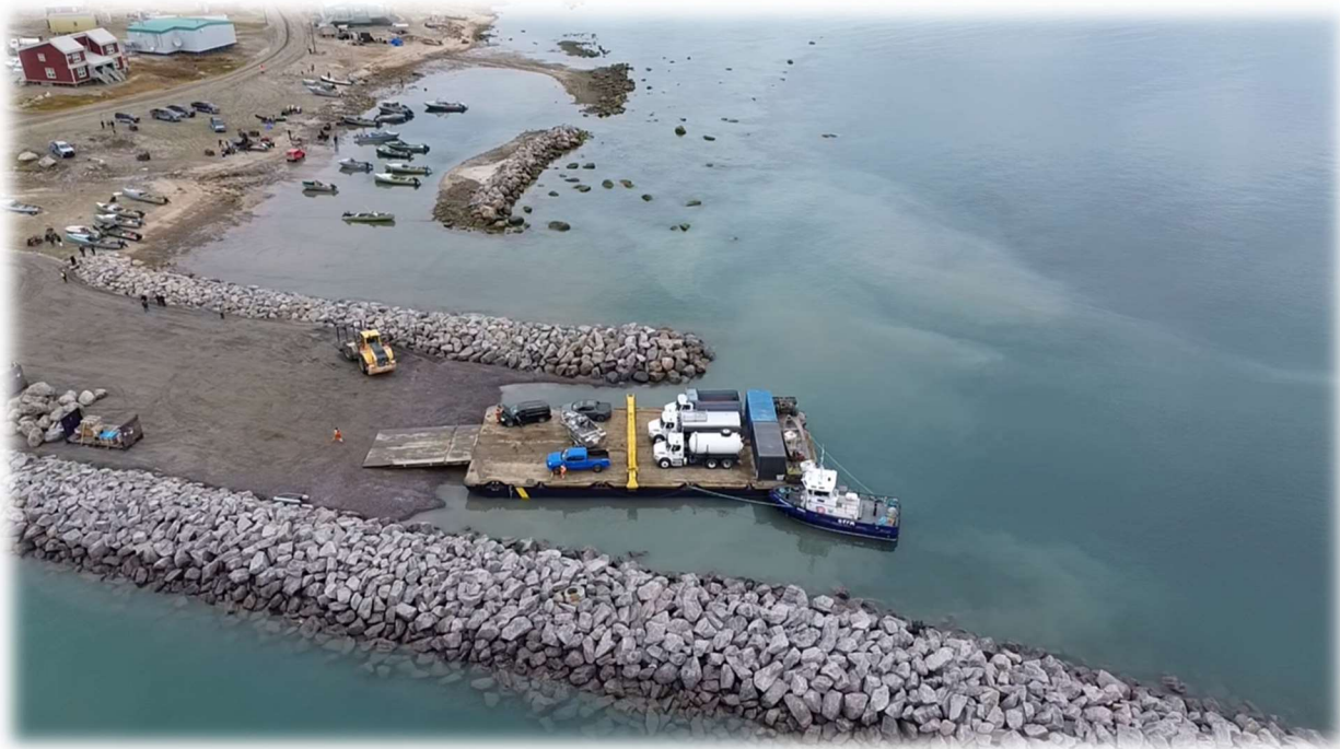
Northeast Breakwater & Sealift Breakwater Construction Completed
