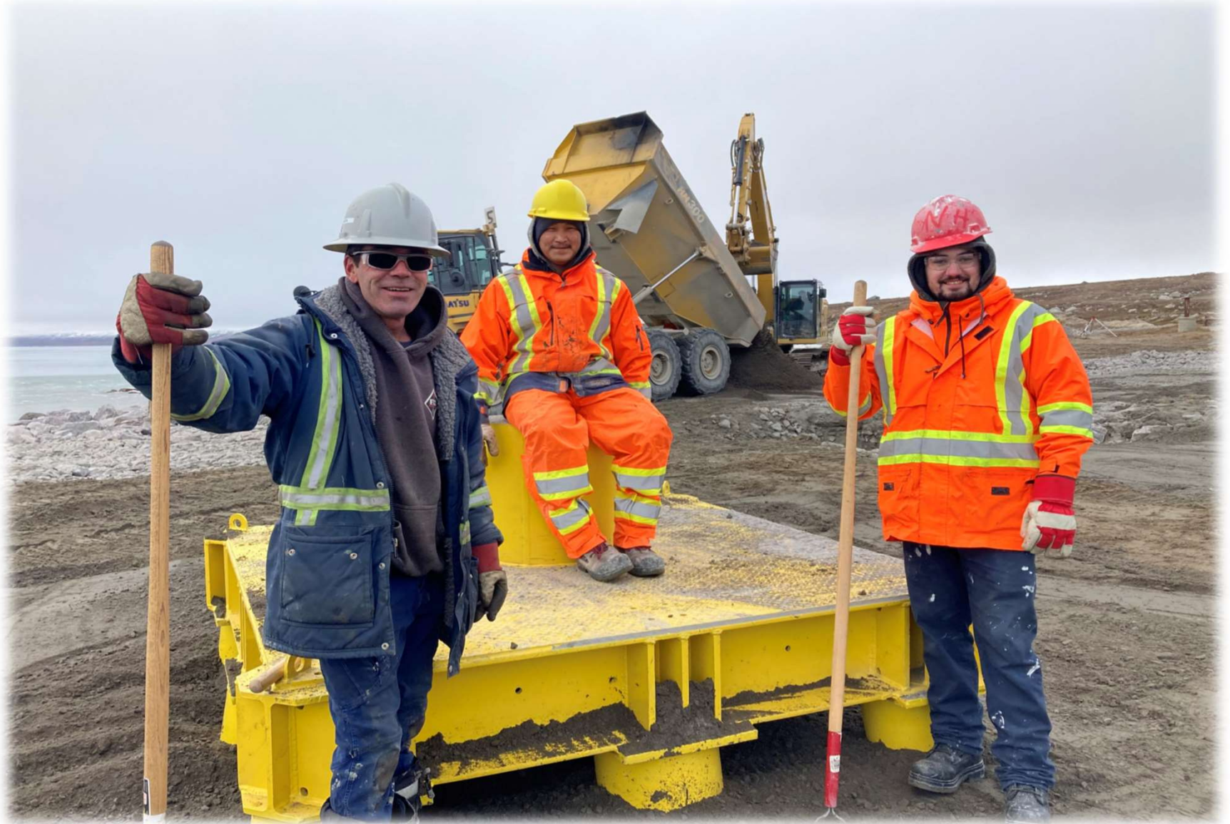
New Mooring Bollard
