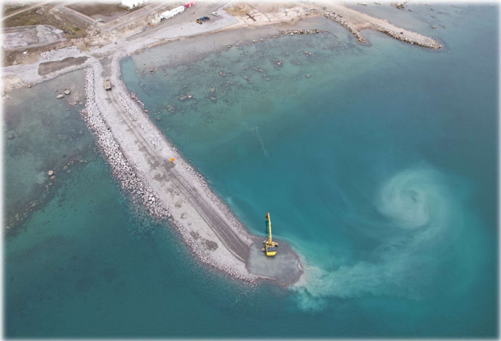
Southwest Breakwater Construction August 12, 2023
