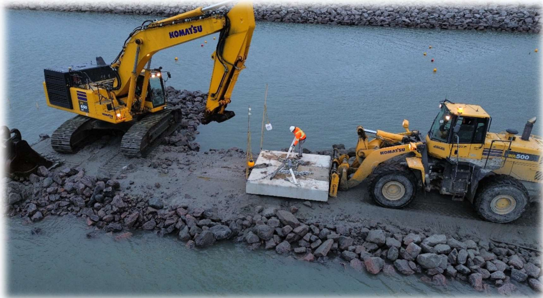
Installation of the Concrete Anchor Blocks for the Floating Wharf
