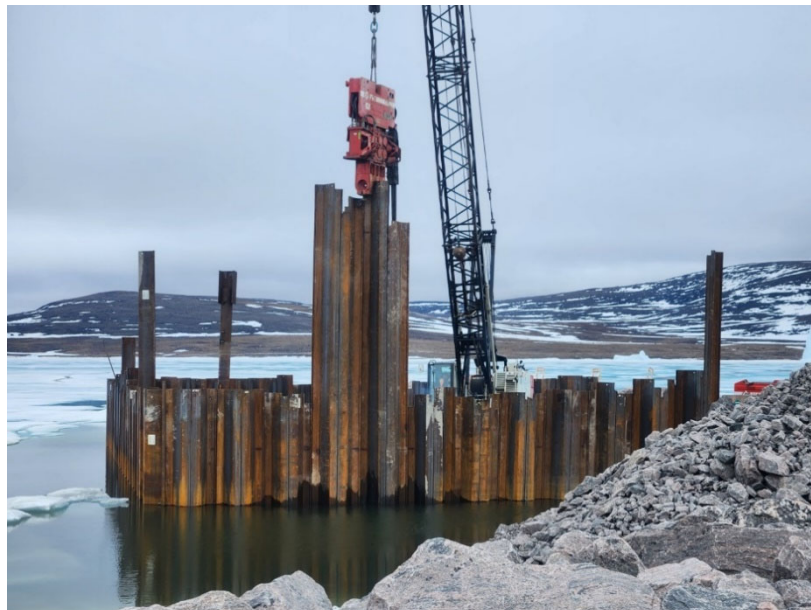
Steel sheet pile installation with the vibrodriver on the west wall
