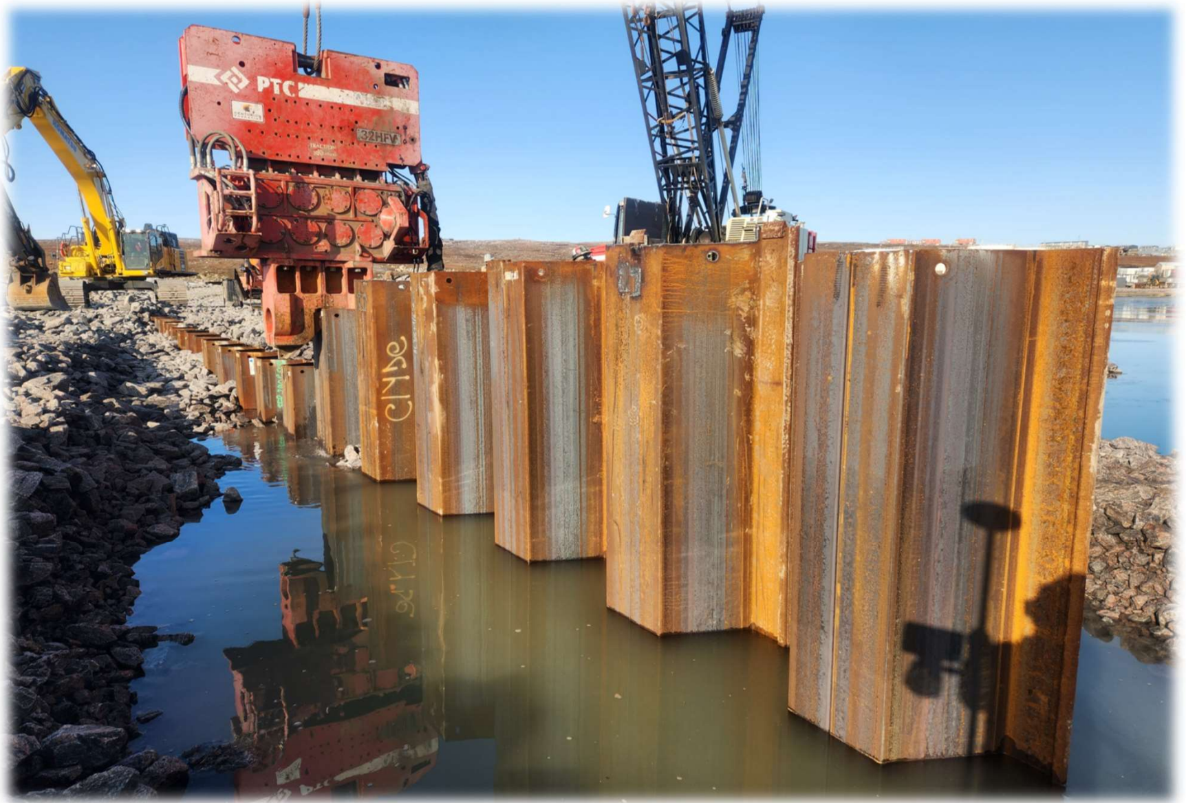
Sheet Pile Installation
