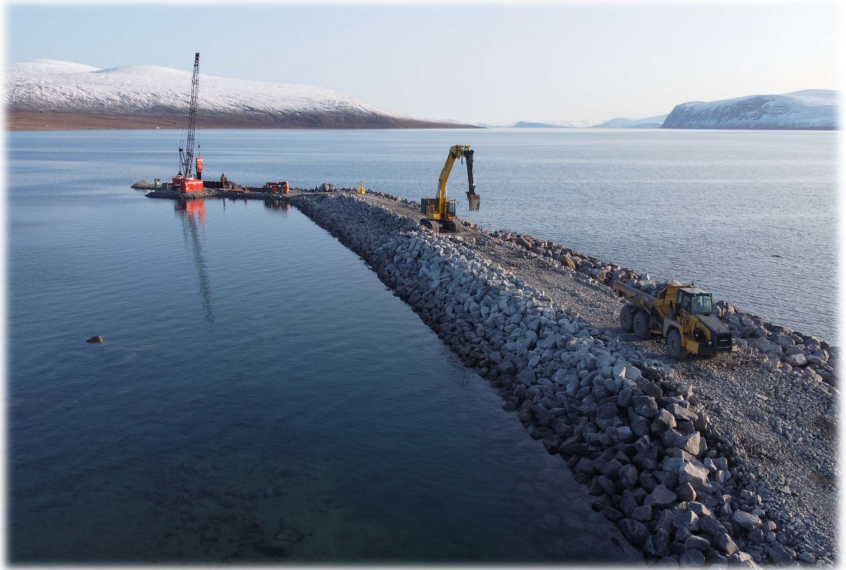
Southwest Breakwater Construction September 25, 2023
