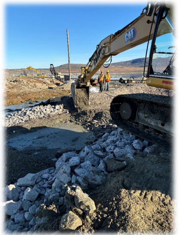
Improvement of the Decantation Basin at the DSDA
