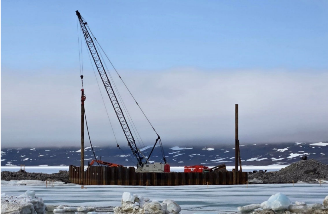
Toe pin installation on the north wall
