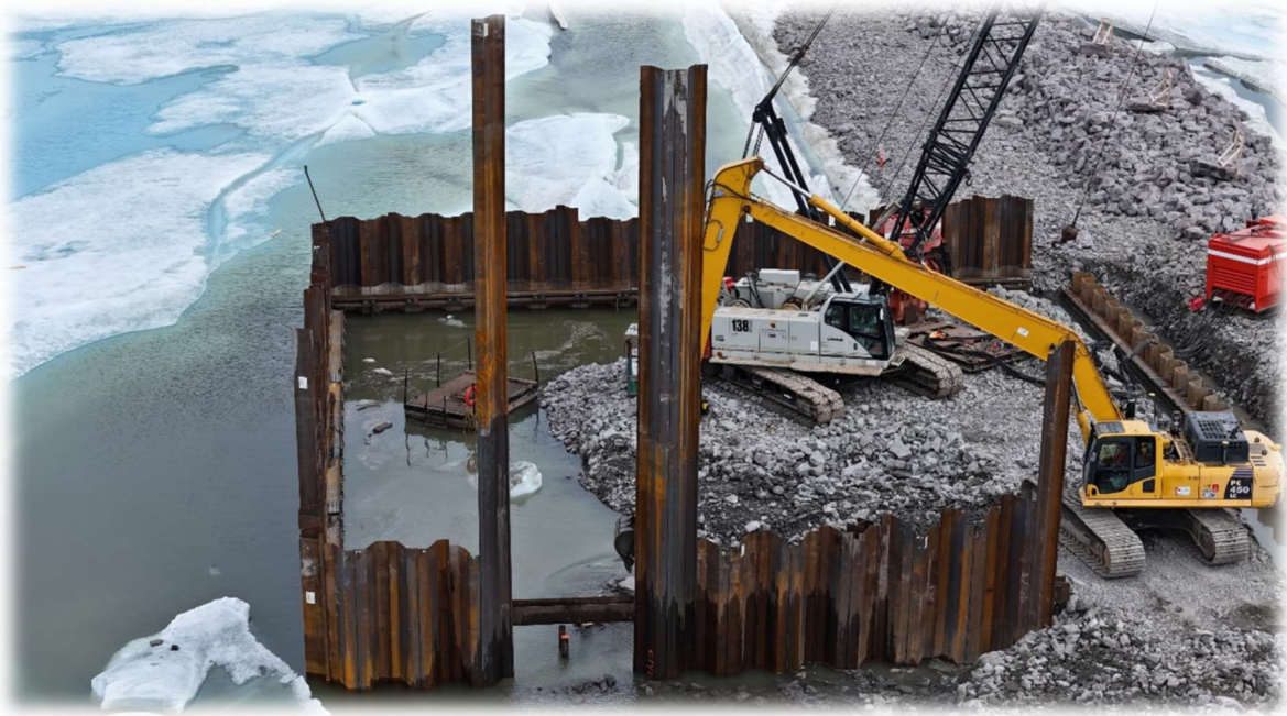
Steel Sheet Pile Installation at the Fixed Wharf
