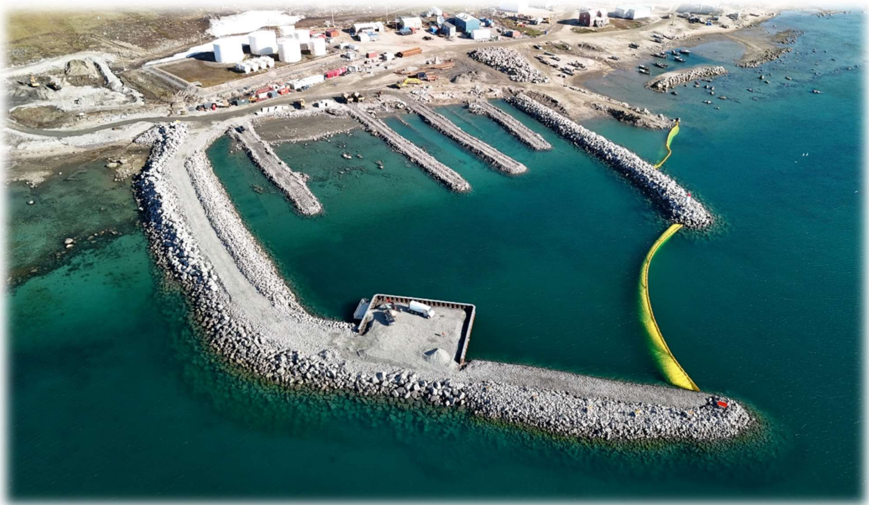
Northeast Breakwater Construction Completed
