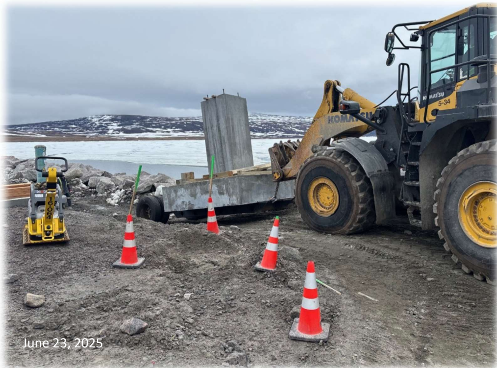
Navigation light foundation installation at the end of the southwest breakwater
