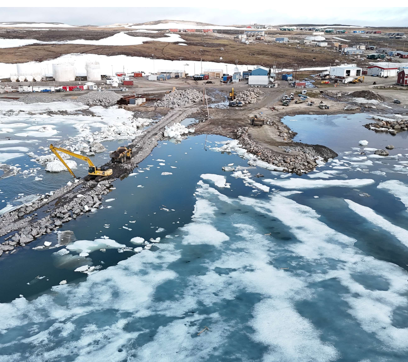
Northeast Breakwater Construction July 5, 2024
