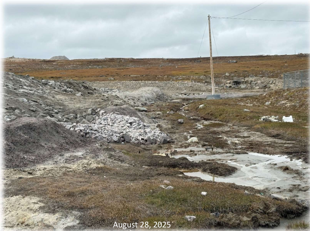
Silt fences removed at the Dredge Spoil Dewatering Area
