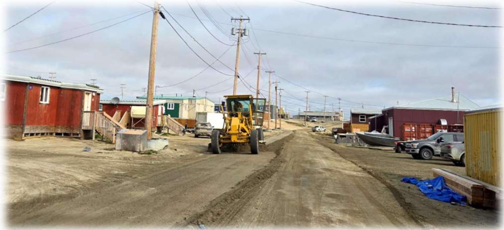
Road Maintenance, Hamlet Road
