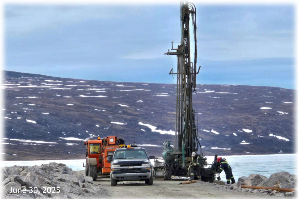
Drilling piles for the power pole installation
