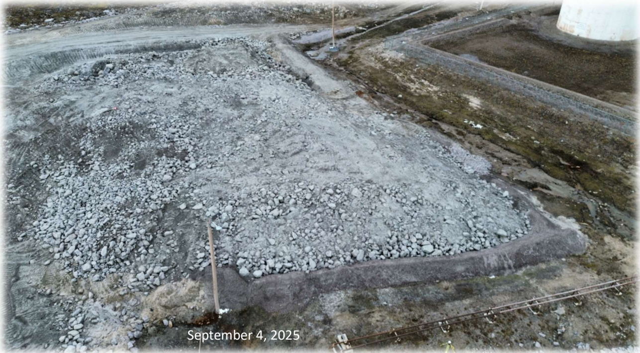
Sediment decantation pond removed
