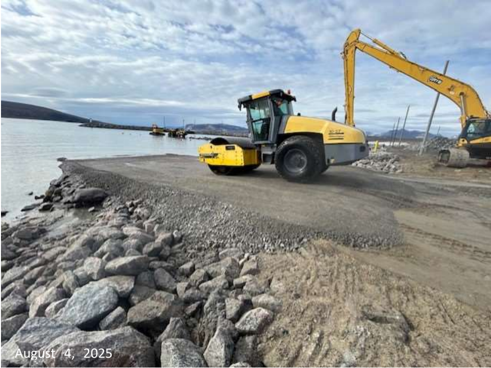
Boat ramp construction
