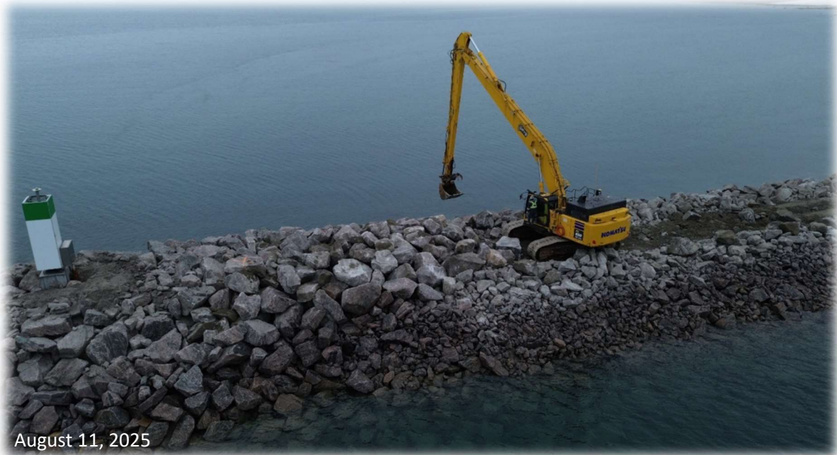
Finalizing the construction of the southwest breakwater
