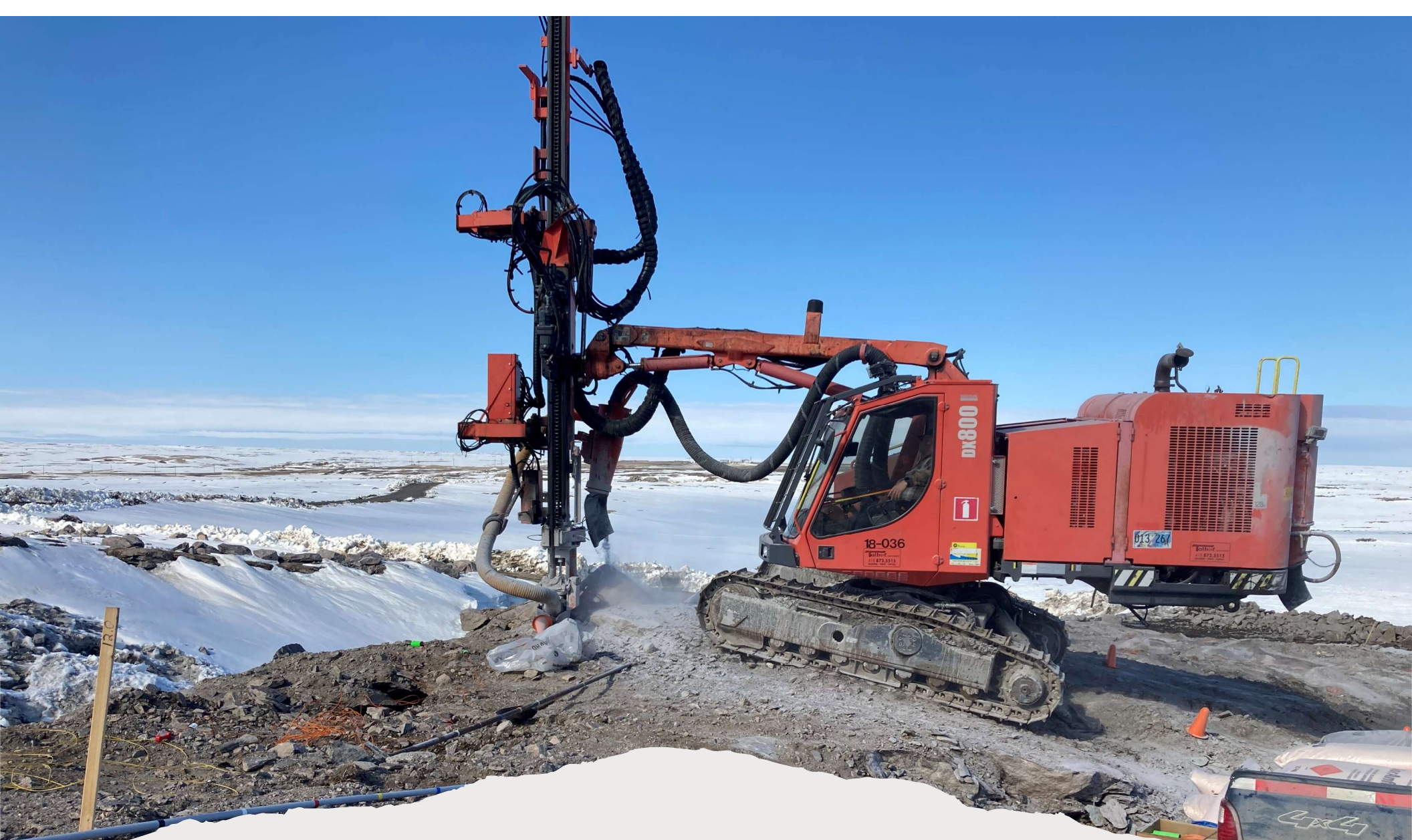
Drilling and blasting at the quarry
