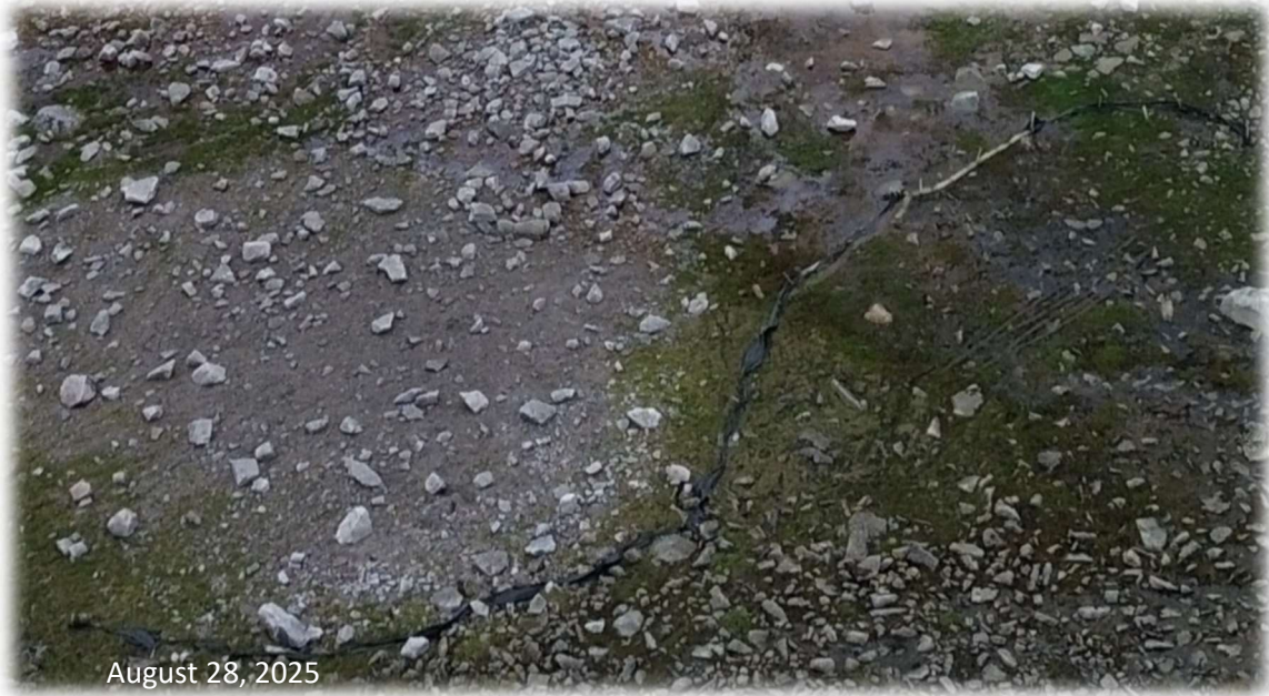
Silt Fences Installed Between the Wetland and the Quarry North End
