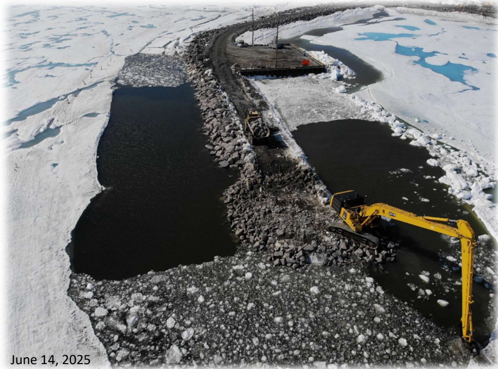
Nose construction of the southwest breakwater
