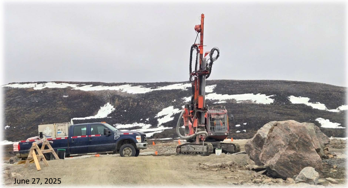
Drilling at the quarry for the last blast
