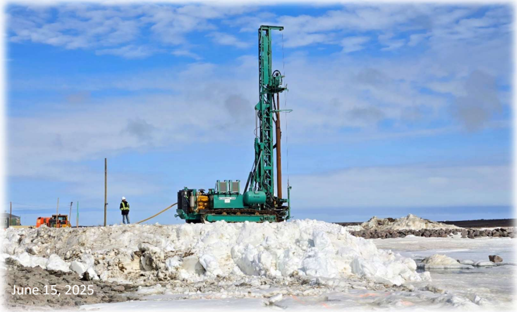
Floating wharf guide pile installation
