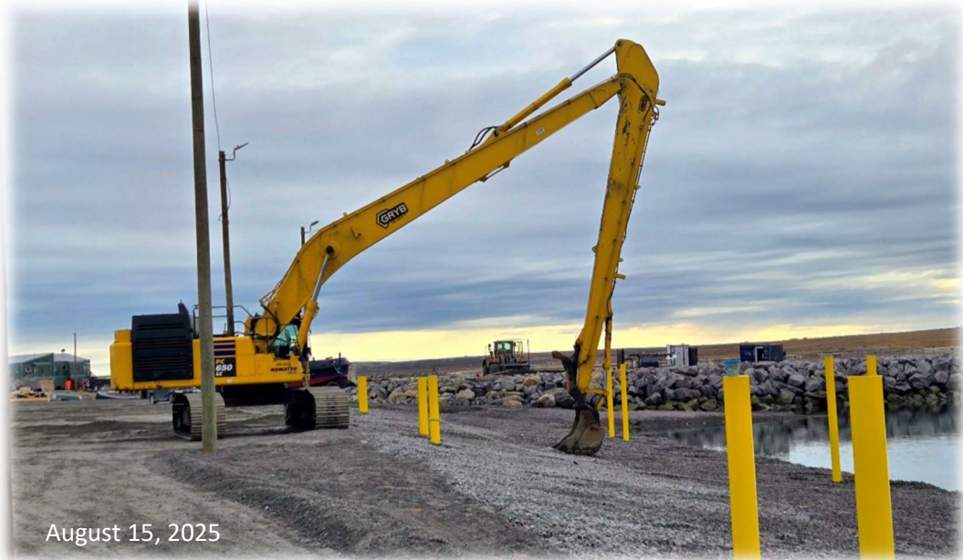
Floating wharf guide piles installed
