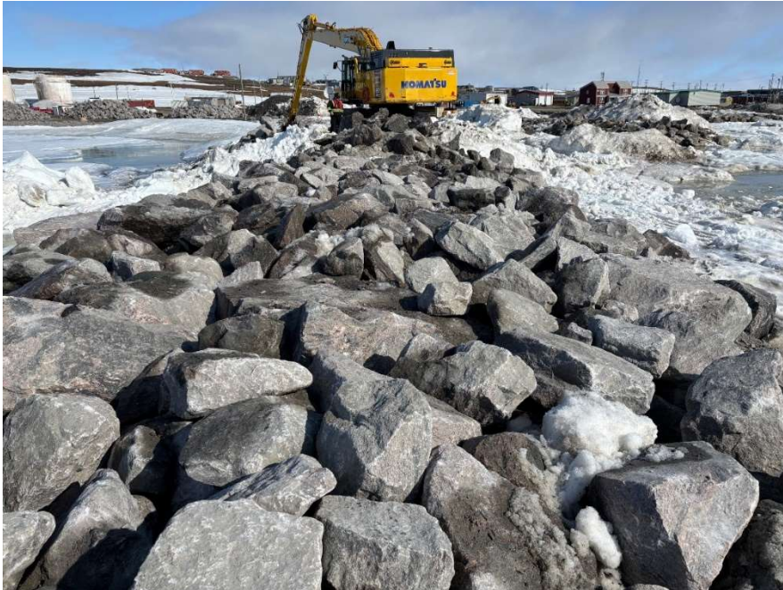
Excavator placing smaller rocks on the northeast breakwater
