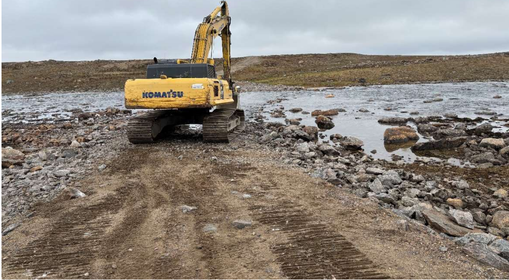
Figure 4: Removal of the North side
