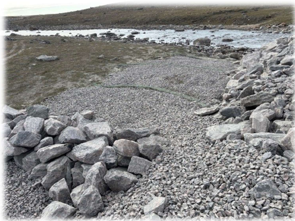
Permanent erosion protection measures on each side of the bridge approaches
