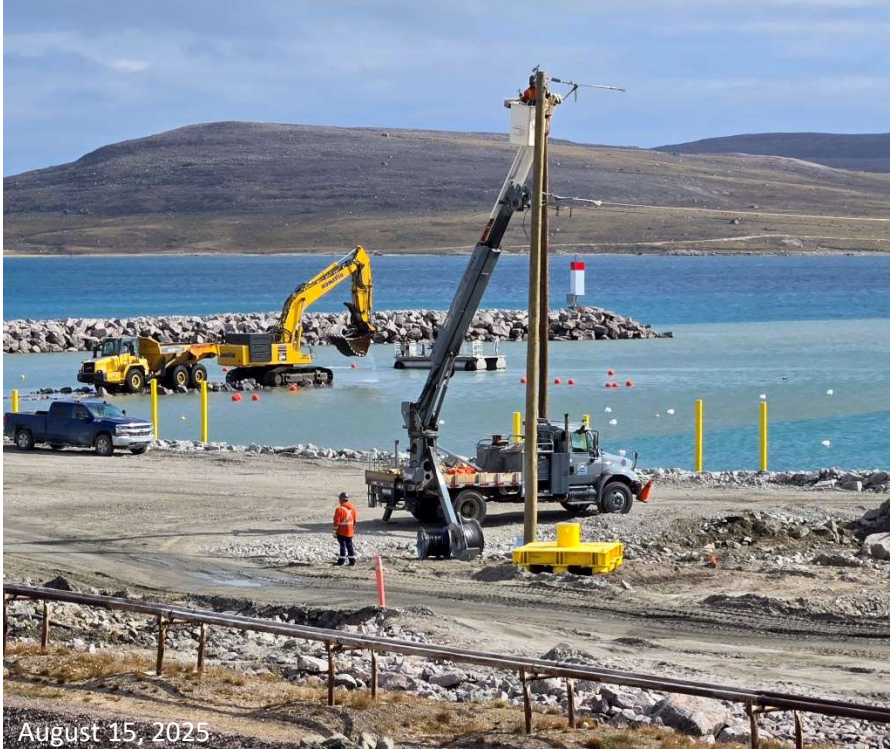
Overhead lines and flood lights installation
