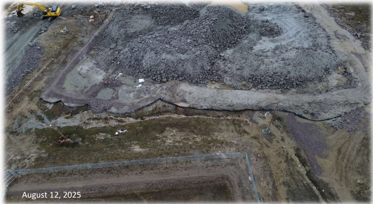
Silt fences installed at the Dredge Spoil Dewatering Area
