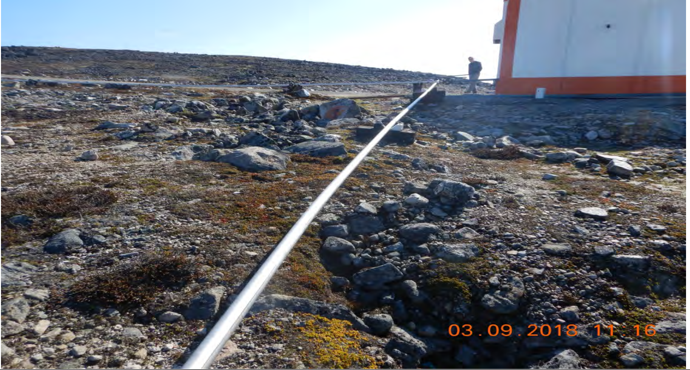
Description: intake pipe to pump house.
