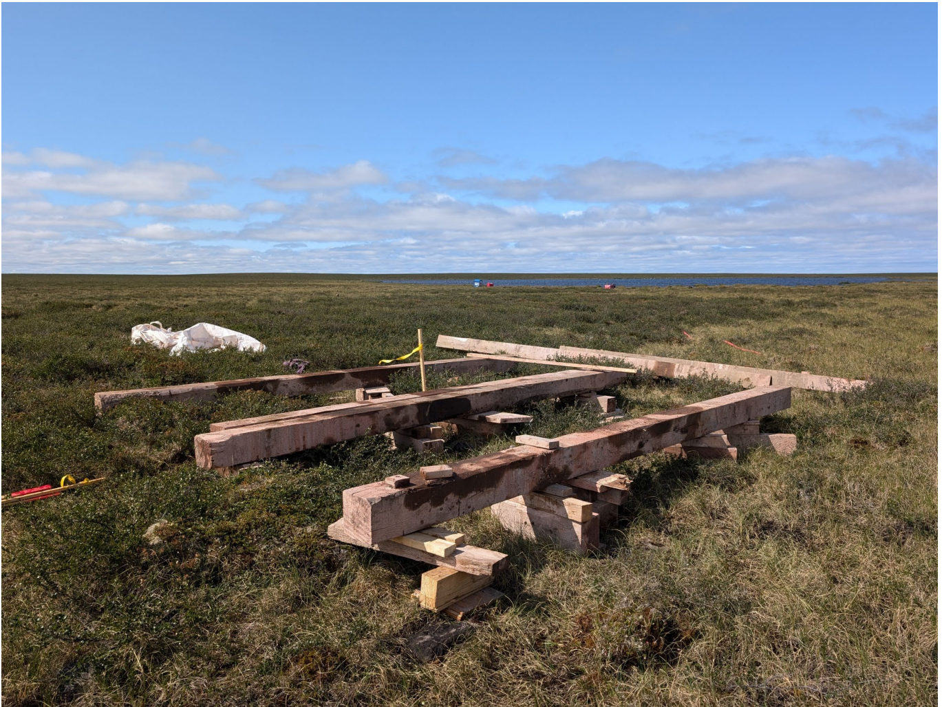
Figure 10-12 Constructing a drill pad at the Tatiggaq target area.
