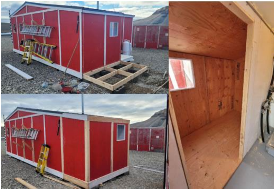
Photo 5 – Water utility room expansion.
